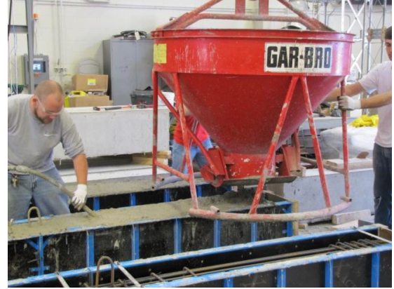
(b) Concrete placement
