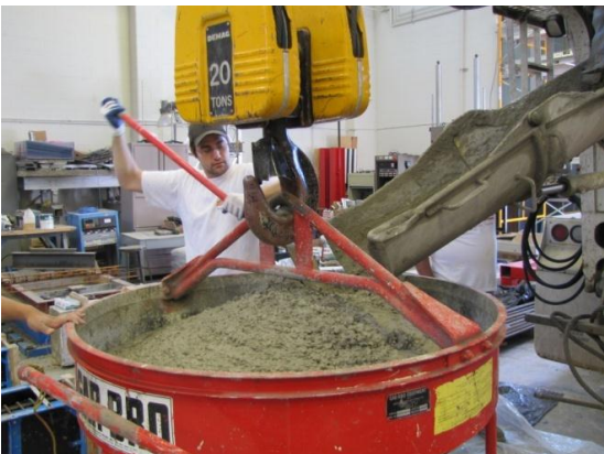
(c) Concrete placement
