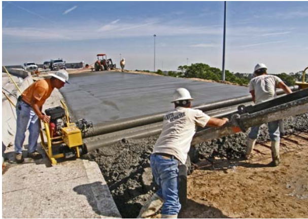
a) Roadway Placement (Roadway Access Ramps, 2012)
