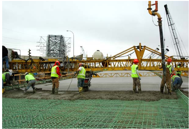
b) Bridge Deck Placement (Memorial Bridge)
