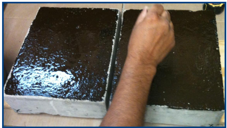
Application of EBL Tack Coat before Placing an HMA Overlay
