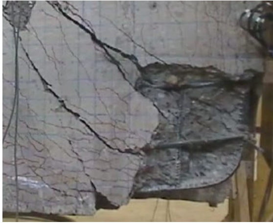
(a) Failure at the exterior corner
