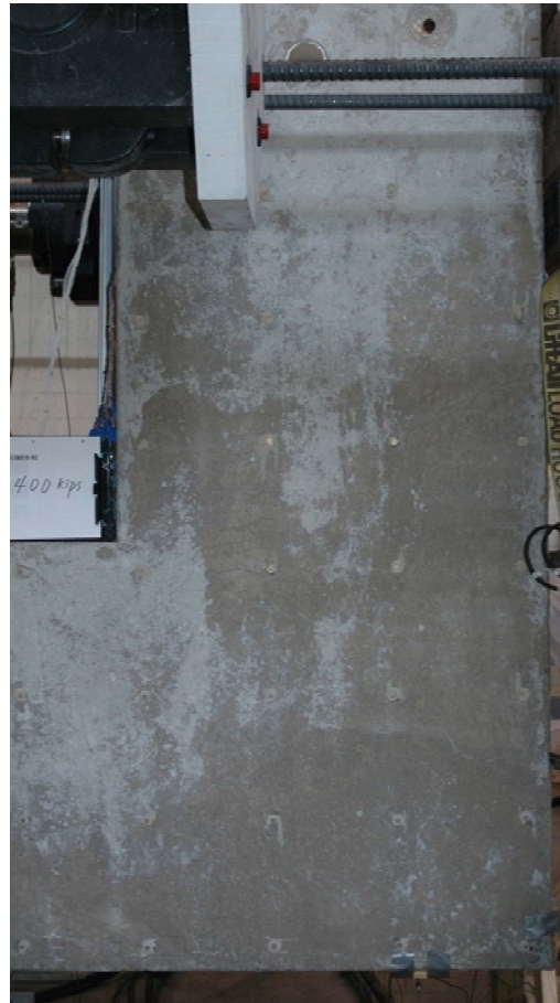
(b) Singly reinforced beam
