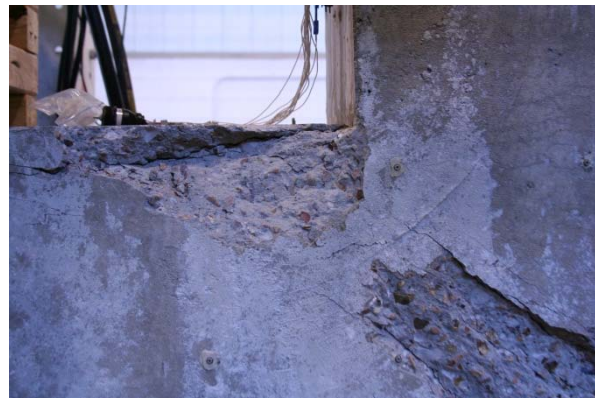
(d) After removal of the spalled concrete
