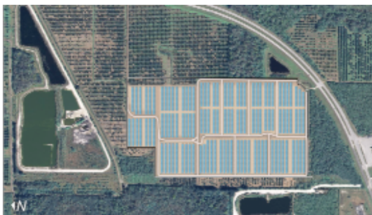
The center of this graphic shows an artist's rendering of the FPL Space Coast solar facility, to be built on KSC land.
