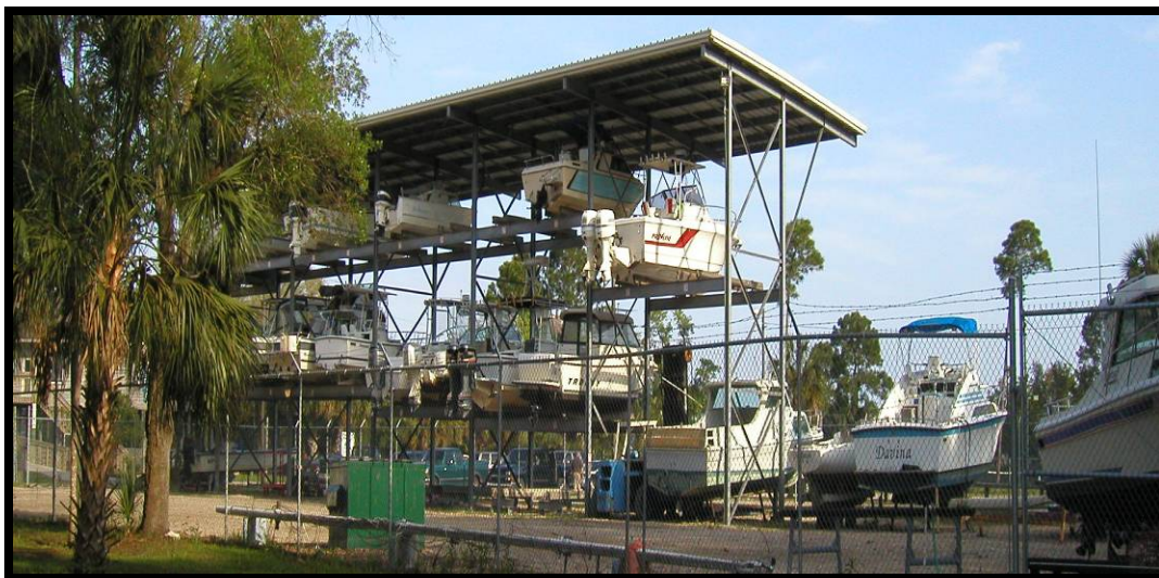
Panacea Dry Dock Storage Facility
