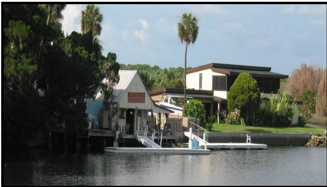
Former fish house in Aripeka
