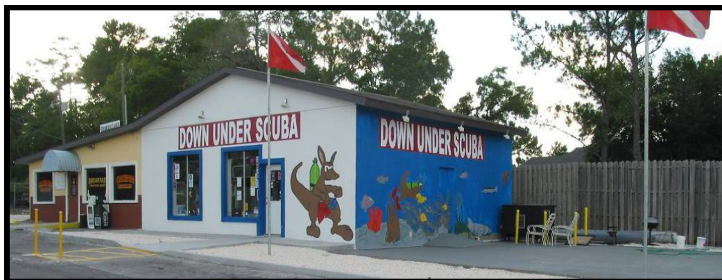
Dive Shop along Highway 19 in Spring Hill
