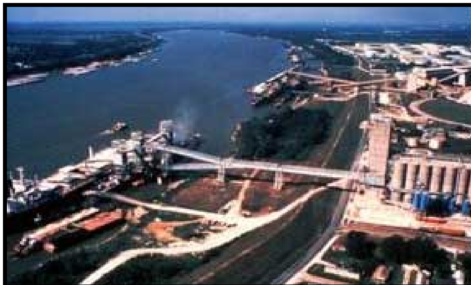
Industrial Area in St. Charles Parish (courtesy of stcharlesgov.net)
