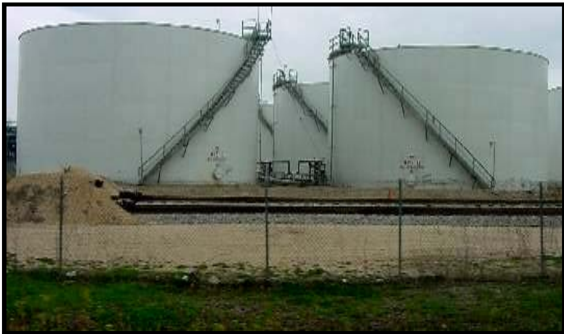
Petroleum Storage Facility at Braithwaite
