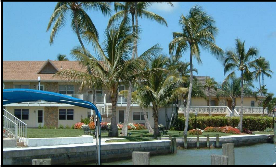
Condominiums on Marco Island
