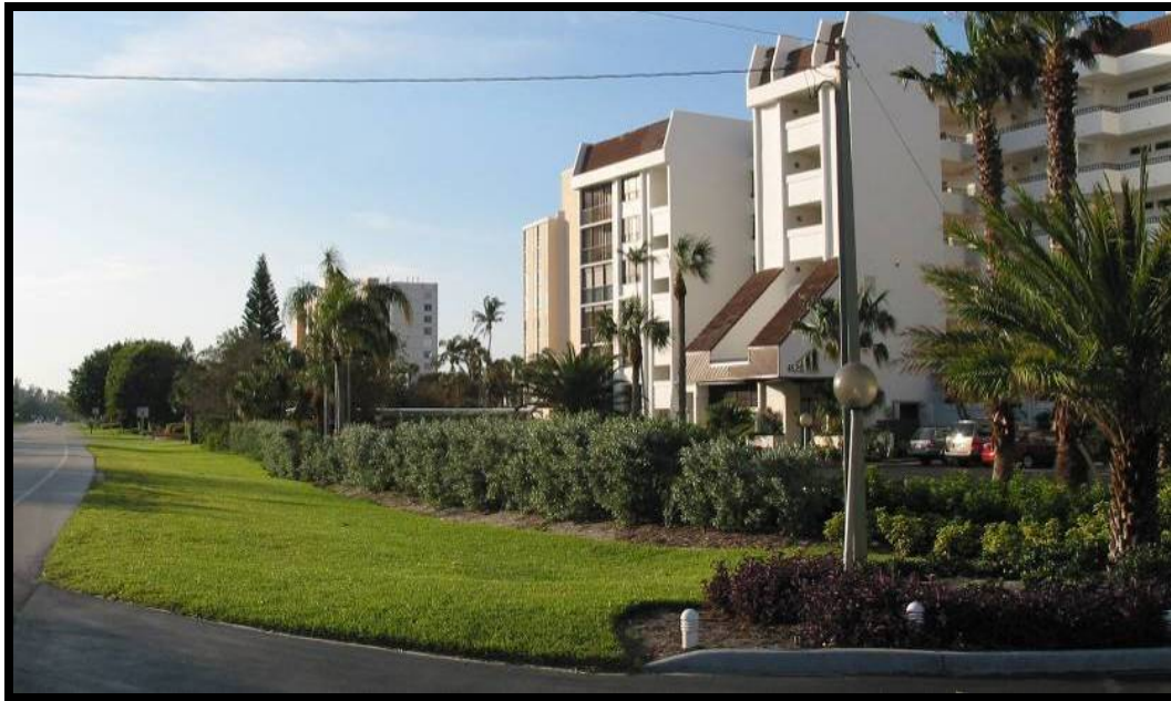
Condominium Development in Longboat Key
