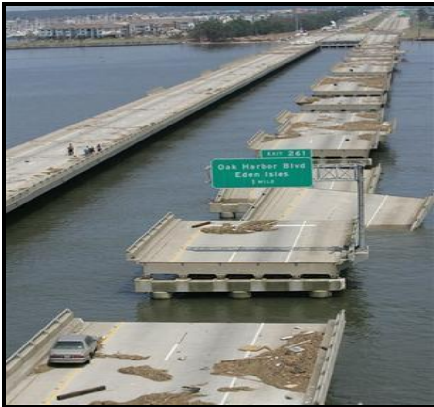
Immense Infrastructure Damage after Hurricane Katrina: Slidell (Online source: Brandon Baker)
