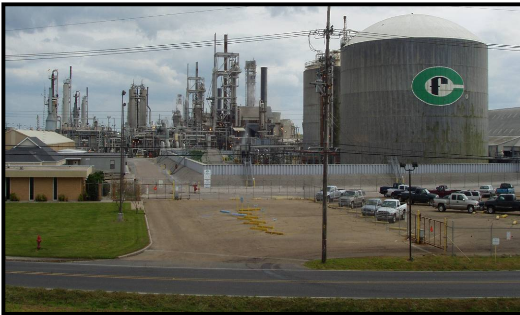
Petrochemical Plant in Donaldsonville Area
