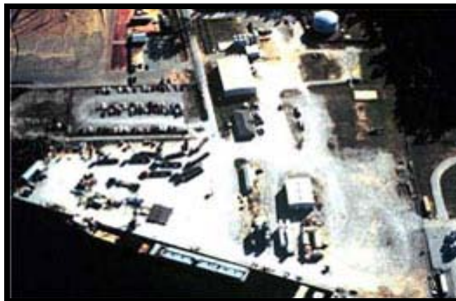
Aerial Image of Industrial Area in Theodore (Courtesy of midstreamfuel.com)
