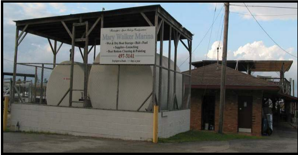
Fuel Tanks at Marina in Gautier
