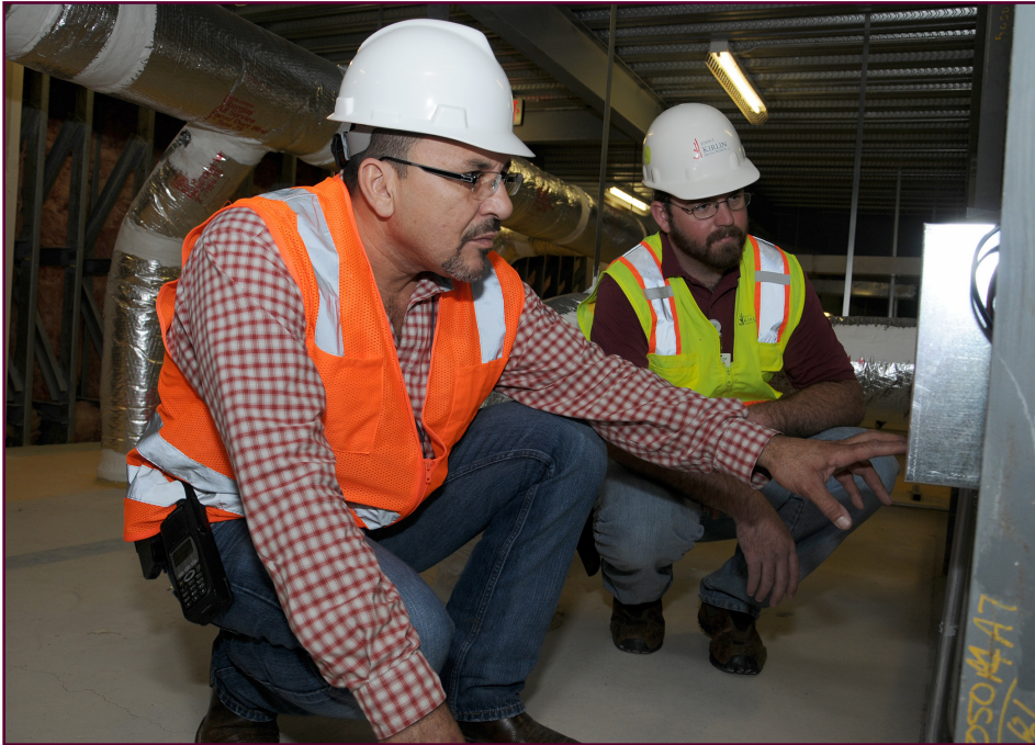
ISR Civilian of the Year, Narciso "Chicho" Salinas Jr., inspects completed duct work while Robert Payne, project manager looks on.
