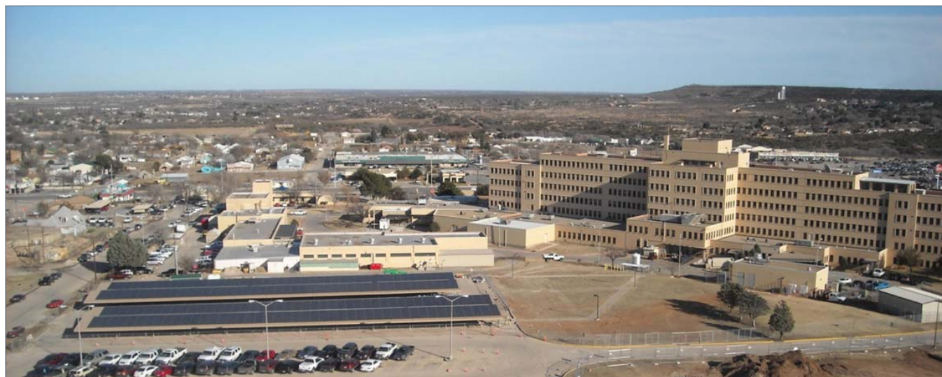
Carport-mounted photovoltaic system at the West Texas VA Medical Center.
