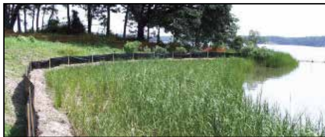
Newly planted marsh with fiber logs allowing plants to establish root system and stabilize shoreline. Source: VIMS.
