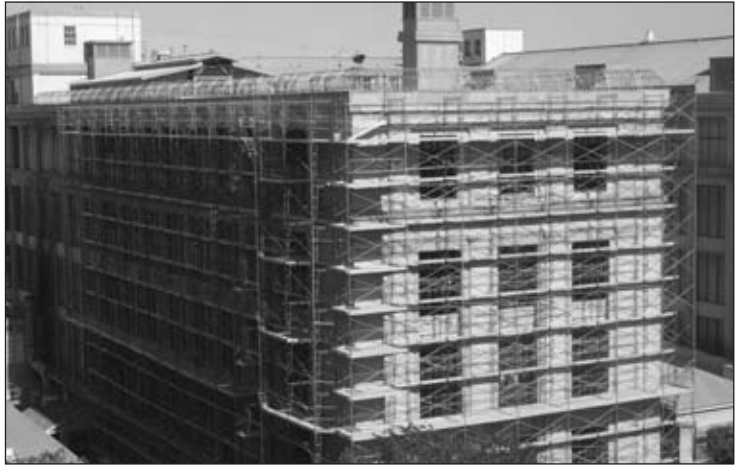
Limestone facade renovation underway at the Washington, DC facility.
