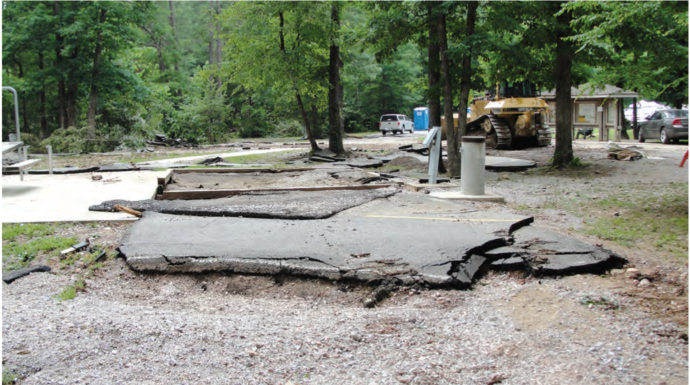
Figure 14. Remnants of the asphalt pavement in Area D of the Albert Pike campground.
