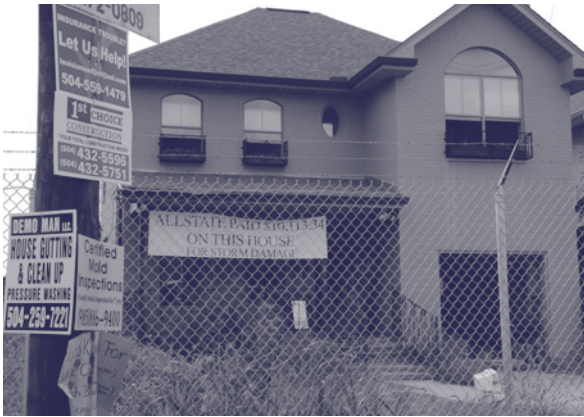
Flood-damaged home in Lakeview neighborhood, New Orleans, LA.
