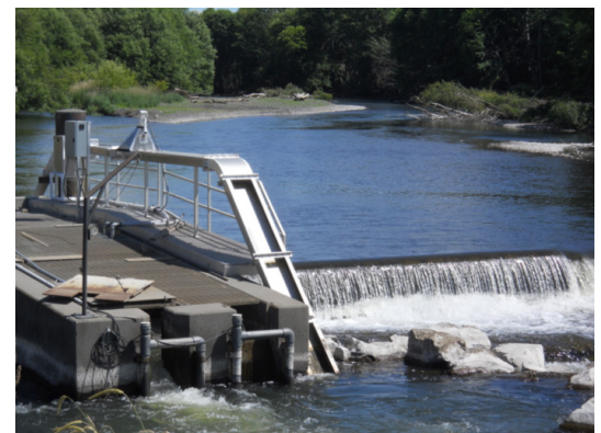
A newly-installed lamprey passageway in the Umatilla River, OR.
