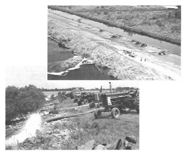
AND PORTABLE TRACTOR-POWERED PUMPS
