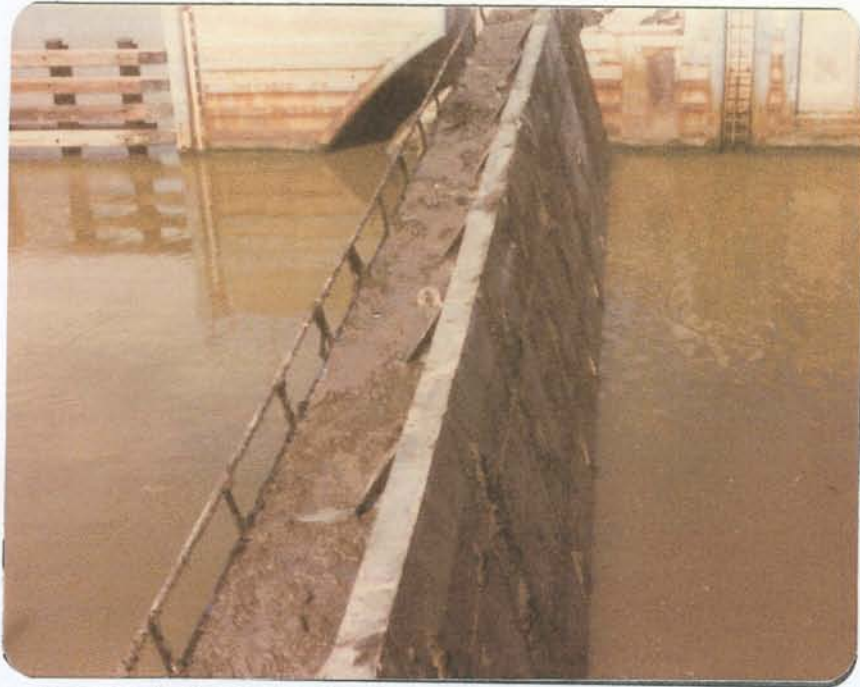
PHOTO NO. 1 - CORRODED WALL ARMOUR & LADDER: SOIL DEPOSITS ON FLAP GATE WALKWAY
