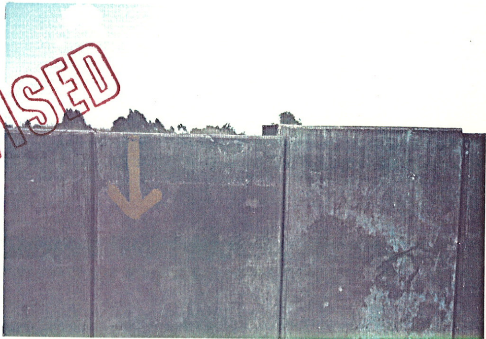
PHOTO NO. 4 - Differential settlement among members of concrete floodwall.
