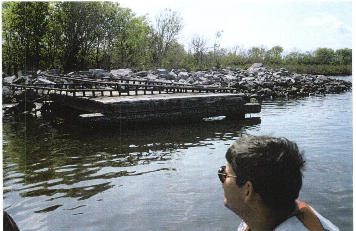
PHOTO NO. 24 – BOAT DOCK. NOTE STEEL FRAMES STORED ON DECK.
