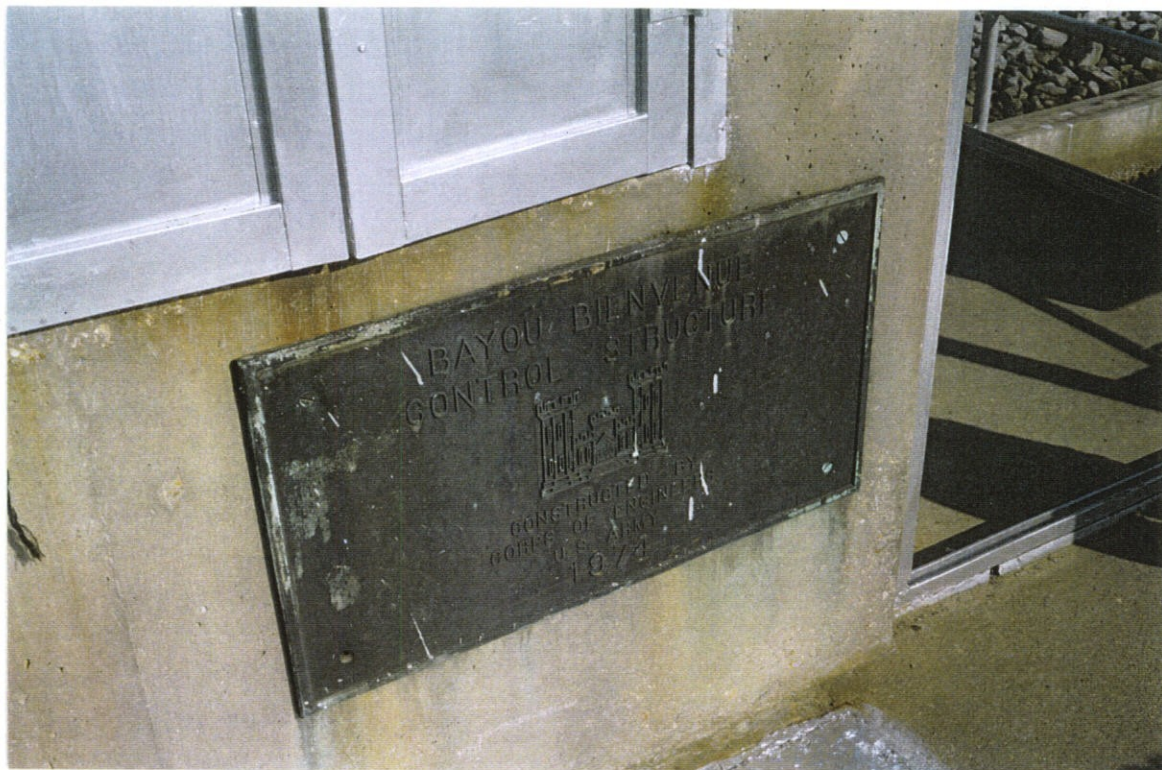
PHOTO NO. 2 – CONSTRUCTION PLAQUE ON THE NORTH CONTROL HOUSE.
