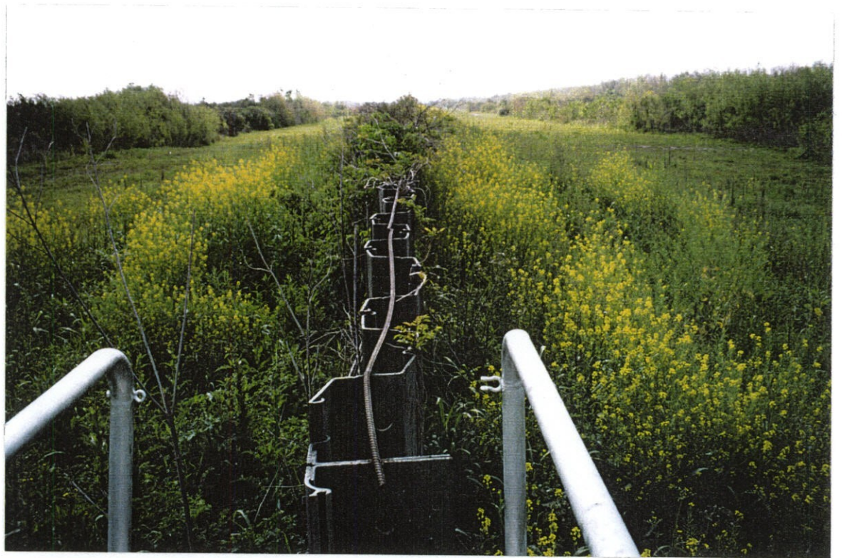
PHOTO NO. 19 – SHEET PILE FLOODWALL TIE IN TO LEVEE ON EAST SIDE OF STRUCTURE.
