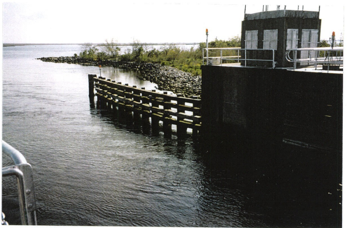
PHOTO NO. 22 – NORTHEAST TIMBER GUIDEWALL.
