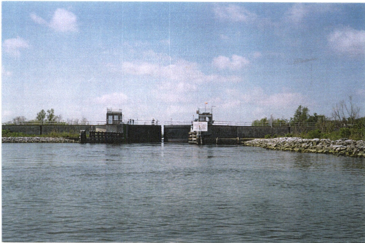
PHOTO NO. 1 – LOOKING WEST AT FLOODSIDE OF THE CONTROL STRUCTURE.
