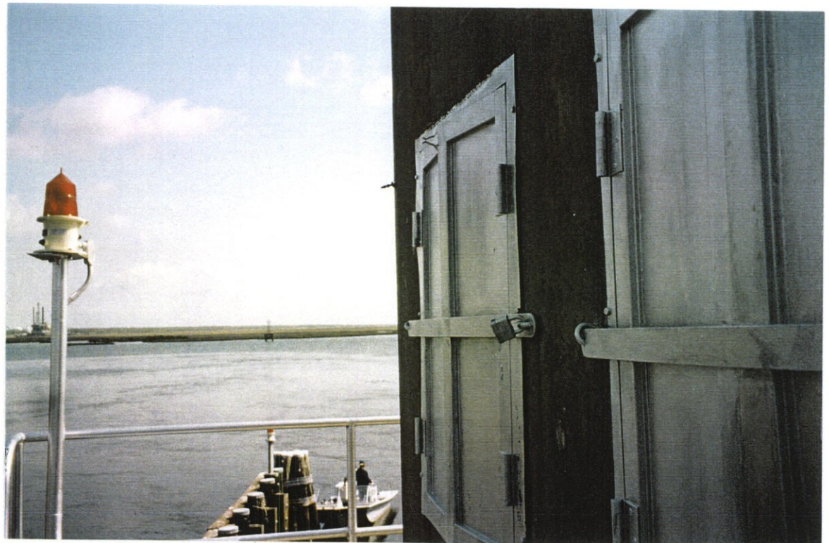
PHOTO NO. 14 – STEEL SECURITY SHUTTERS ON CONTROL HOUSE WINDOWS.
