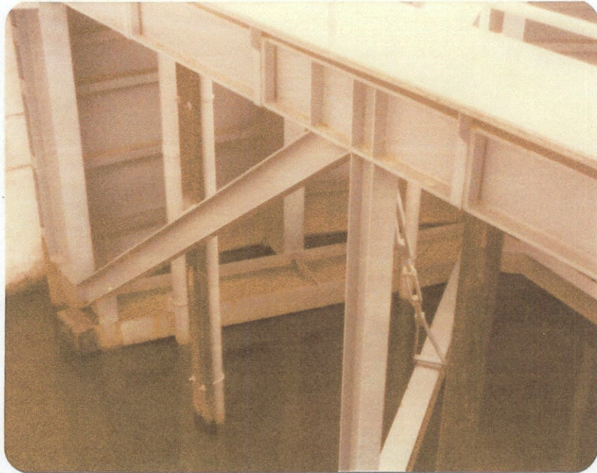
Photograph No. 1 - Spot Rust on Structural Steel Members of Sector Gate
