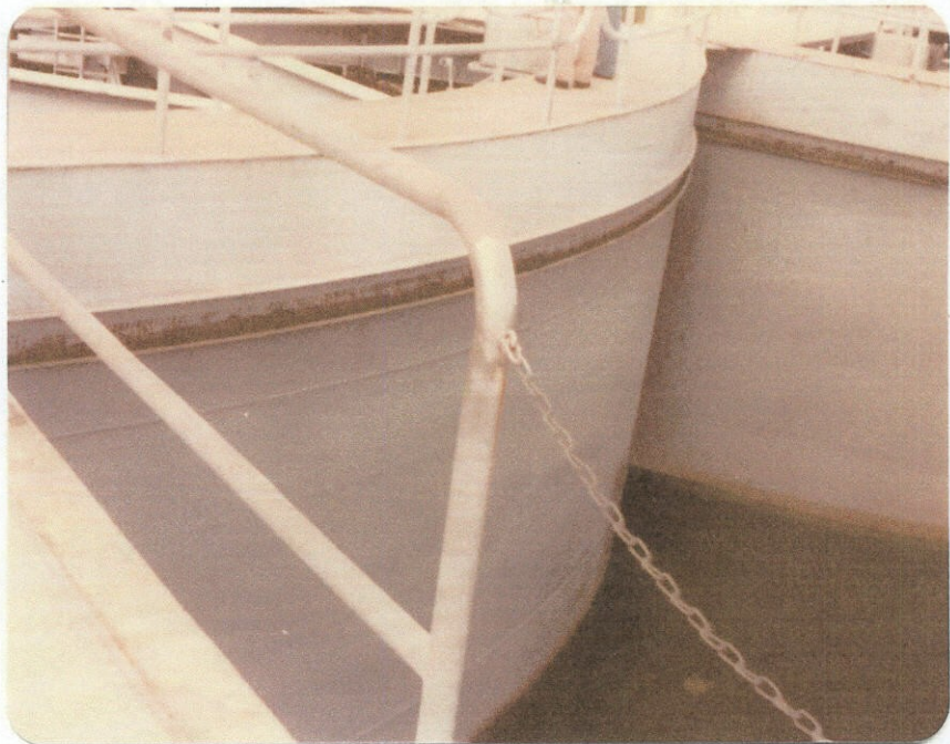
Photograph No. 4 - Corrosion on Sector Gate at Water Line
