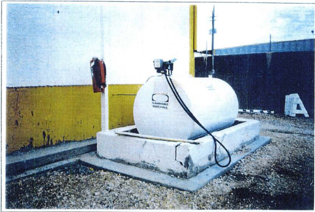
7. View to the northwest of a 500-gallon diesel tank which is used by the maintenance department of the New Orleans Port Authority.
