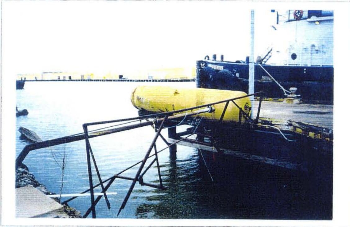
9. View to the southwest of a cylindrical above ground storage tank (Structure 41A) which was used to contain compressed air. The tank is abandoned with most of the associated piping disconnected.
