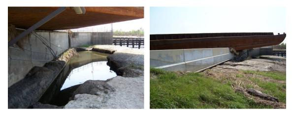
**4.** <u>**Bayou Dupre Control Structure**</u>. This control structure was damaged during the storm event. Adjacent sections of floodwall failed and the fill around other sections of floodwalls was eroded away due to overtopping. In addition there was damage to the mechanical and electrical systems that operate the sector gates.
