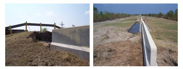
7. <u>Paris Road Closure Structure</u>. This closure structure was damaged during the storm event. There was scour of the structural backfill resulting from overtopping of the closure panels and additional damages due to impact from a loose barge.
