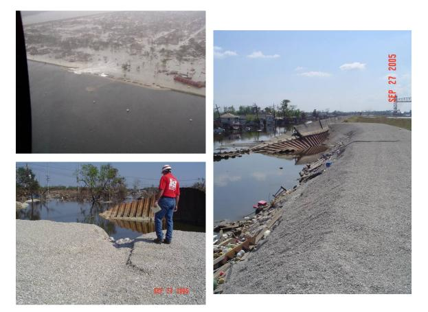
There are two segments of floodwall that were overtopped and the loss of foundation and backfill material on the protected side of the wall has caused some movement of the wall. These two segments are 200 ft. and 2000 ft. in length.
