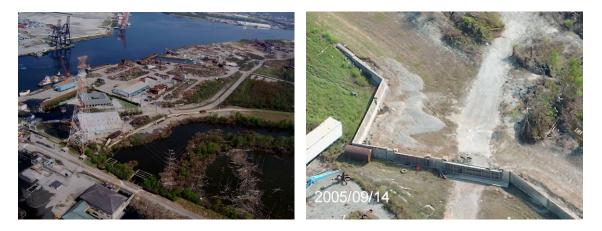
**9.** <u>Levee Damage Along Intracoastal Waterway</u>. There are small areas of scour on the backside of the levee between STA. 65+008 and STA. 277+20. This scour was the result of localized overtopping of the levees in this reach.
