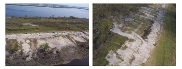
There is 2,300 ft. of levee in this reach that has some damage (assume that 50% of the levee section gone).
