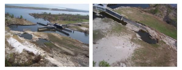
**IHNC Floodwall**. There are two segments of floodwall just north of the IHNC Lock on the east side of the canal that were overtopped and breached by the storm event. These two segments are 350 ft. and 850 ft. in length. The overtopping caused severe damage to these segments and they will need to be replaced.
