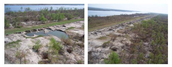
There is 2,500 ft. of levee from Bayou Dupre to STA 1007+91 that lost approximately 8' of elevation (assume that 50% of the levee section is gone)
