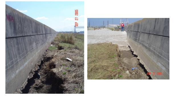
There are two segments of floodwall that were overtopped with loss of foundation and backfill material on the protected side of the wall. There has not been any movement of these two segments. These segments are 620 ft. and 2000 ft. in length.
