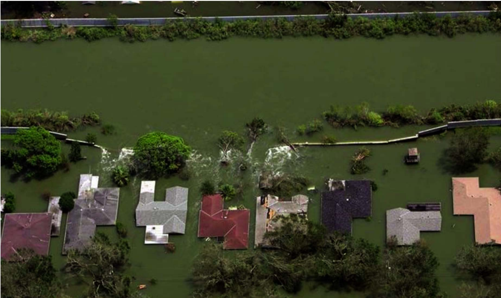
Figure 2 – The north breach at the London Avenue canal occurred at 7:00 AM to 8:00 AM on August 29, 2005. The breach, on the west side of the canal, is approximately 410 feet wide.
