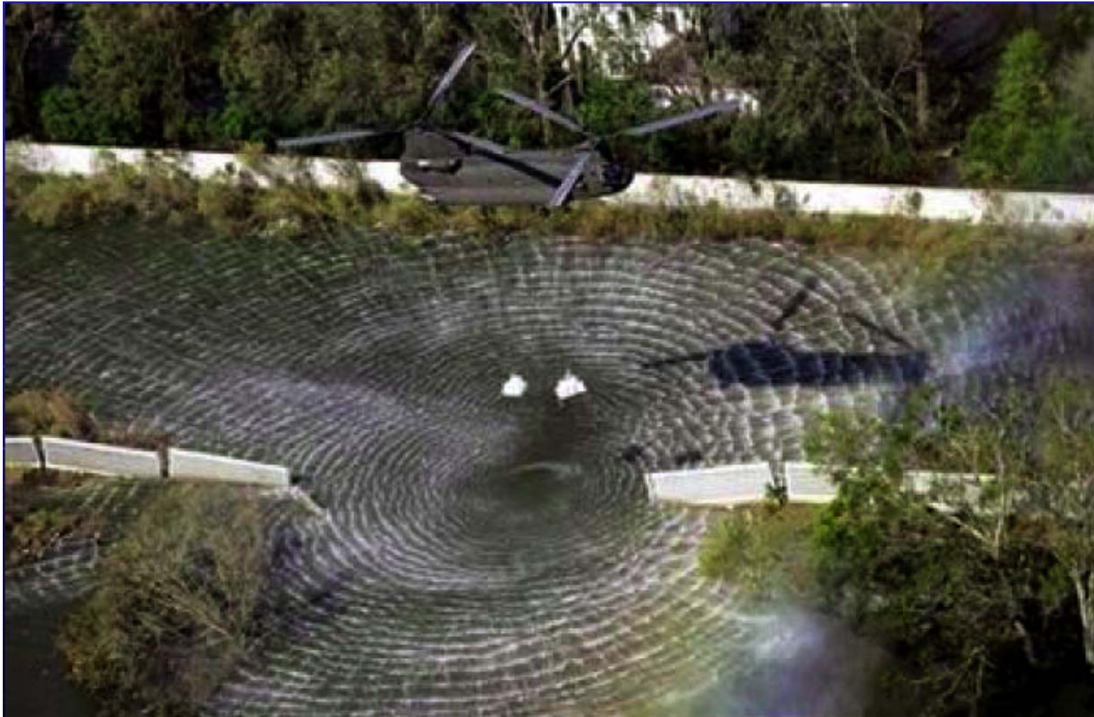
Figure 1 – The south breach at the London Avenue canal occurred at 6:00 AM to 7:00 AM on August 29, 2005. The breach, on the east side of the canal, was approximately 60 feet wide.
