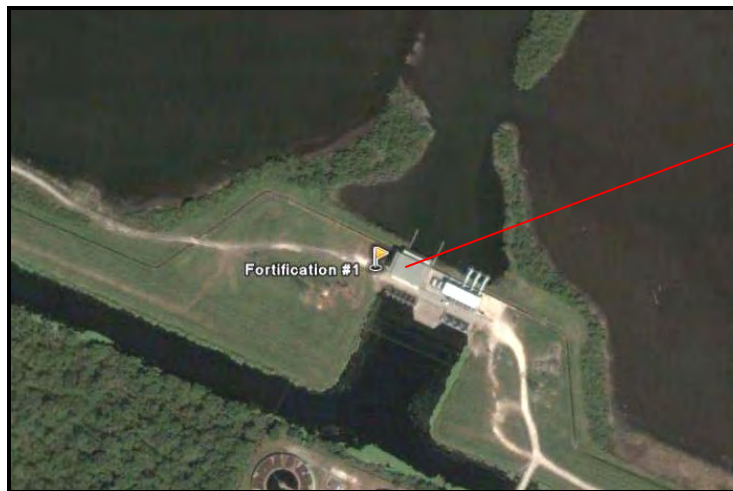
Pre-Hurricane Katrina – Arial view of pump station
