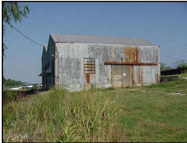
Pre-Hurricane Katrina – View from the south end
