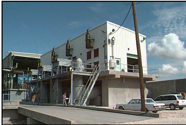
Post-Hurricane Katrina – View from the Inlet Canal
