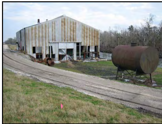
Post-Hurricane Katrina – View to the South
