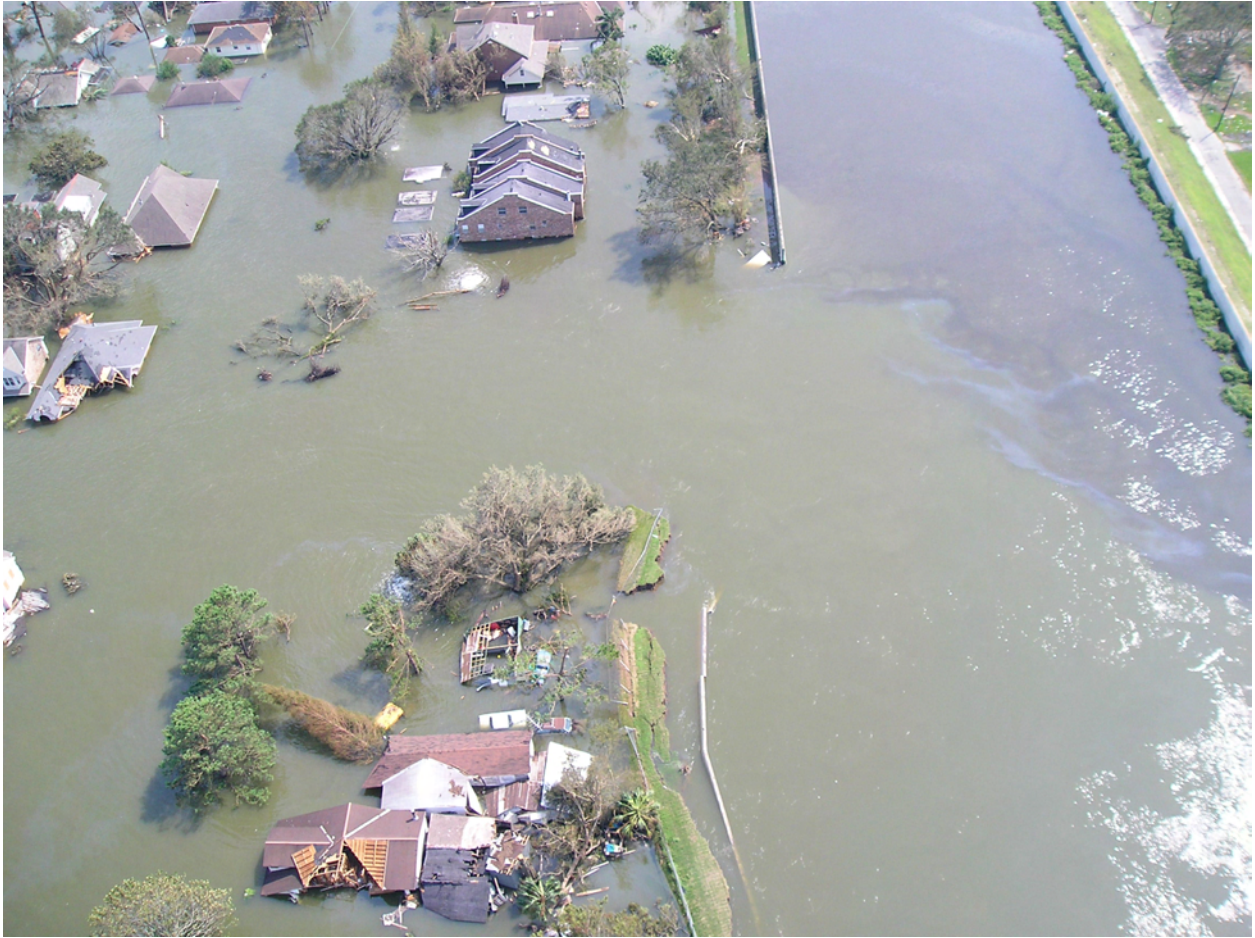
Figure VI-3. Aerial photograph of the 17th Street Canal breach showing I-wall and embankment translation
