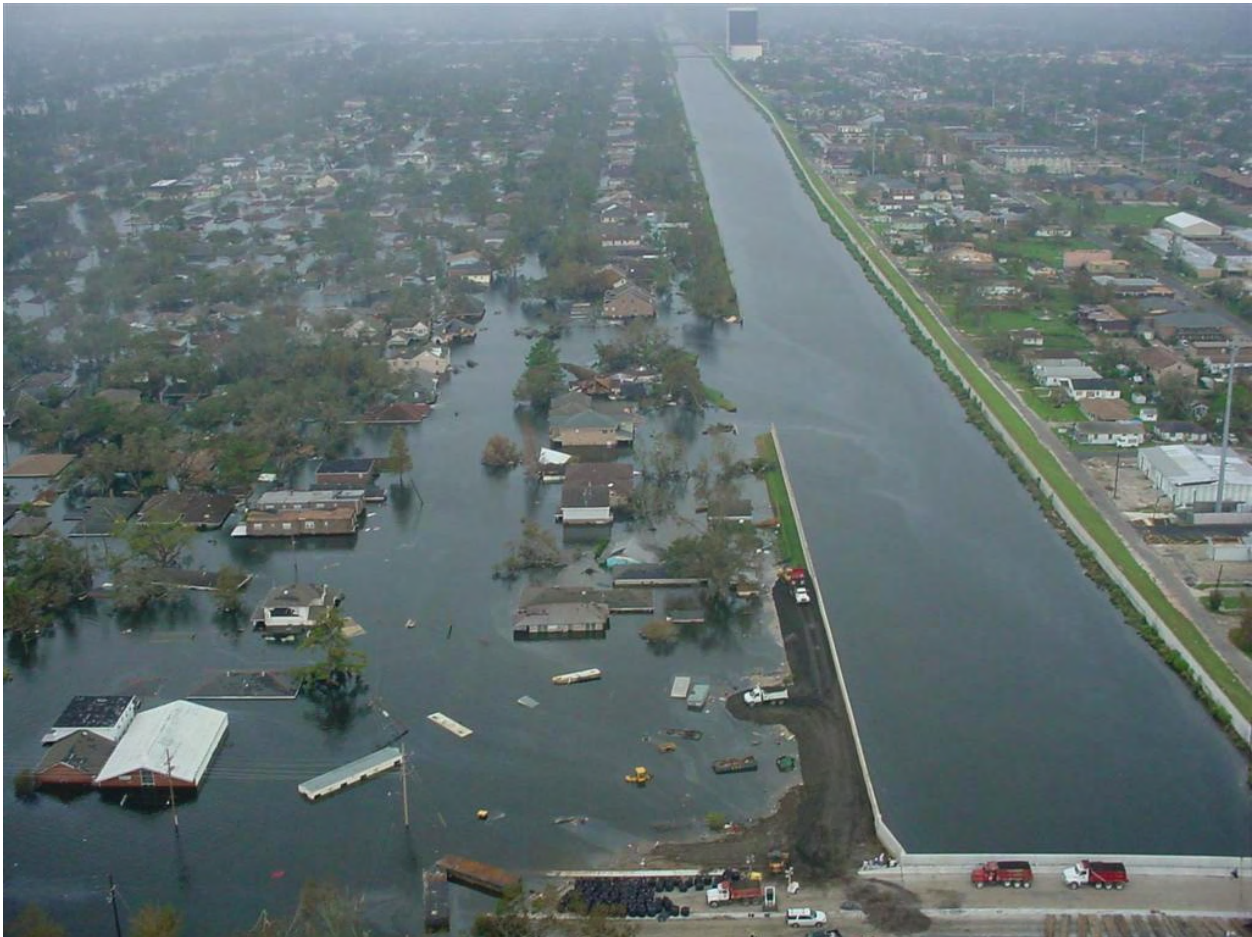
Figure VI-1. Aerial photograph of the 17th Street Canal breach looking south from Old Hammond Road bridge
