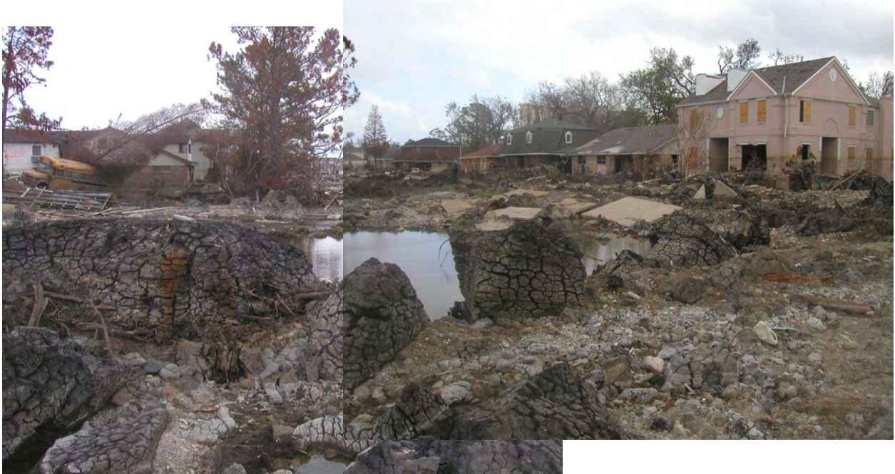
Figure VI-7. Peat blocks from the levee embankment
