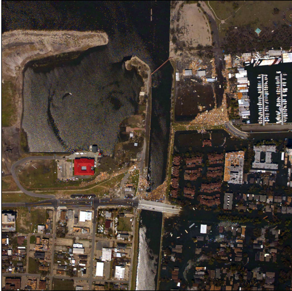
Figure V-82. Debris field against Hammond St. Bridge
