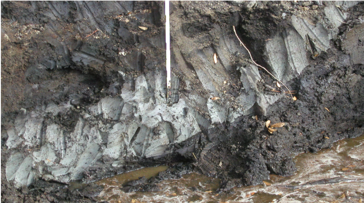
Figure VI-9. Exposed failure plane
