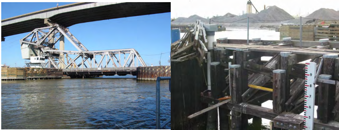
Figure III-26. (Left) IHNC Almonaster Bridge—low chord elevation 3.51 ft NAVD88 (2004.65). (Right) Leveling to USGS recording gage and Orleans Levee District staff gage on I-10 bridge over IHNC
