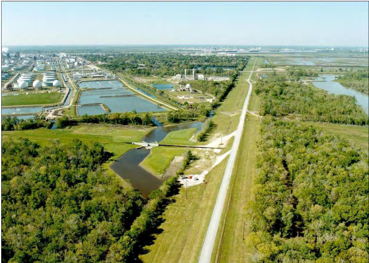
Figure 5. Typical New Orleans levee.
