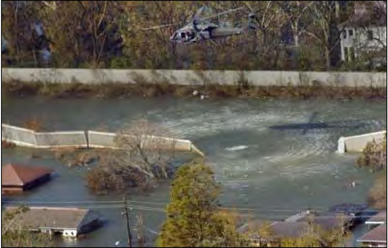
Figure 12. Katrina damage to concrete capped I-wall.
