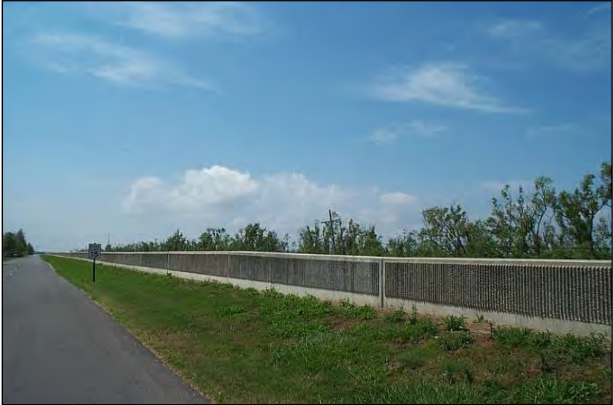
Figure 9. Concrete capped I-wall.
