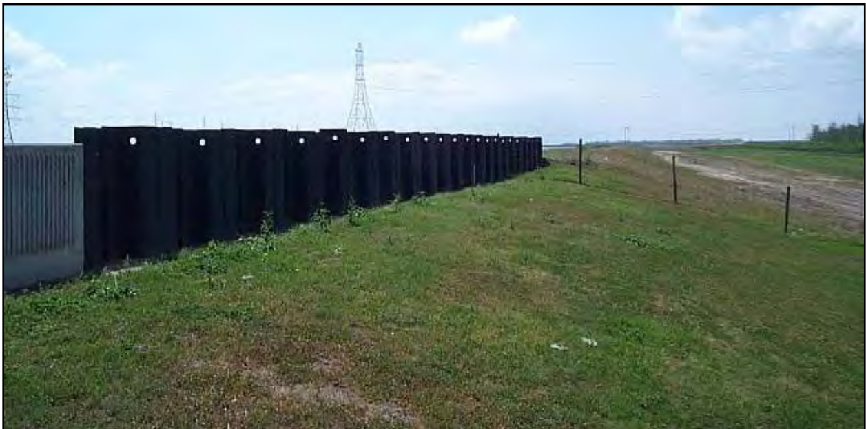
Figure 19. I-wall transition to concrete structure and levee.
