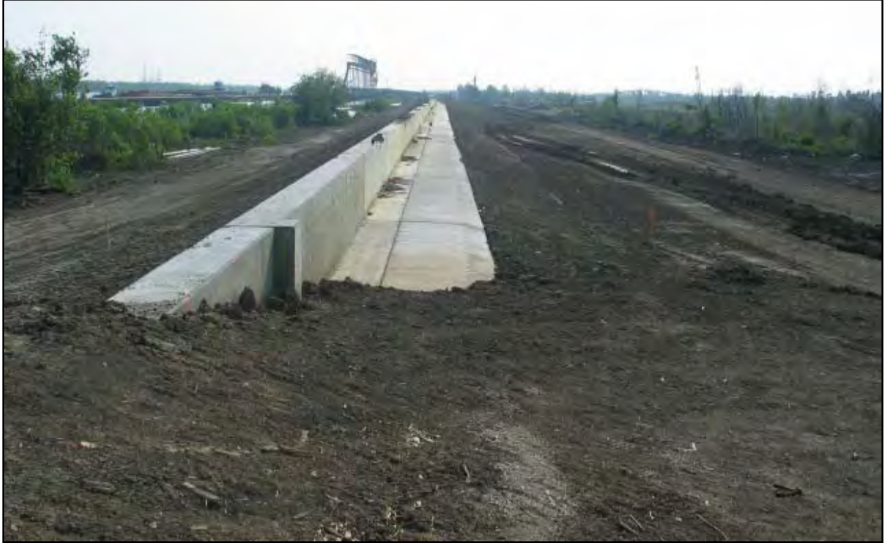
Figure 15. Typical L-wall.
