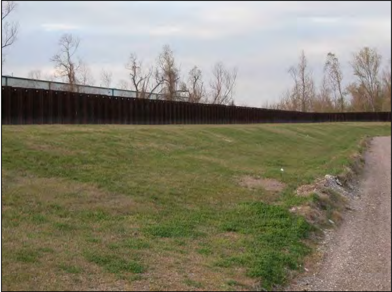
Figure 7. Typical sheet-pile I-wall.
