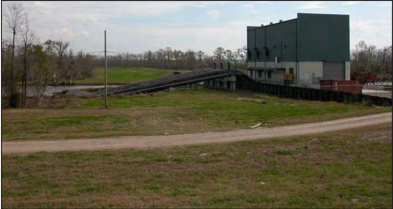
Figure 18. Local pump station.
