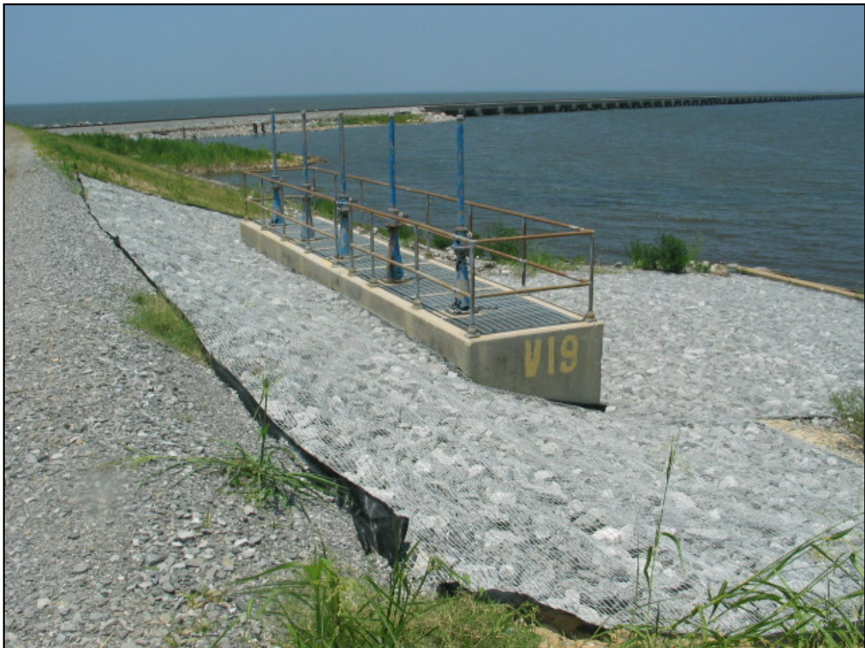
Figure NOE 27. Scour Repairs to Drainage Structure Headwalls (Note: Reach NOE10 drainage structure repairs – typical)
