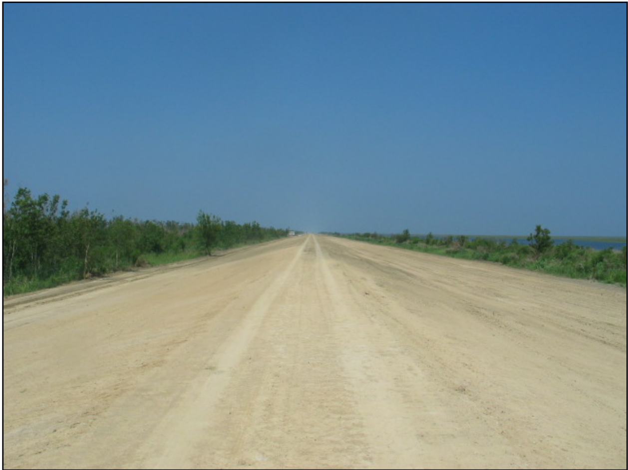
Figure NOE 29. New Levee Along the GIWW (East Back Levee)
