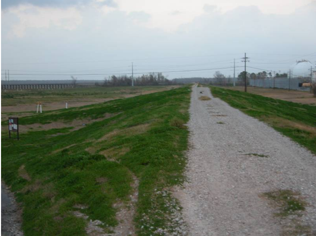
Bonnet Carre Guide Levee Looking North from the Spillway gates
