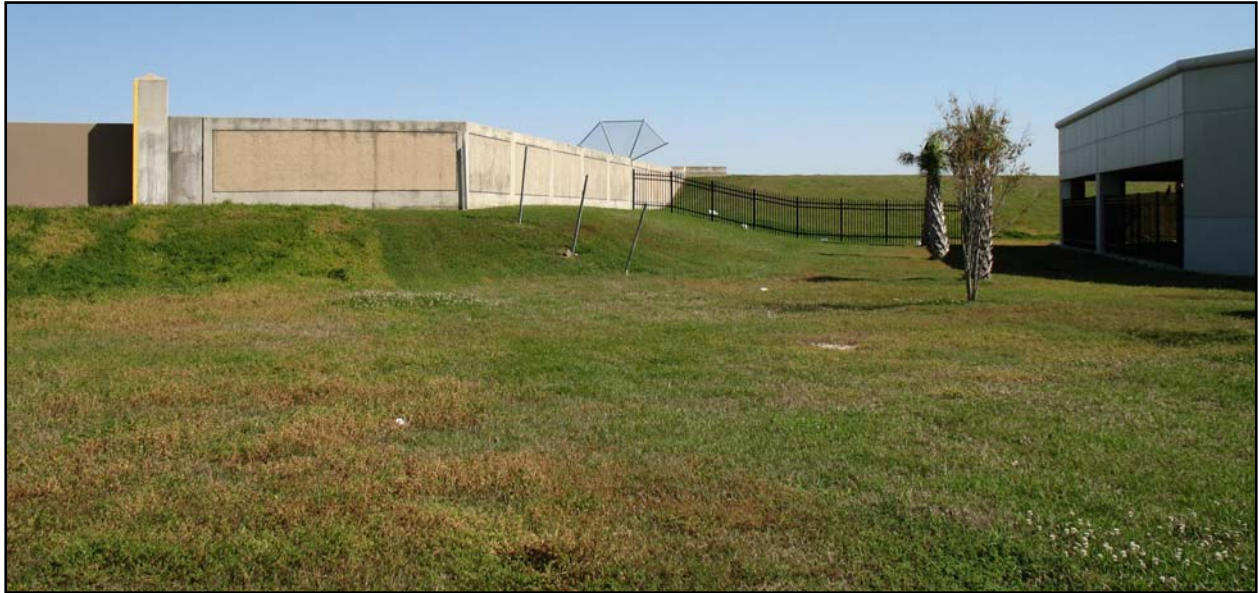
Figure 7. Floodwall and Levee behind the University of New Orleans
