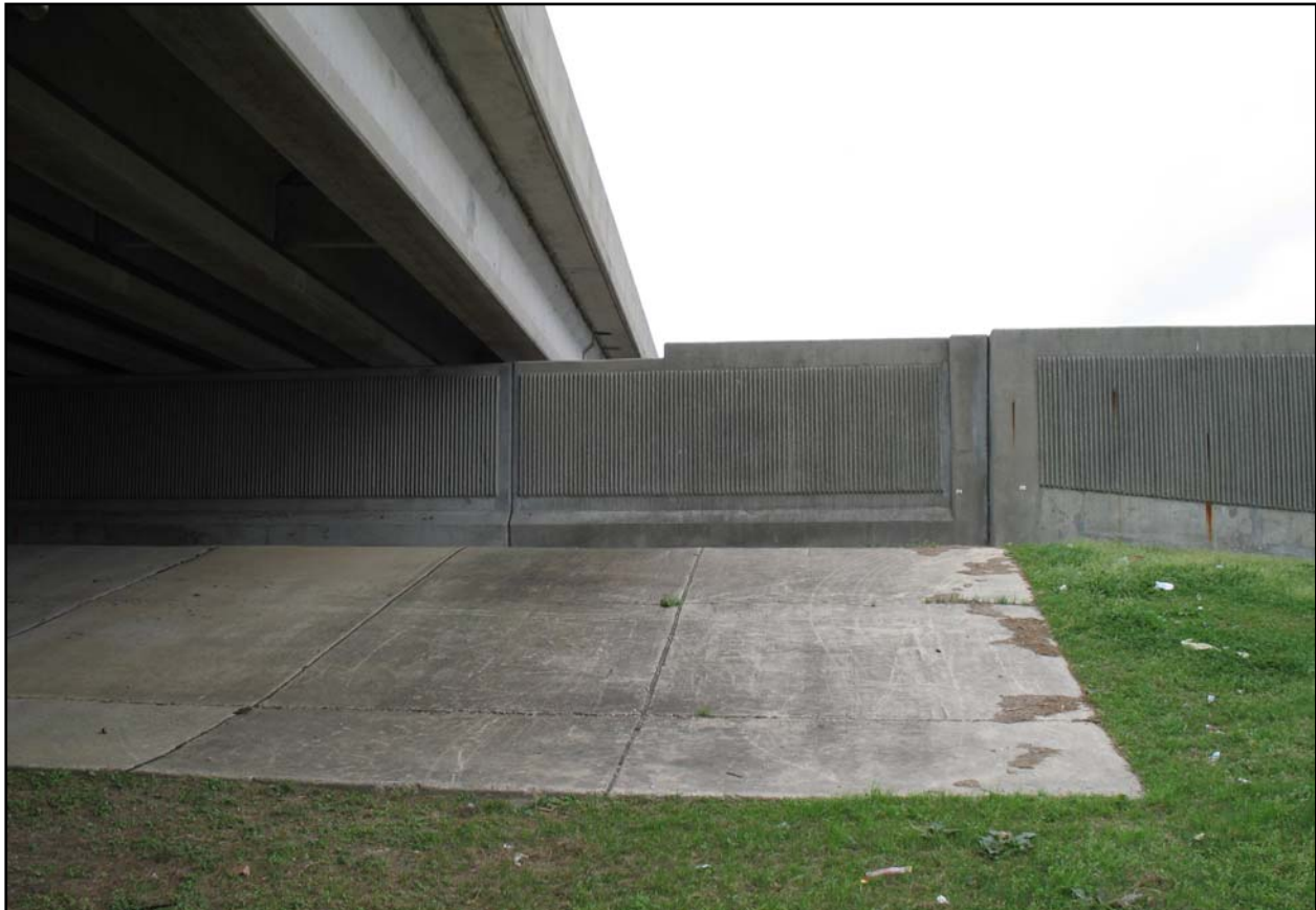
Typical T-Wall Transition in the Floodwall in Kenner Return Levee
