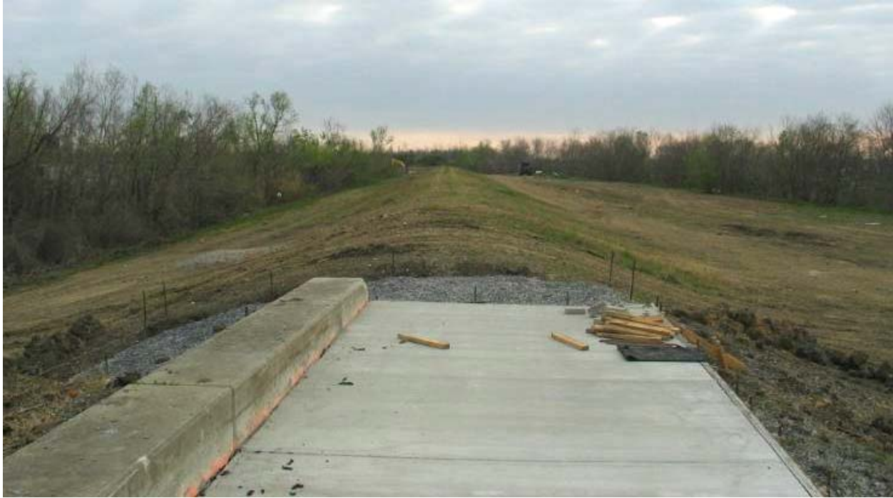
Figure STB 9. Beginning of Reach STB5 at end of I-wall (Note TFG improvements to Reach STB4 in foreground)
