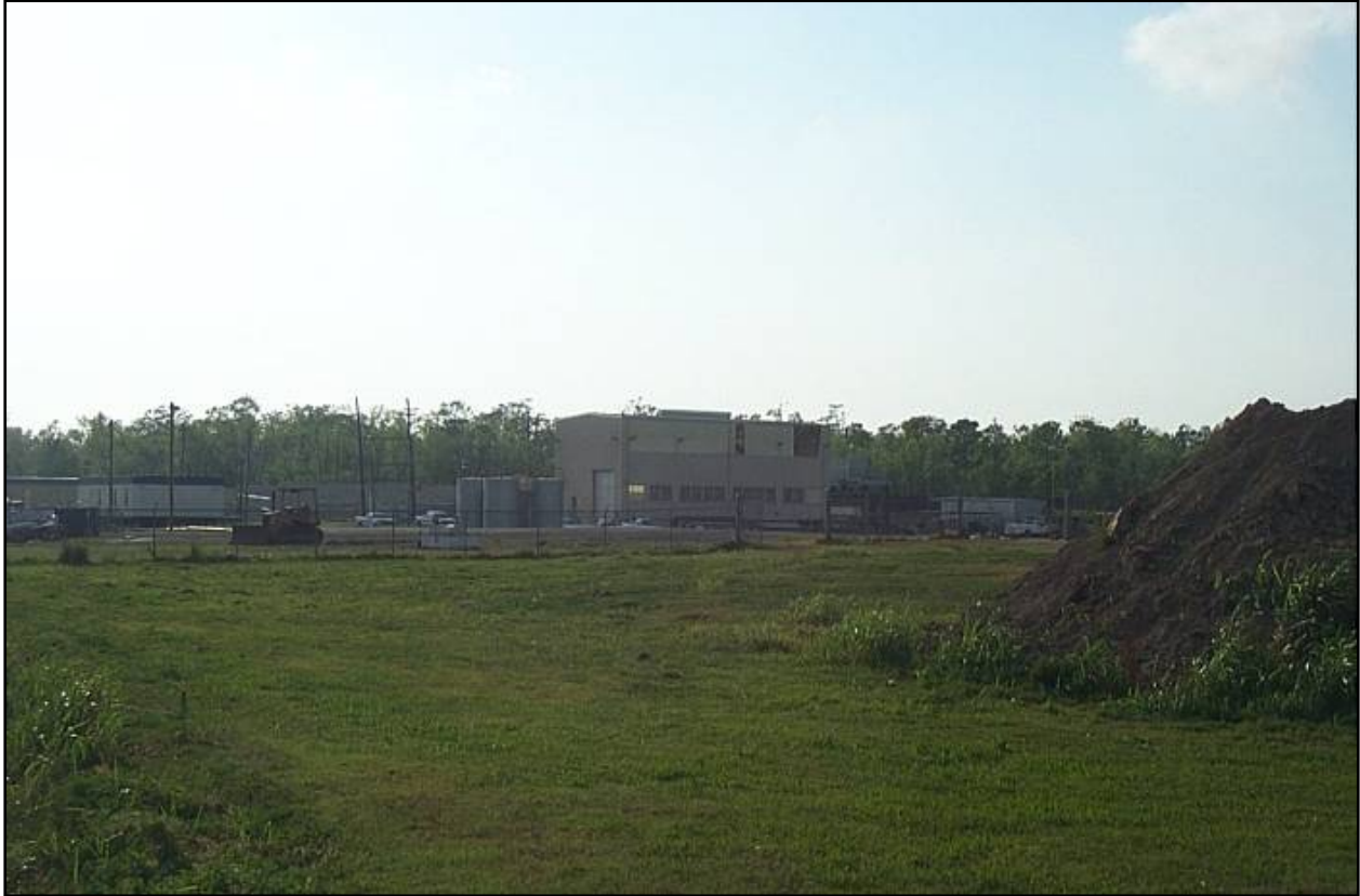
Ames Pump Station
