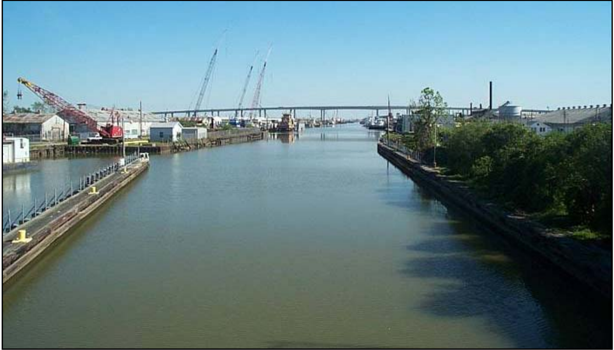
Looking south down Harvey Canal from Hwy 45 Bridge near Harvey Lock
