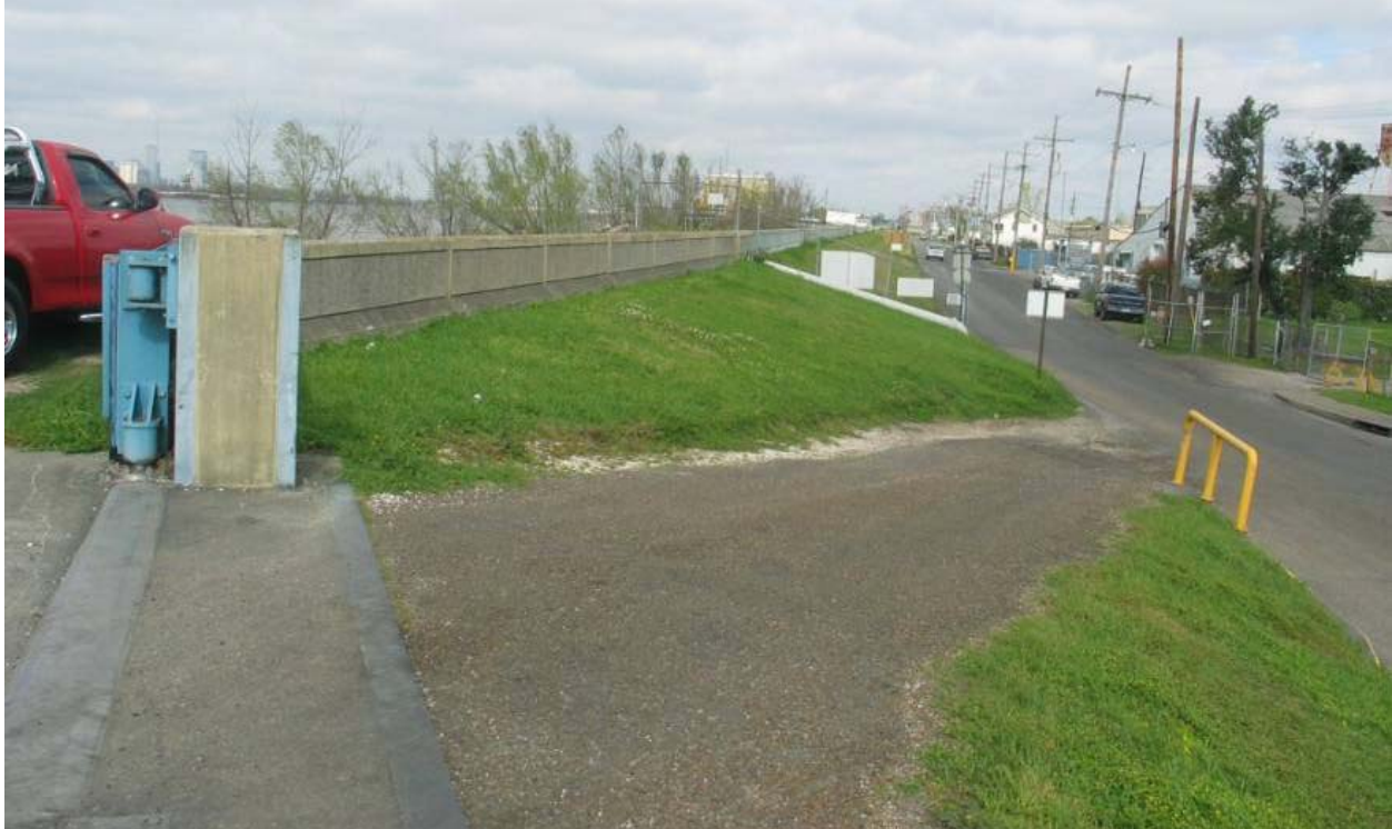
Figure STB 21. Concrete capped I-wall near Domino Sugar Plant (closure represents key point within this reach)
