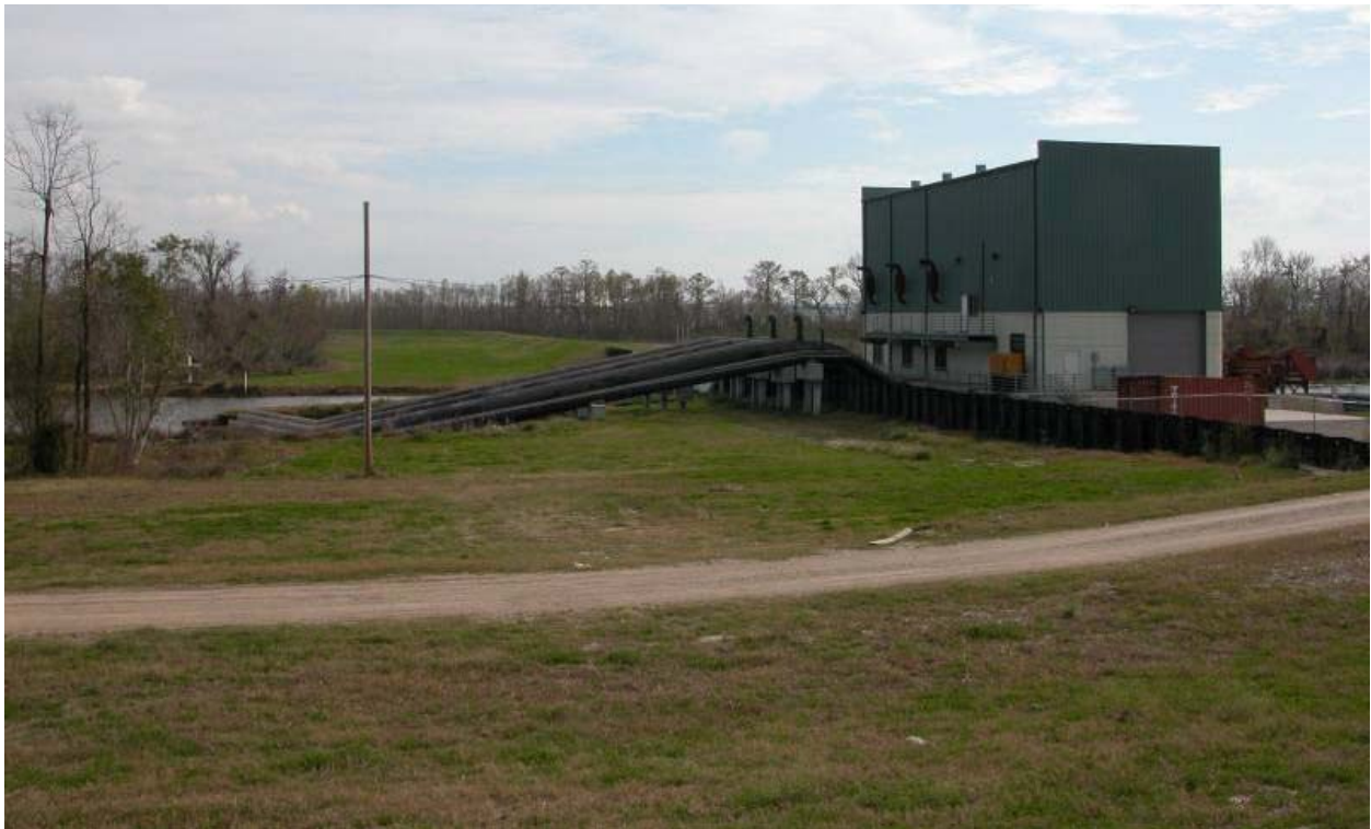
Trepagnier Pump Station
