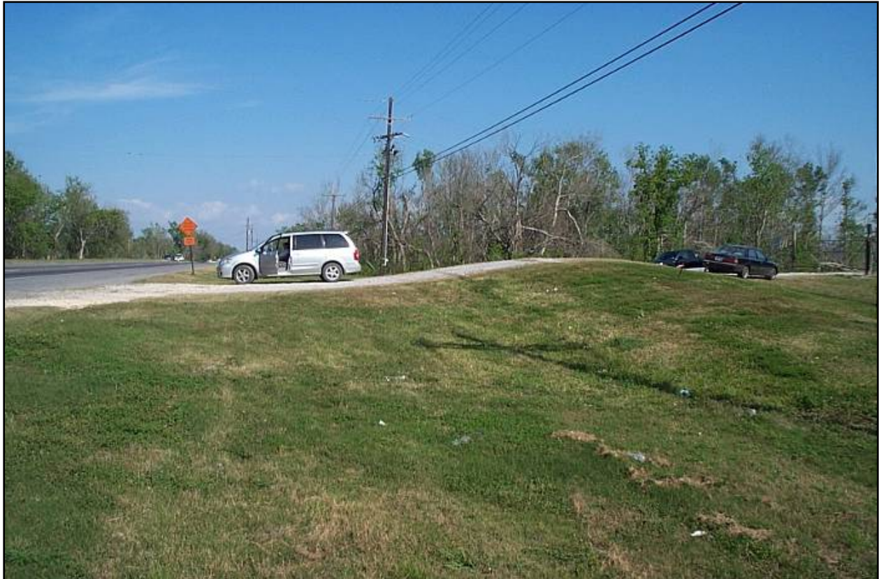
Levee begins at Hwy 90
