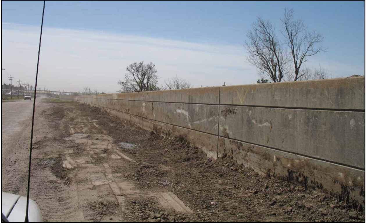
Repair to Scour Along Floodwall.
