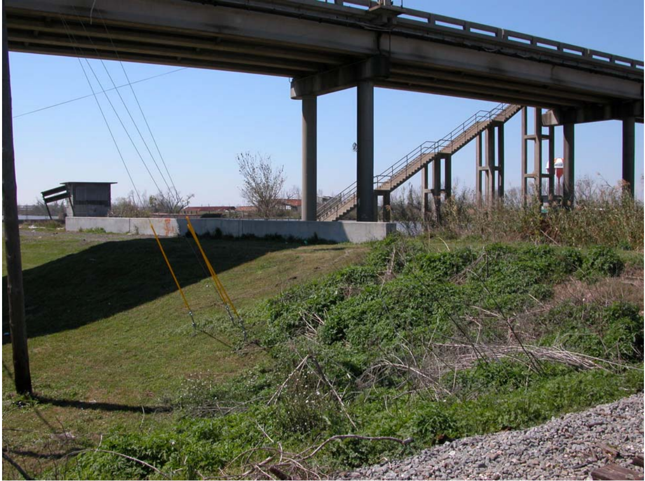
Highway 23 Bridge over GIWW and Levee
