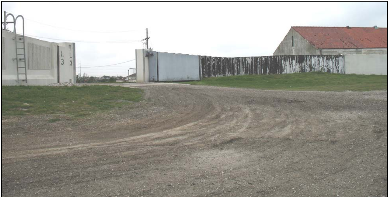
Gate L3 – Duncan Canal Pump Station
