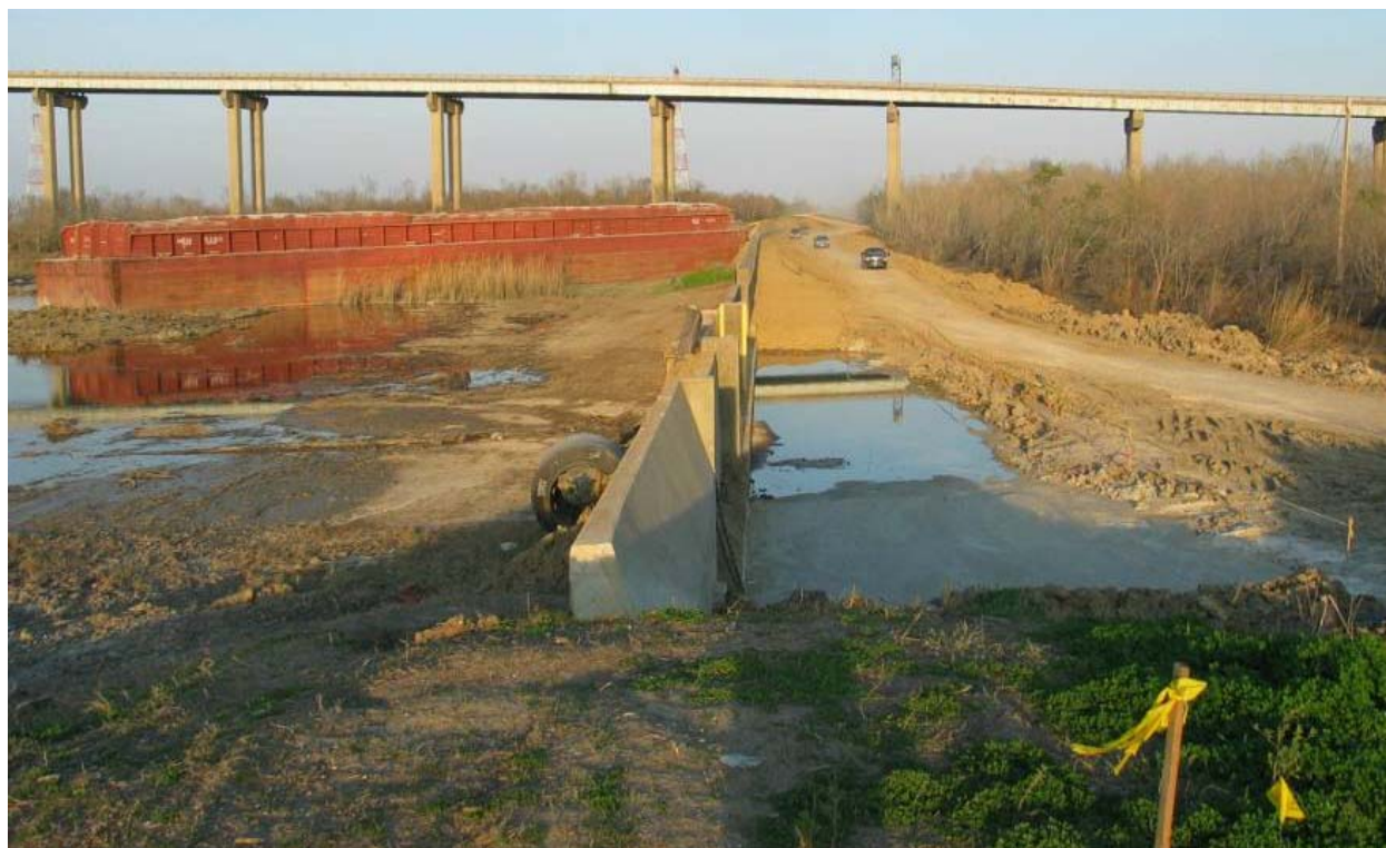
Figure STB 10. Paris Road Floodwall (Reach STB8) (looking east from the west end of the floodwall)
