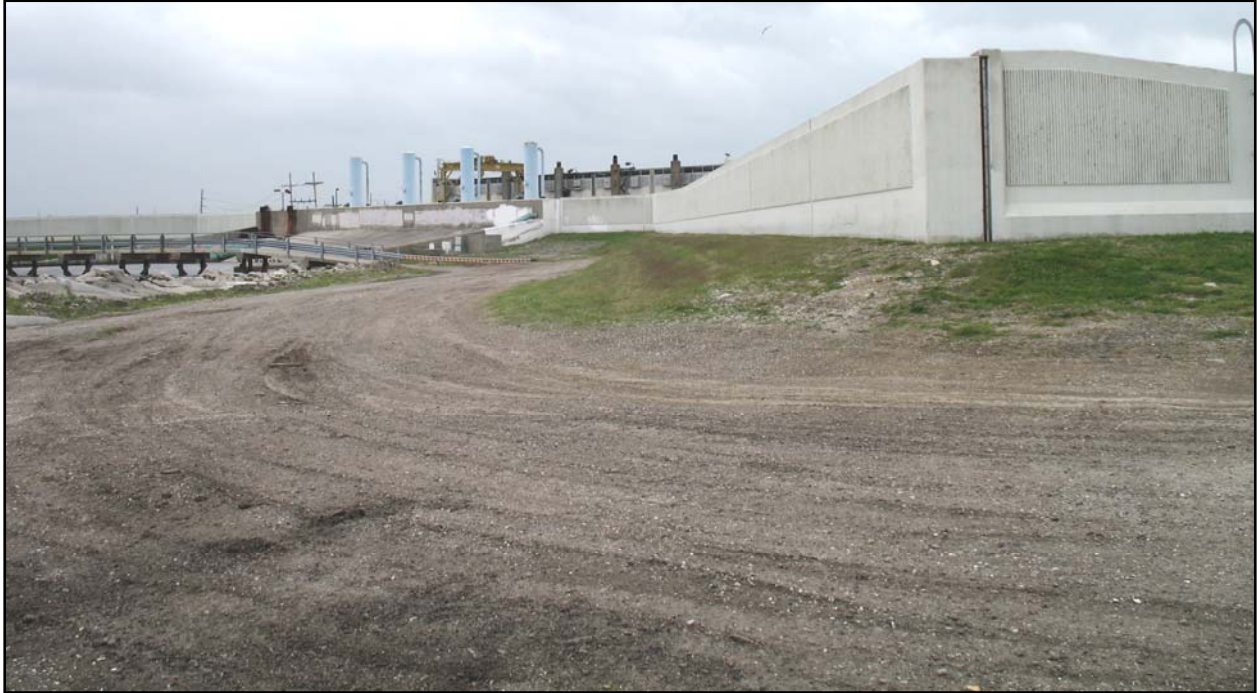
Duncan Canal Pump Station
