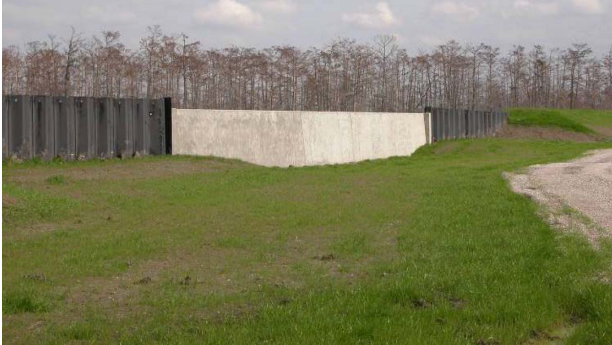
Gulf South Pipeline Crossing
