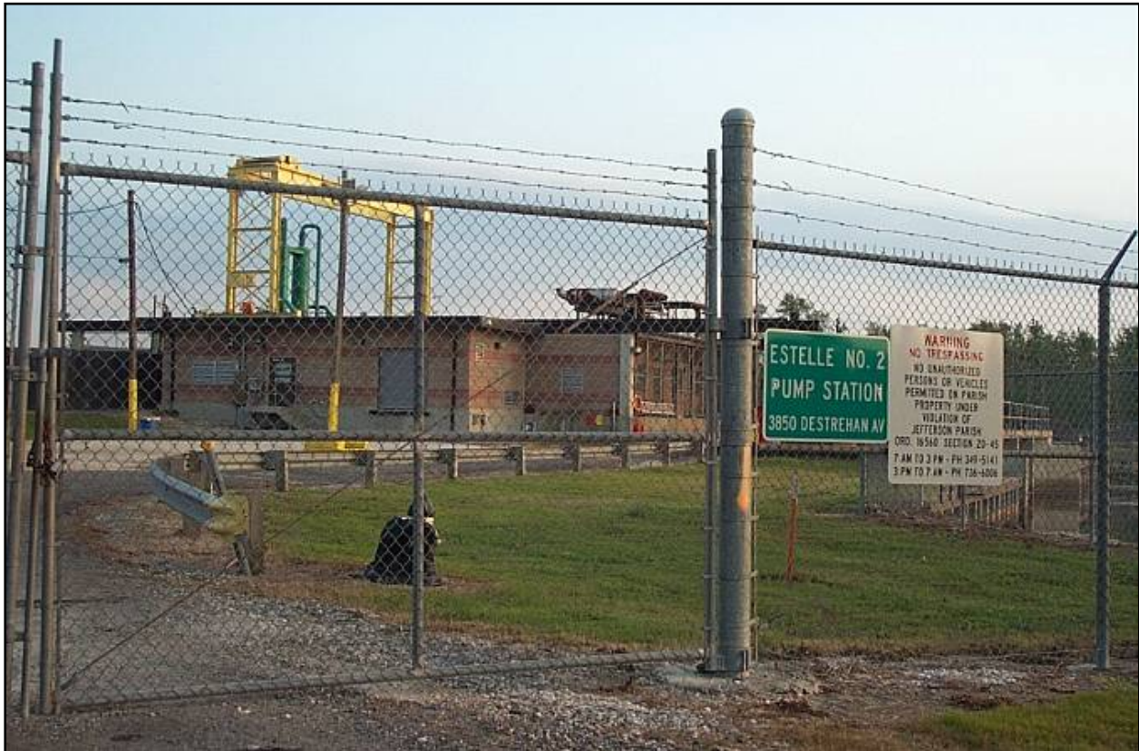
New Estelle Pump Station
