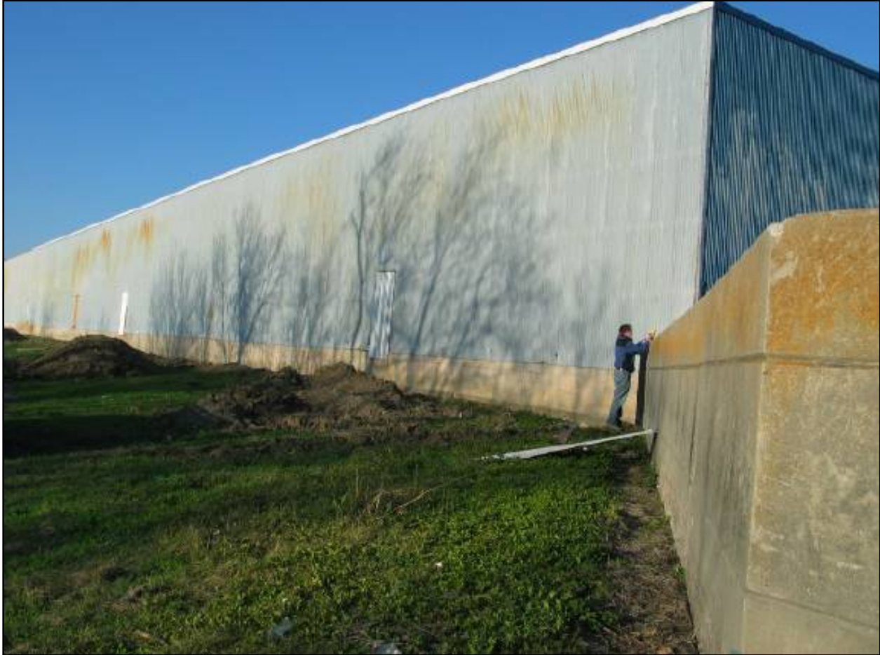
Figure NOE 20. Floodwall Serves as Building Foundation (Dupuy Storage Facility – IHNC East)
