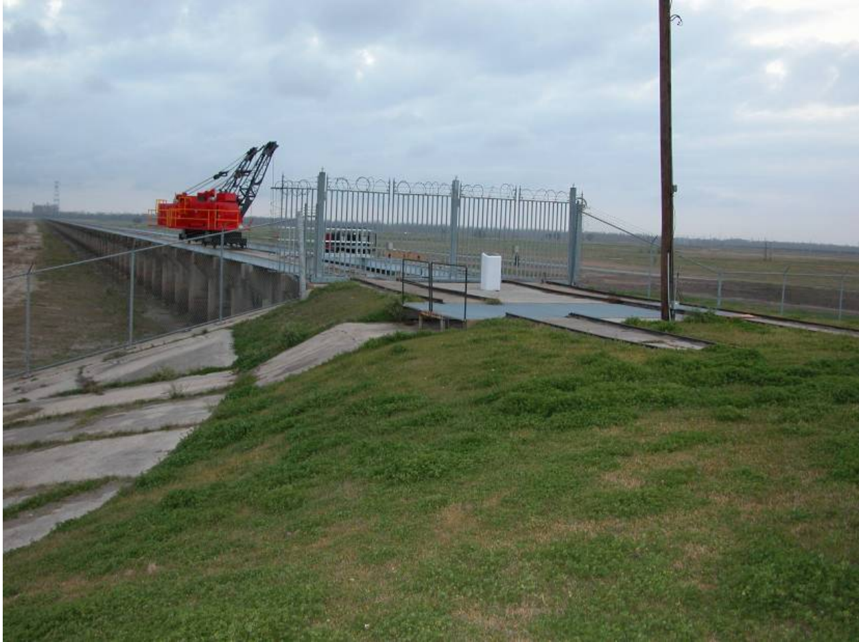
Bonnet Carre Spillway intersection with guide levee
