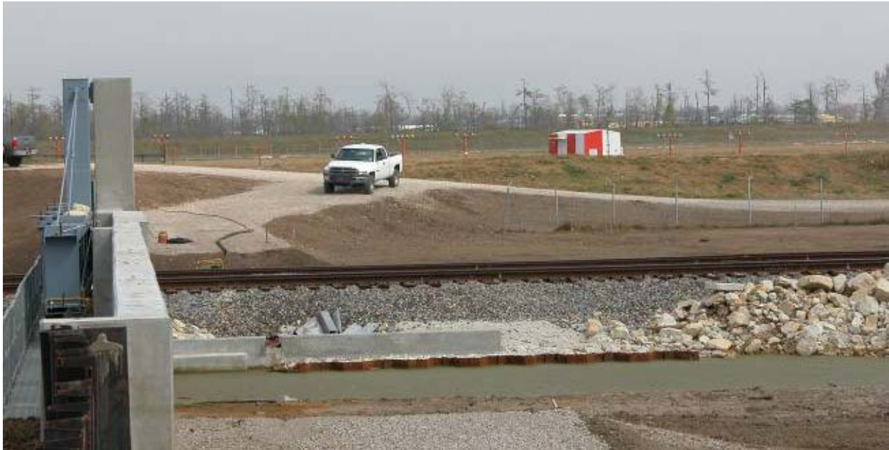
Railway Gated Crossing at Airport Levee (not constructed during Katrina). HPS joins Airport Levee just north of the Railway Gated Crossing
