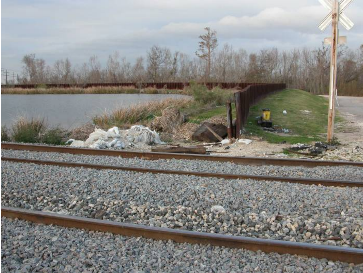
Floodwall as it turns south just north of the railroad crossing
