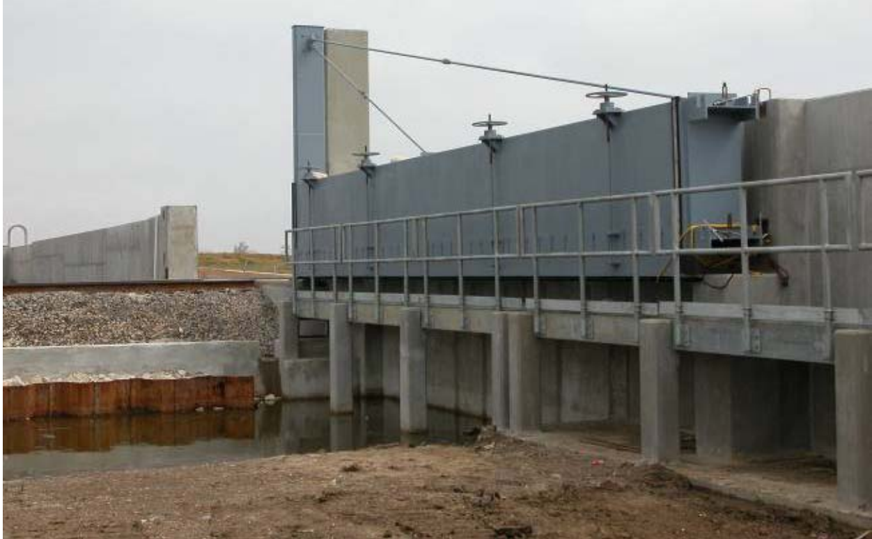
Railway Gated Crossing at Airport Levee (not constructed during Katrina)
