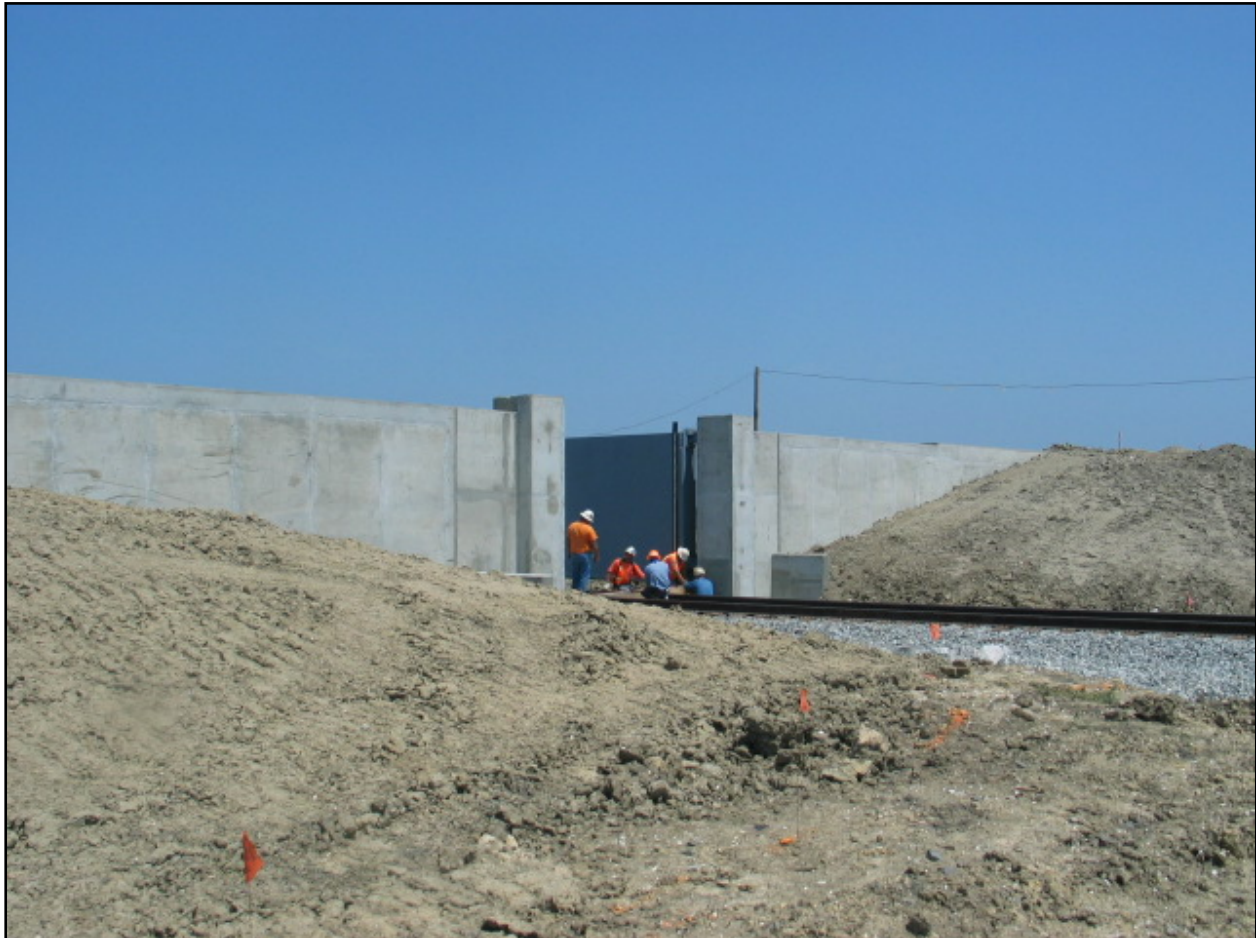
Figure NOE 28. Reconstruction of CSX Railroad Closure Structure
