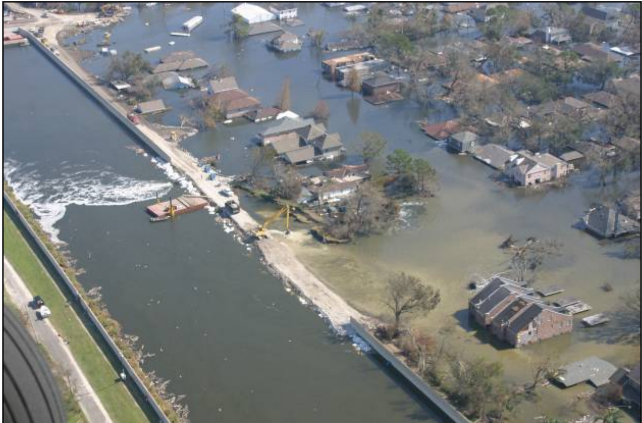
Figure 3. Breach in the 17th Street Canal
