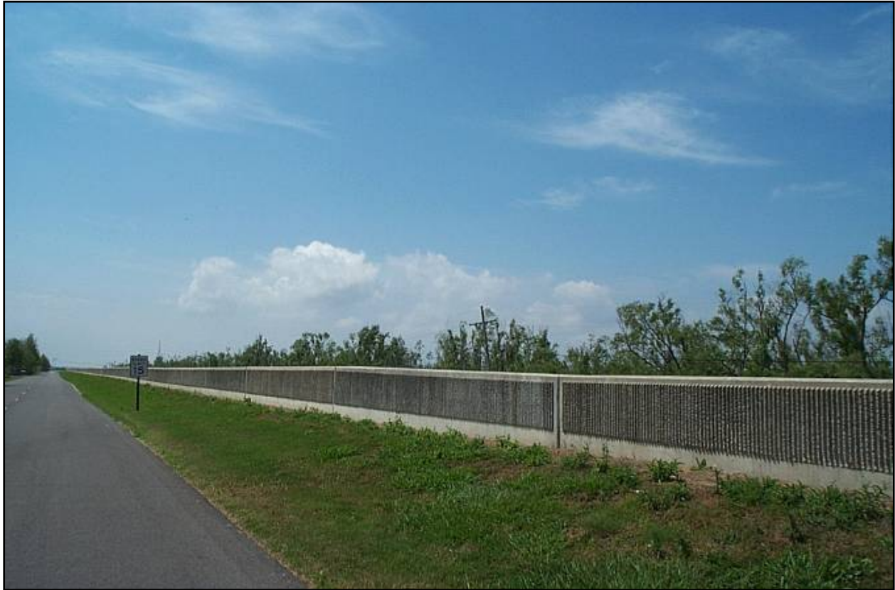
Concrete capped I-wall at the Segnette State Park
