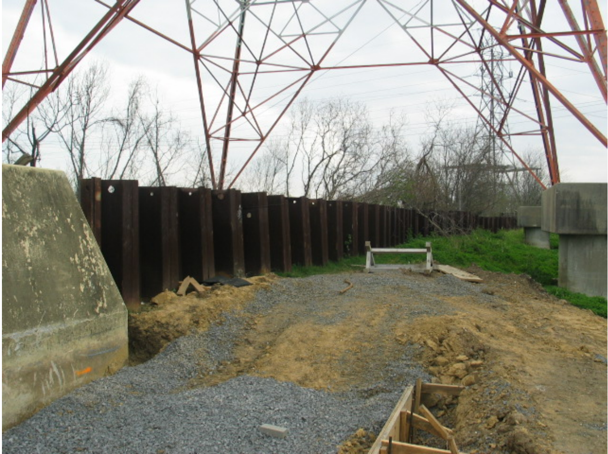
Figure STB 24. Close-up of beginning of interior local levee
