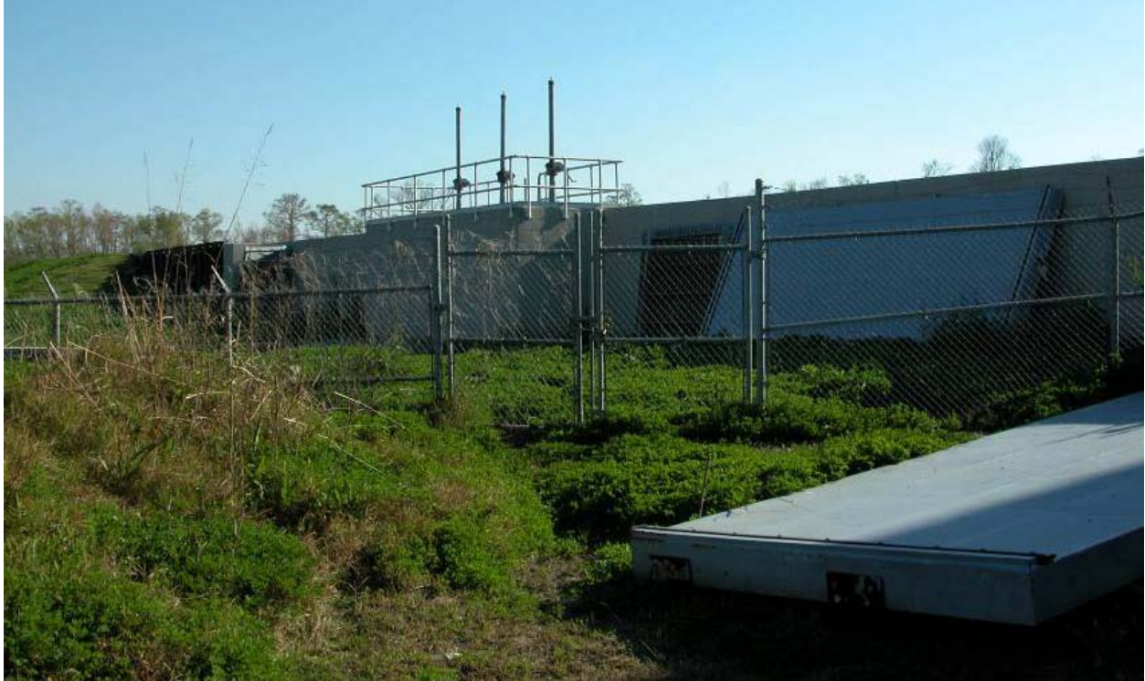
Trepagnier Drainage Structure
