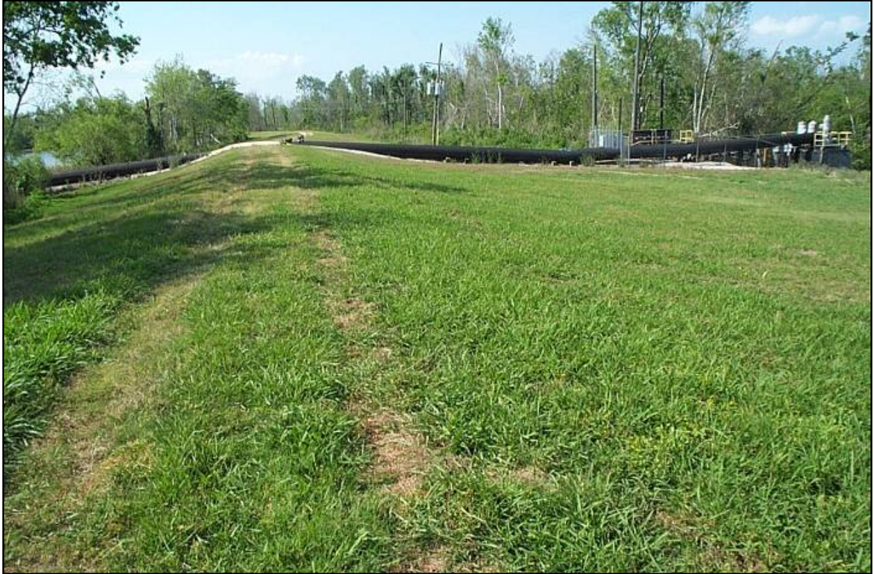
Typical levee in this area
