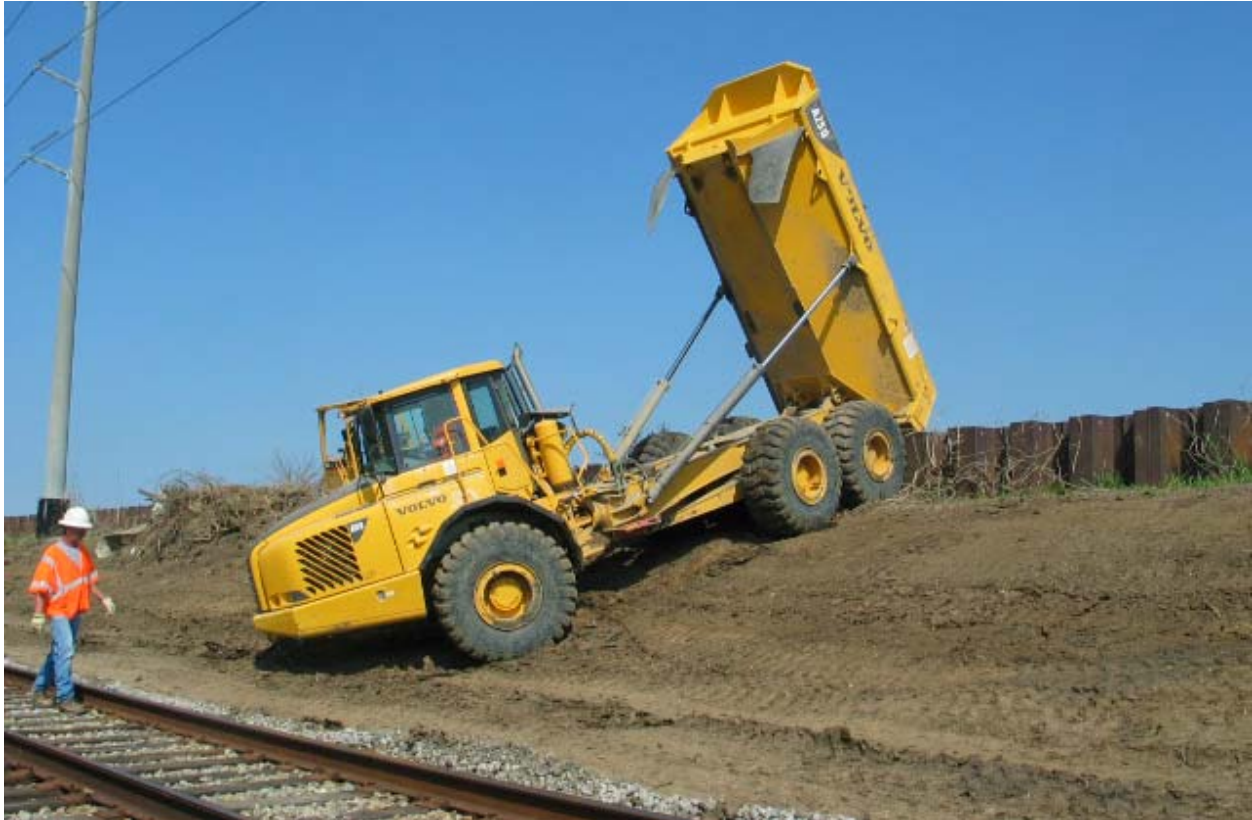
Figure STB 39. Repairs to interior local levee along Reach STB33 near parish border (Note: This section is being returned to pre-Katrina conditions)
