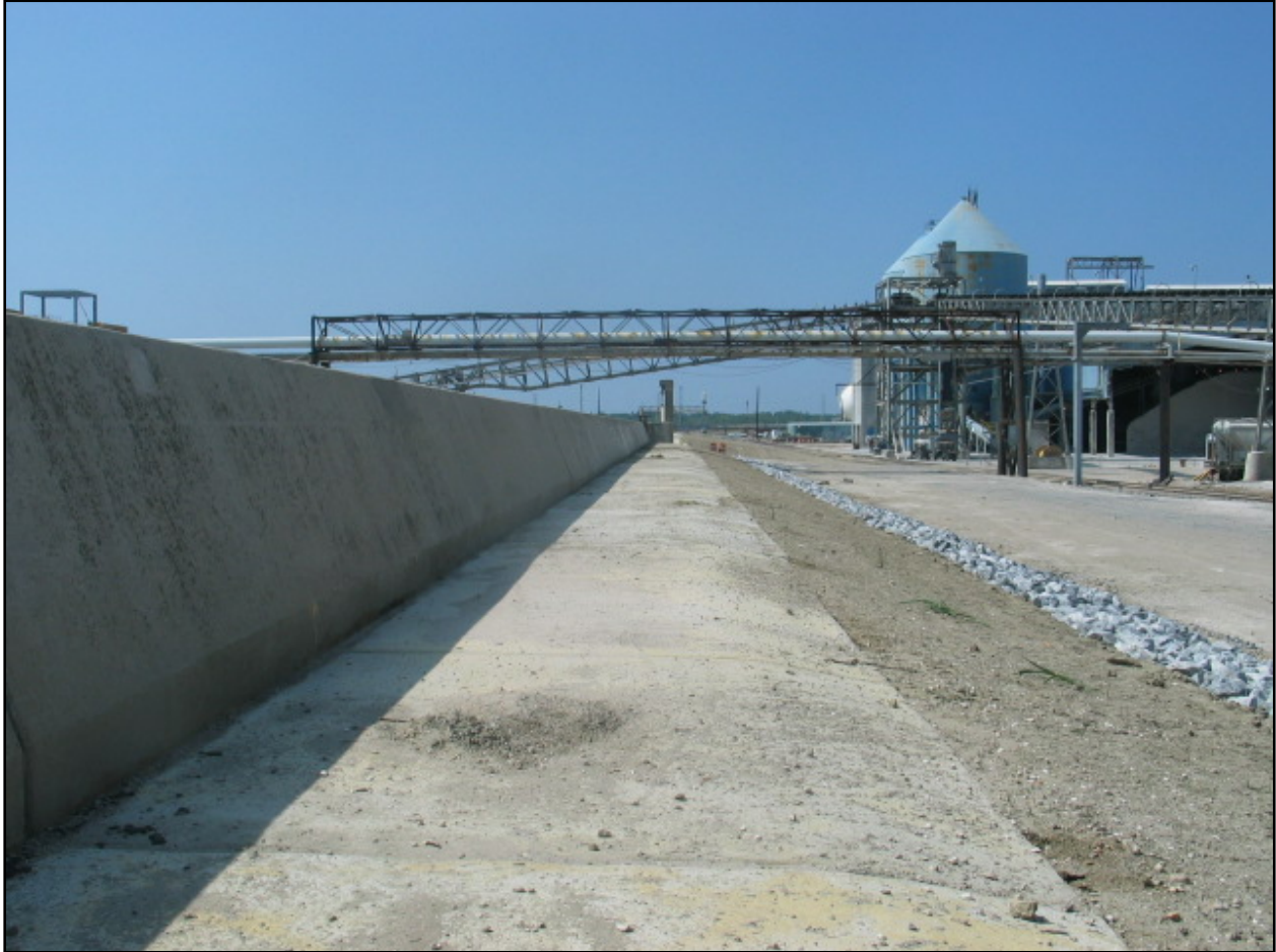
Figure NOE 31. Michoud Canal Floodwall Improvements
