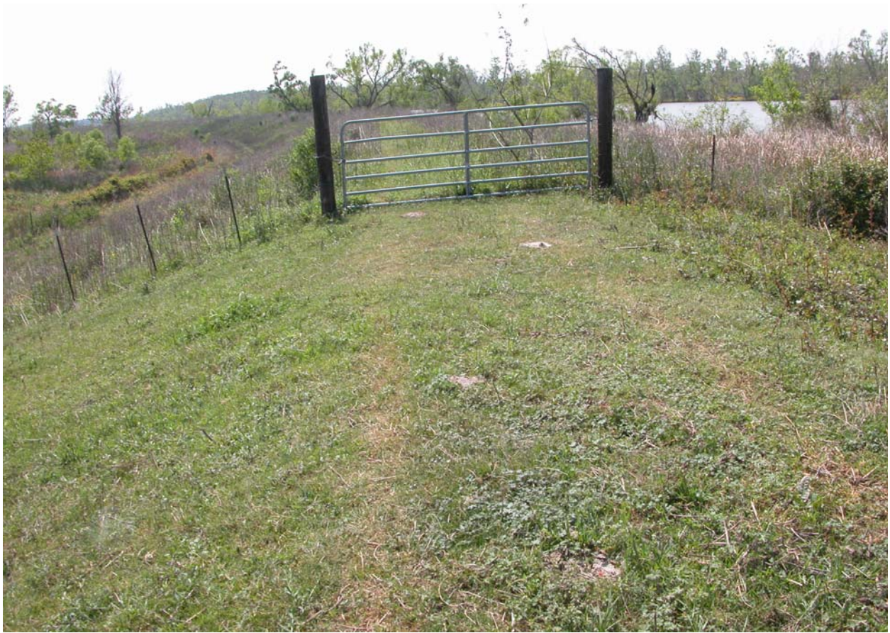
Typical levee section. Numerous gates across levee to contain cattle
