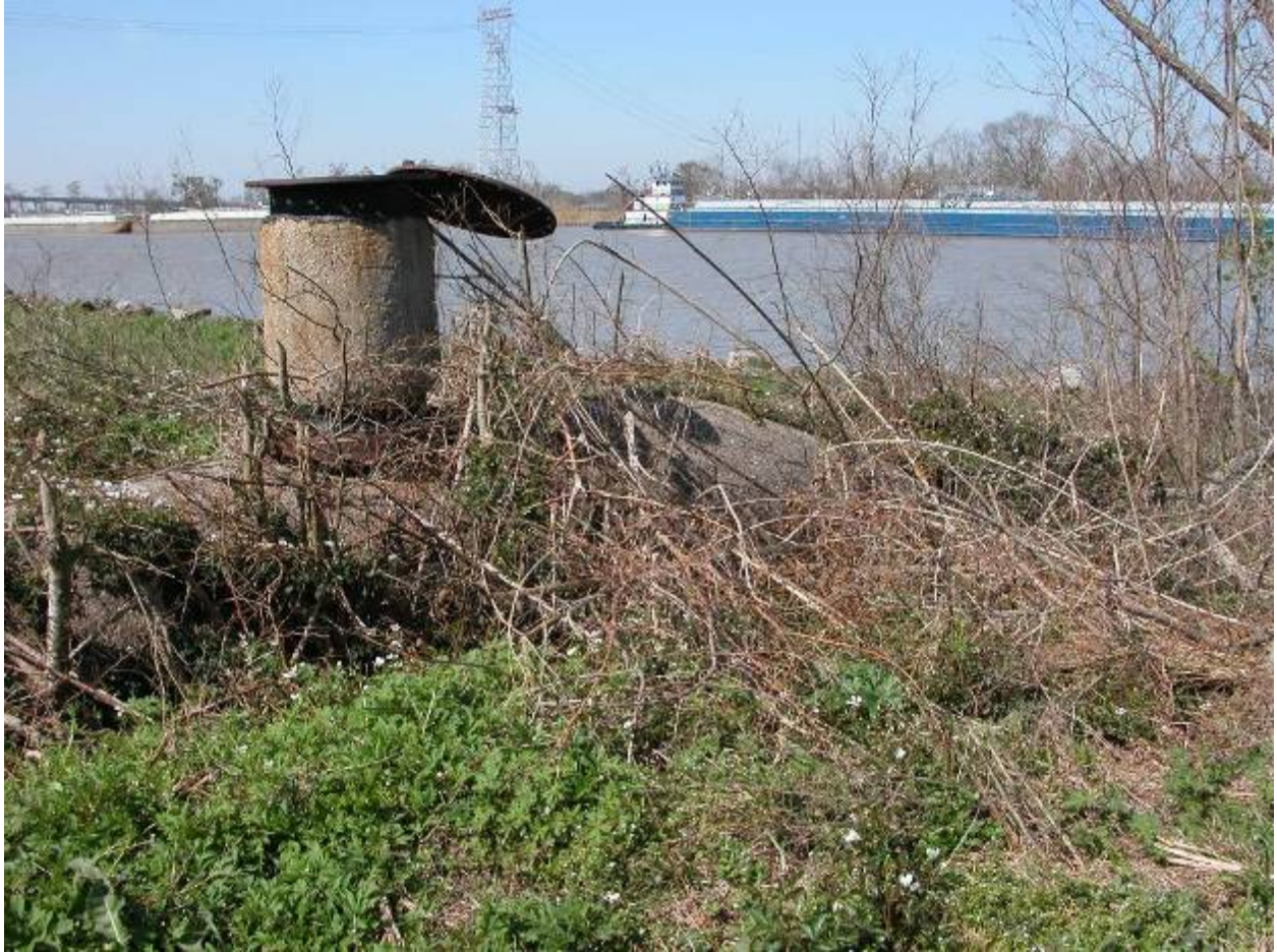
Abandoned pipe crossing through the Algiers Canal
