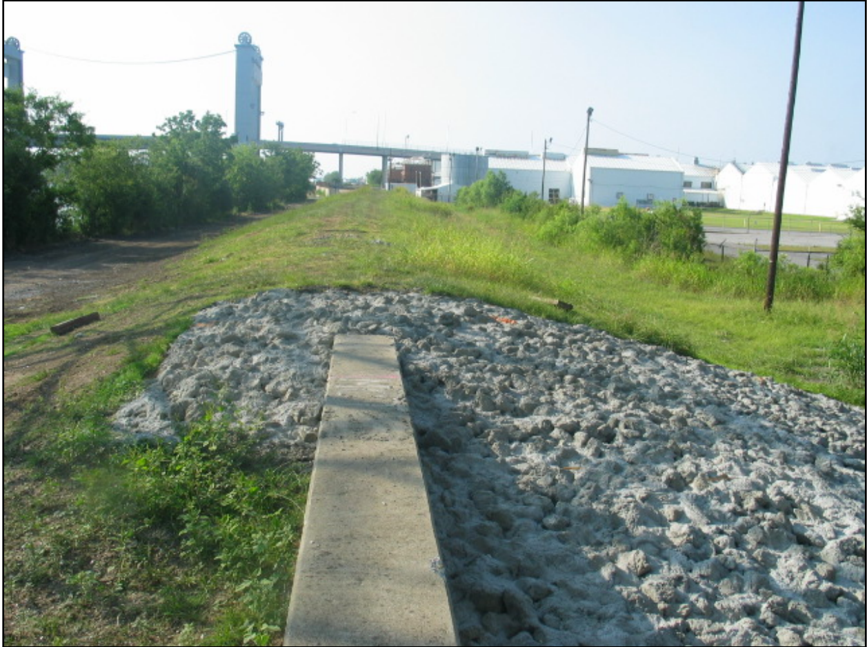
Figure NOE 37. Transition Improvements along IHNC Levee/FW Interfaces
