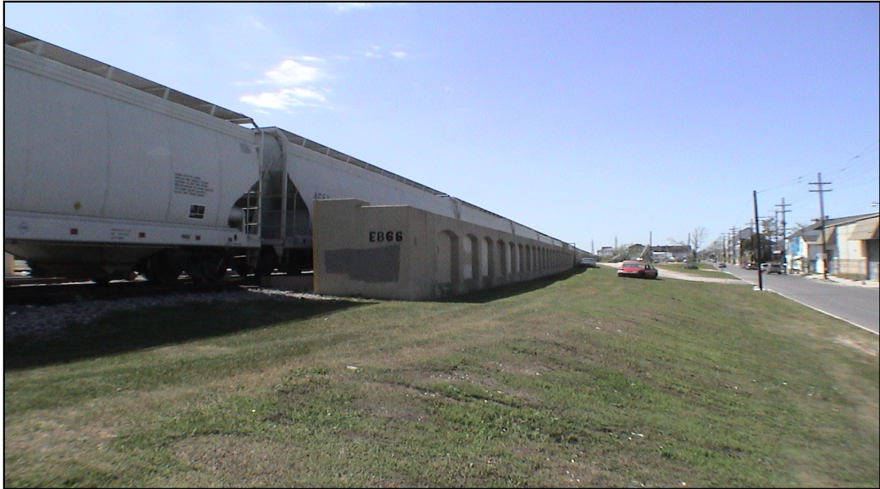
Typical Area on the Mississippi River East Levee and Floodwall.
