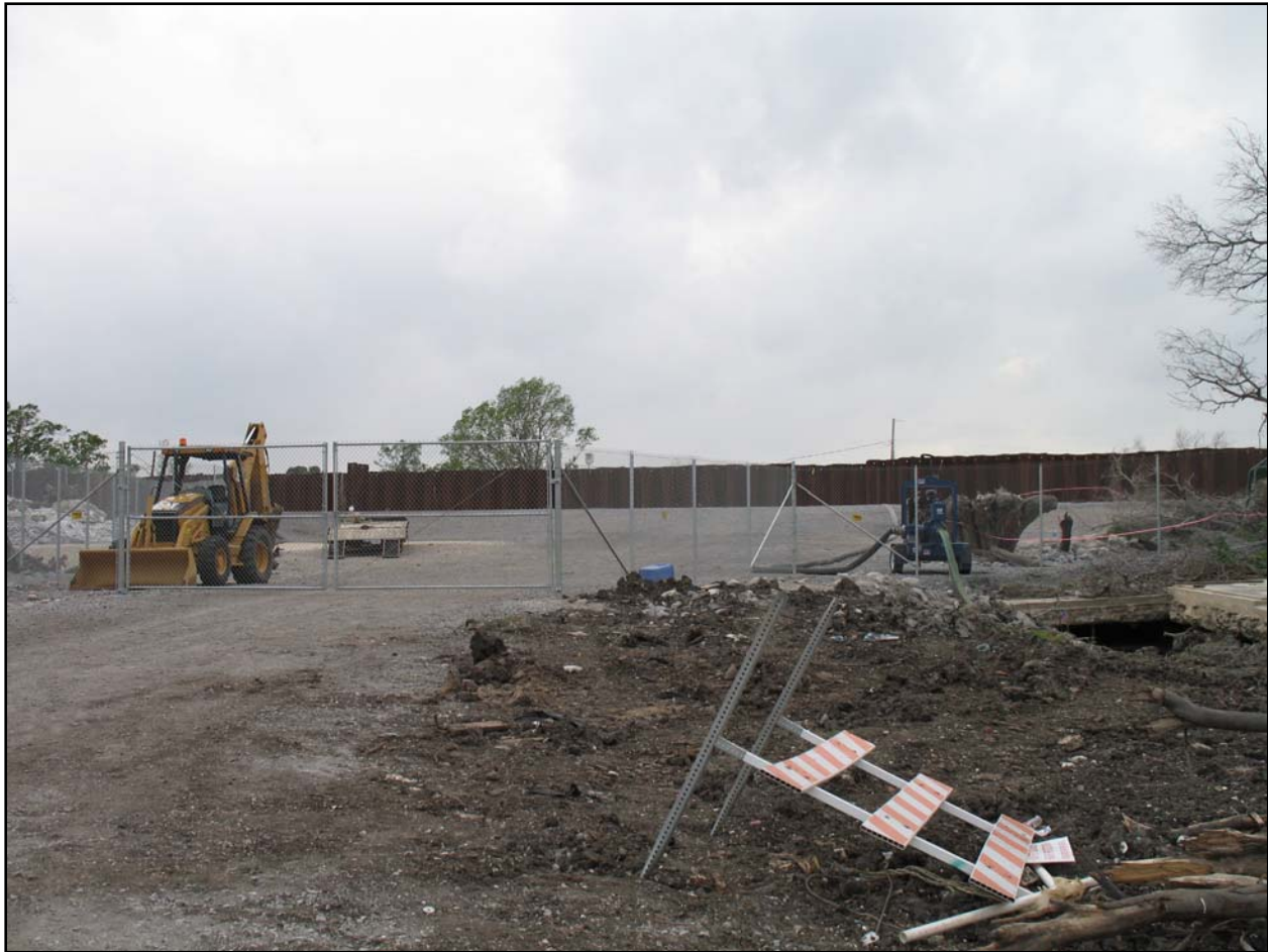
Figure 4. Sheetpile repair along the 17th Street Canal
