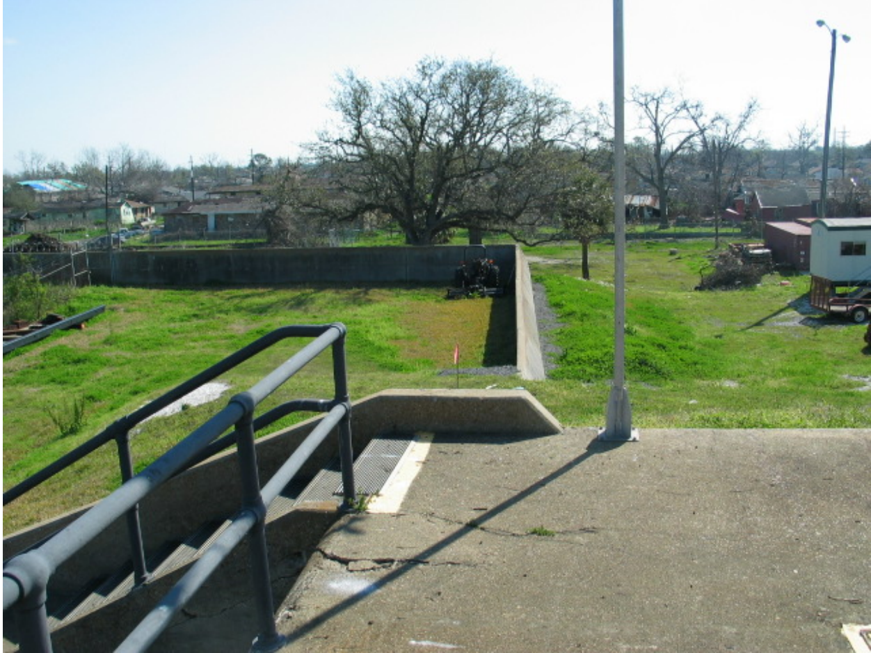
Figure STB 3. I-wall section tying into IHNC lock wall (standing on top of lock wall and looking away from IHNC)
