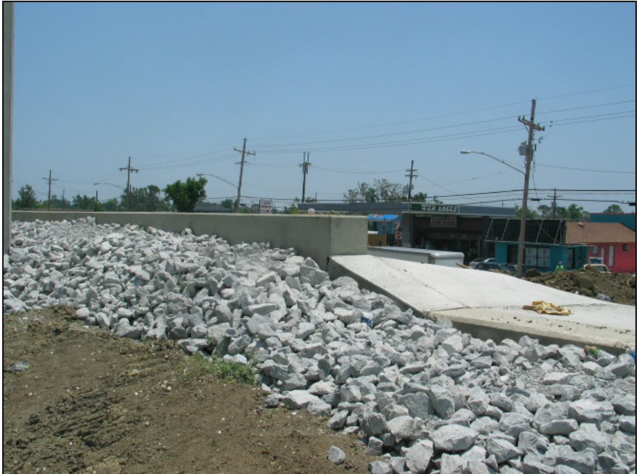
Figure NOE 24. Transition Improvements Between Reaches NOE 4&5 (Note: refer back to Figure NOE 6 taken from same location)
