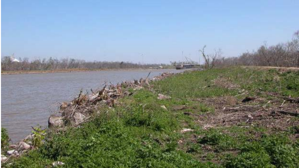
Typical Algiers Canal levee; no armor
