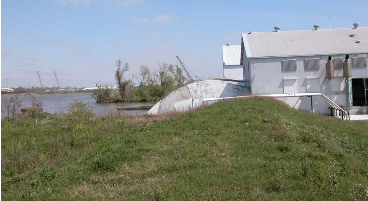
Plaquemines Pump Stations 1 and 2
