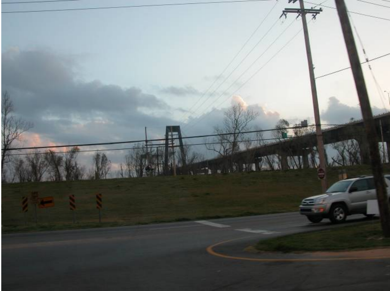
I-310 passing over the Mississippi River Levee
