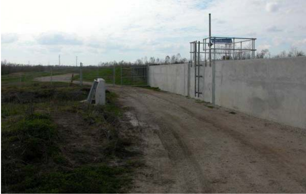
Alemedia Drainage Structure
