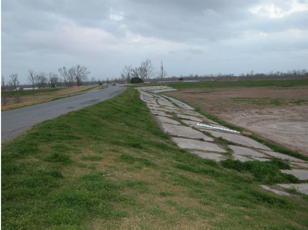
Mississippi River Levee intersection with Bonnet Carre Guide Levee
