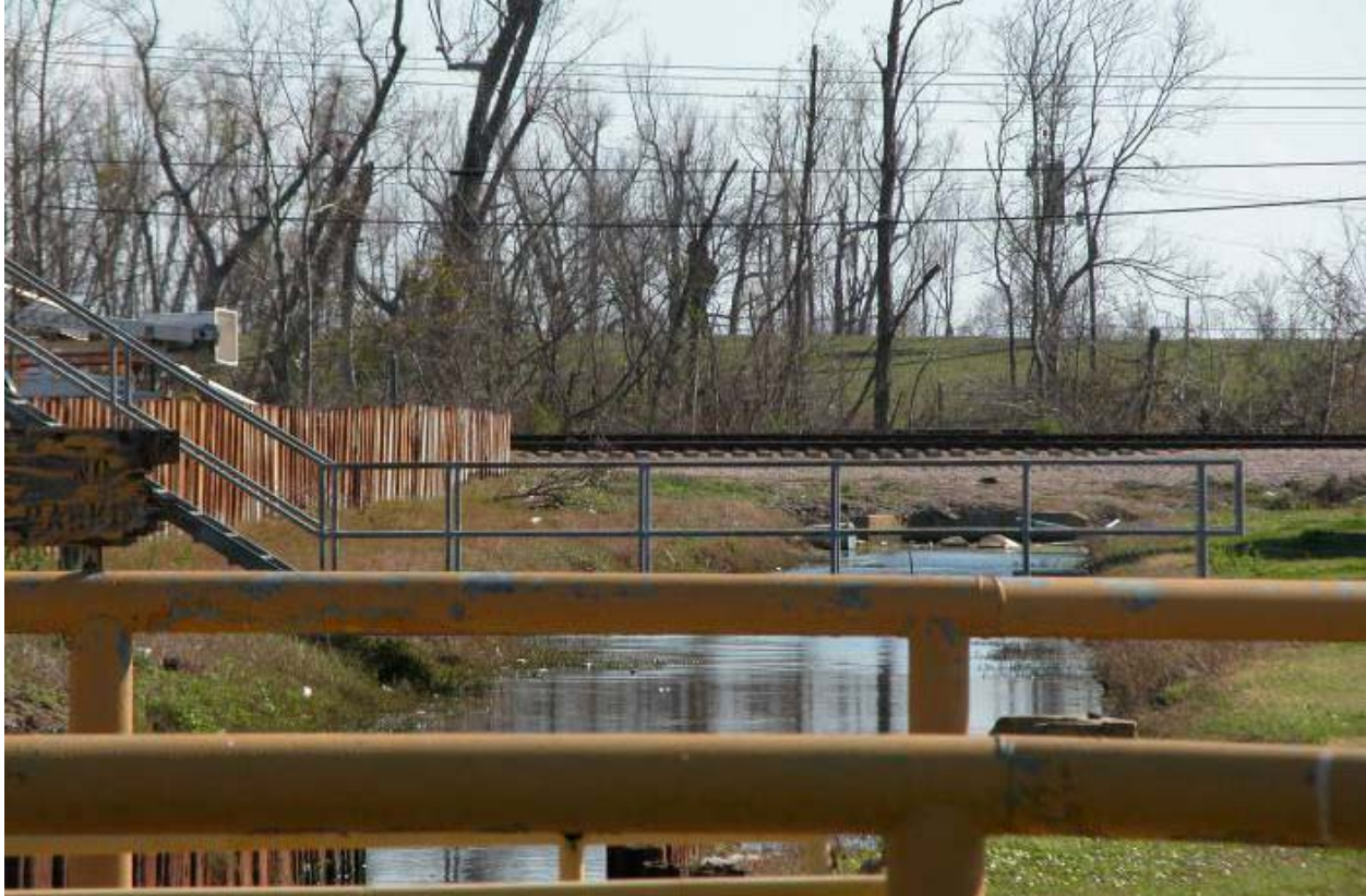
St. Charles –Jefferson Levee at South side of US 61
