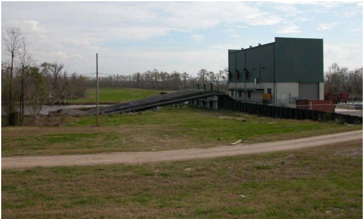
Trepagnier Pump Station
