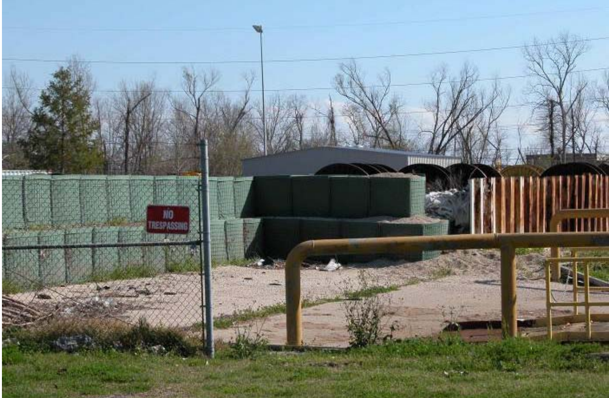
Short Transition Section of HPS from South of US 61 toward railroad
