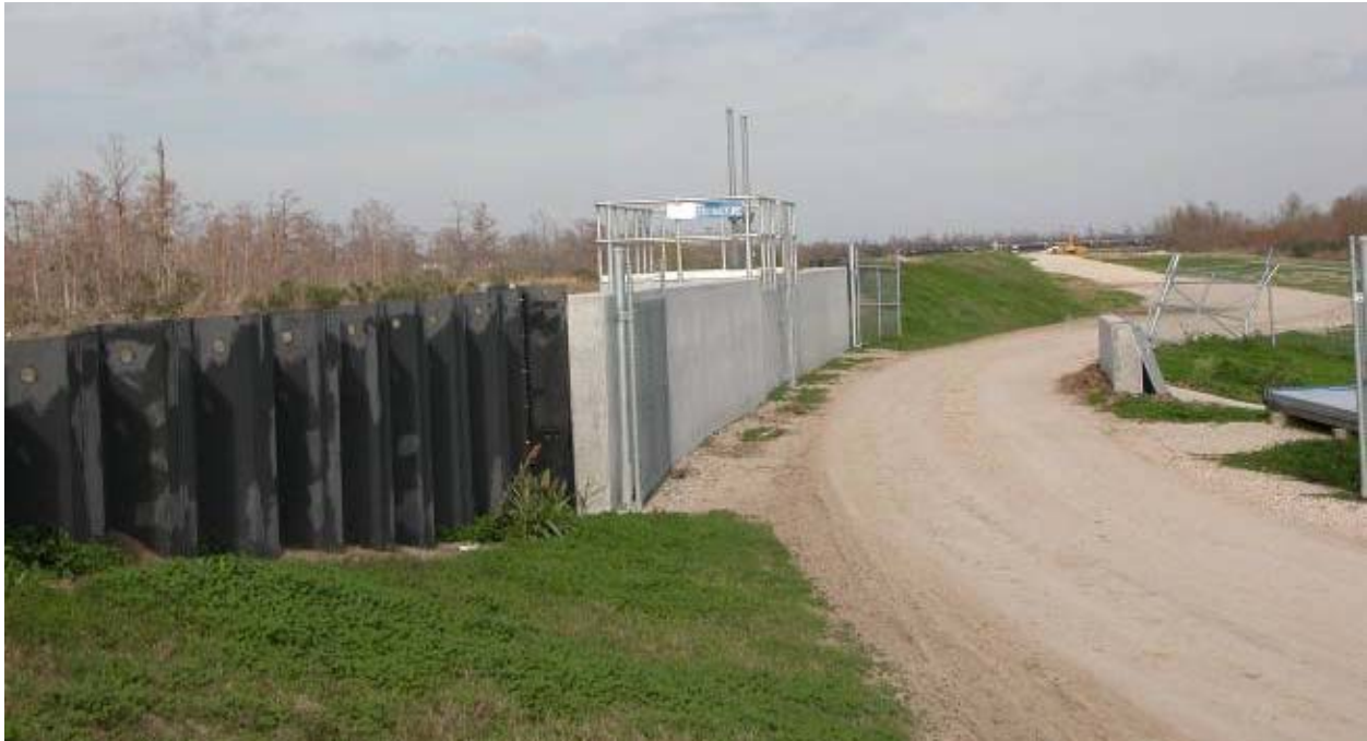
Walker Drainage Structure with sheetpile transition
