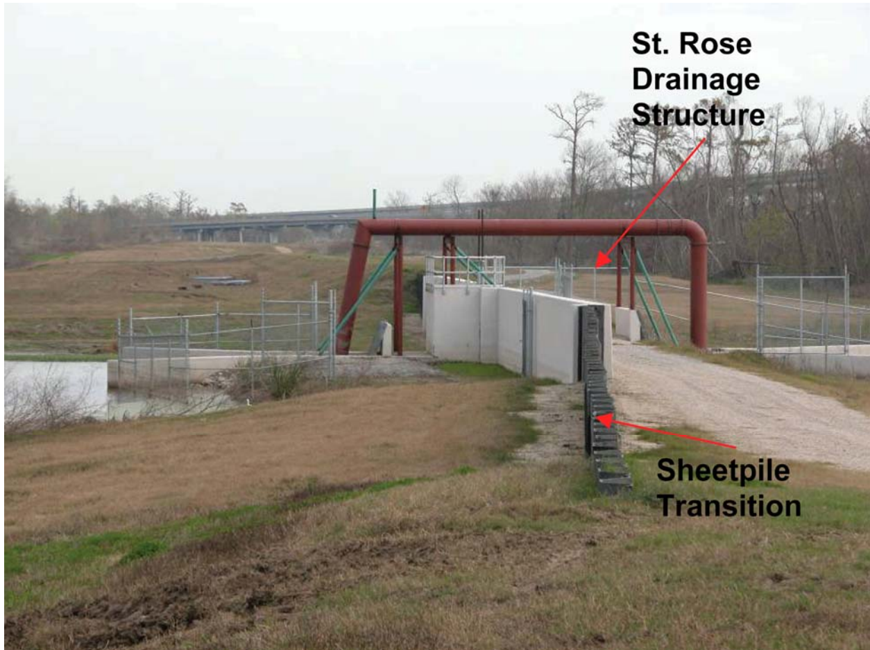
St. Rose Drainage Structure
