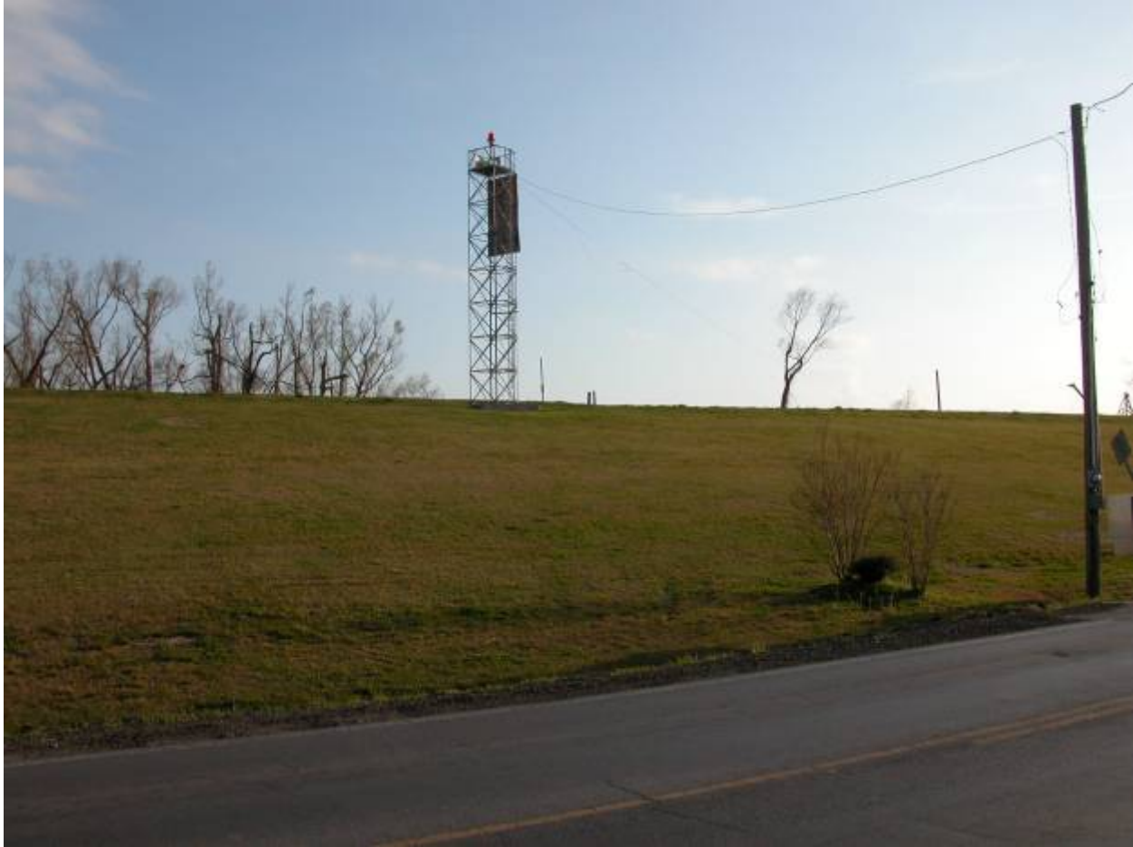
Mississippi River Levee at the St. Charles-Jefferson boundary at Hwy 48
