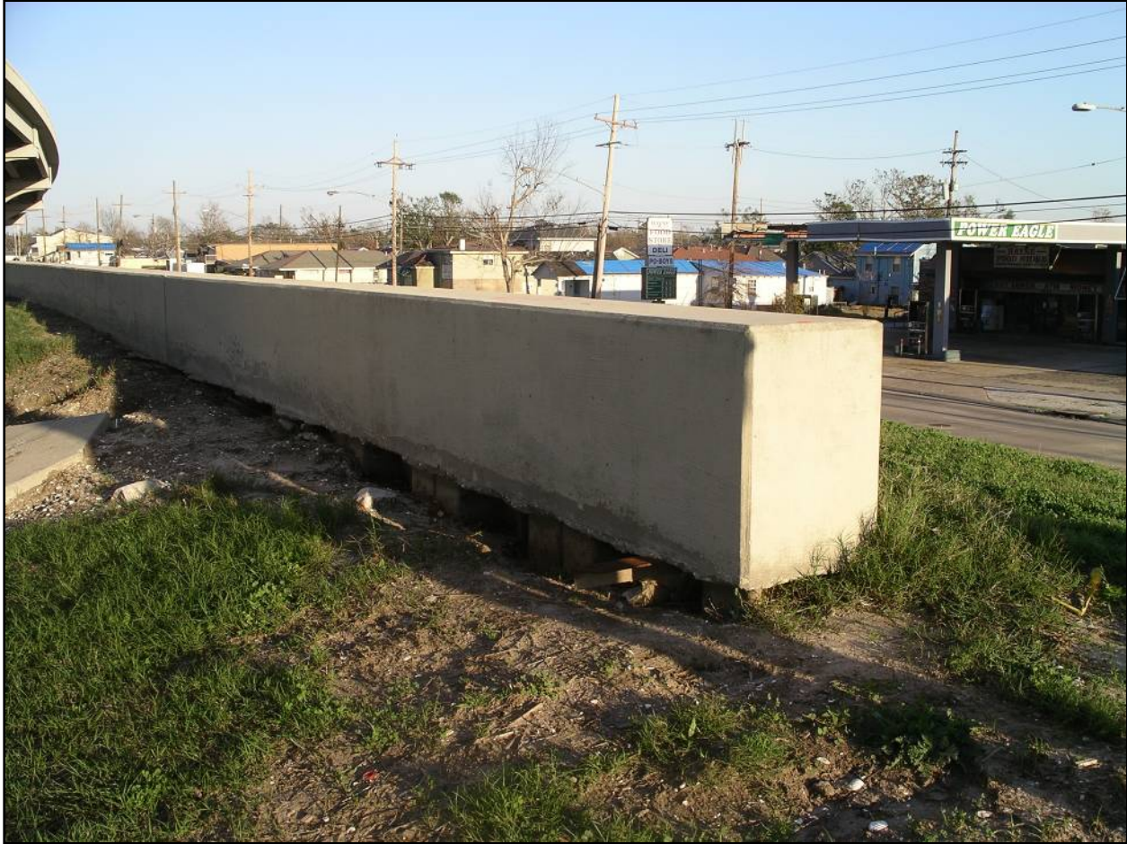
Figure NOE 6. Transition between Reaches NOE4 (Levee) and NOE5 (FW)
