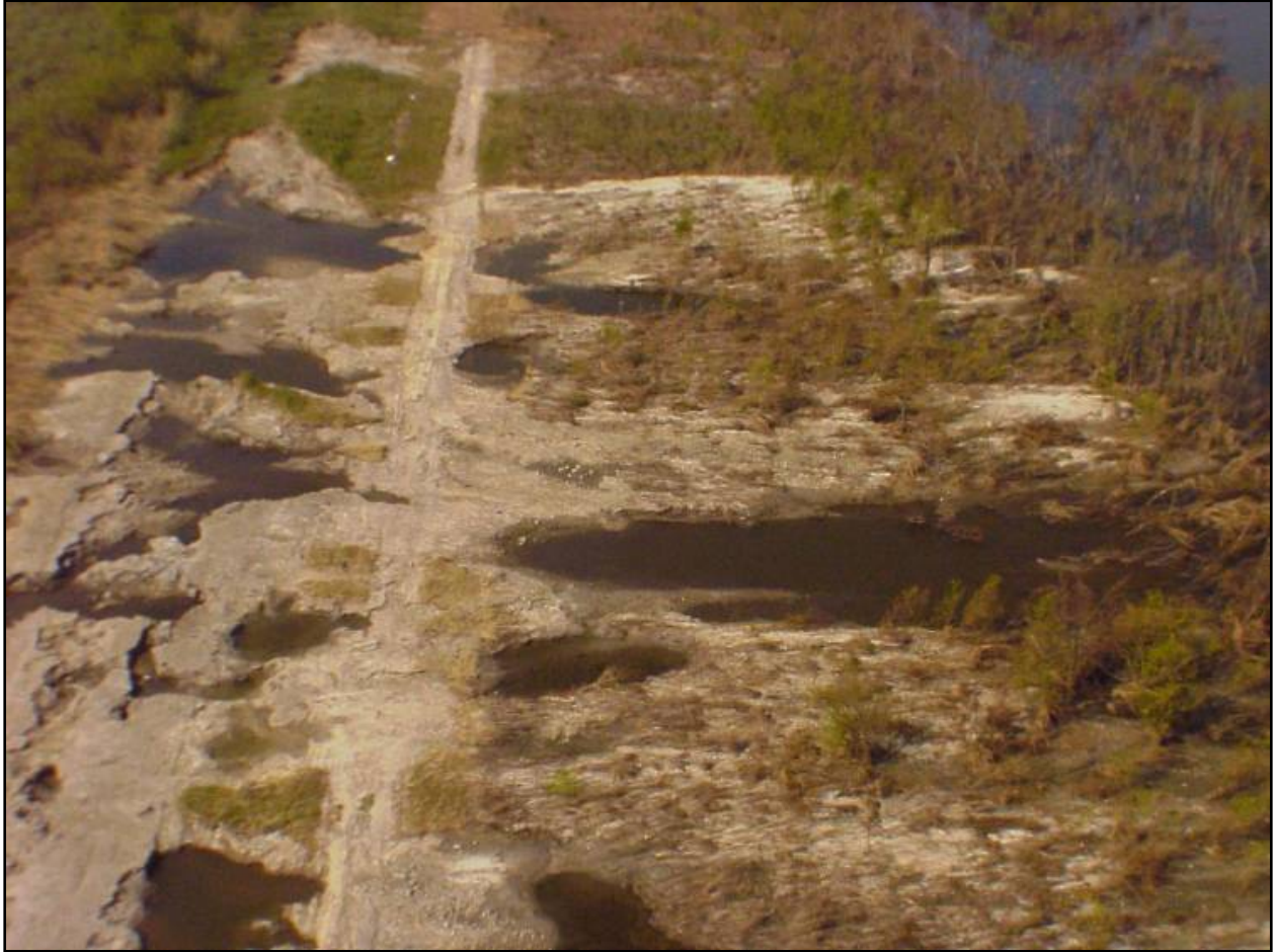
Figure NOE 11. Failure of Levee by Overtopping East of Pump Station #15 (East Back Levee)
