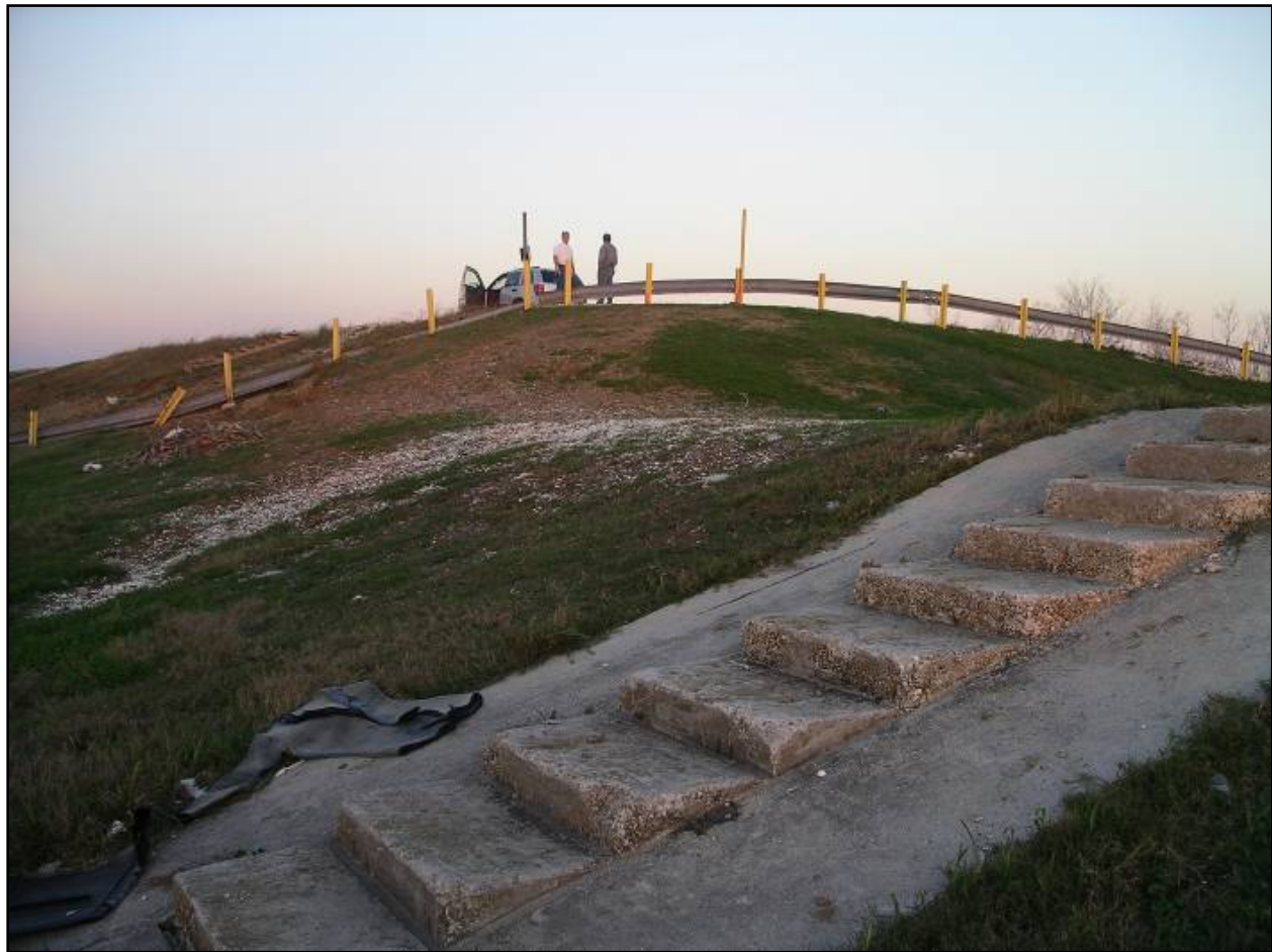
Figure NOE 9. Begin Lakefront Levee at Citrus Lakefront and Paris Road (Lakefront Levee @ El. 18.6± and Citrus Lakefront Levee @ 12.6±)
