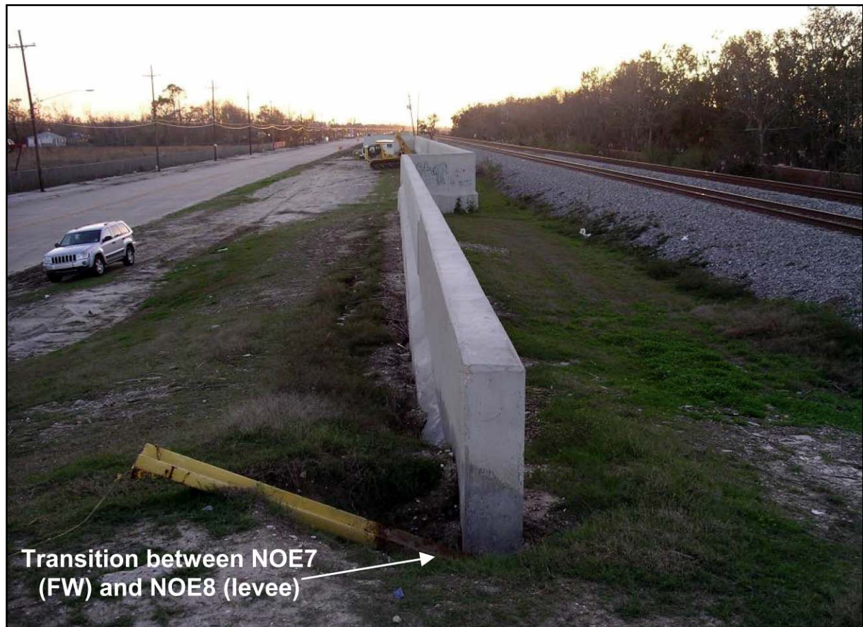
Figure NOE 8. Lincoln Beach Floodwall (Reach NOE7) (Looking west from Reach NOE8)
