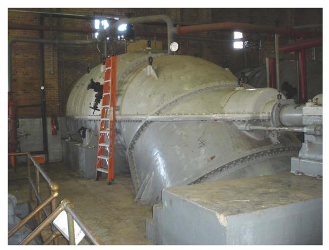
Figure 7. Large horizontal shaft pump.
