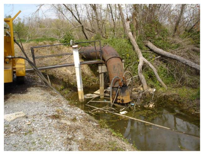
Figure 25. Hydraulically driven submersible pump.
