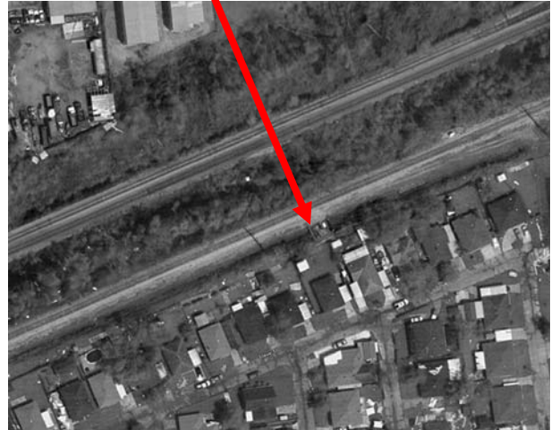
Arial view of the pump station
