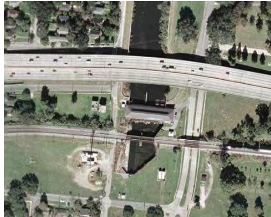
Before Hurricane Katrina: Aerial view of the pump station
