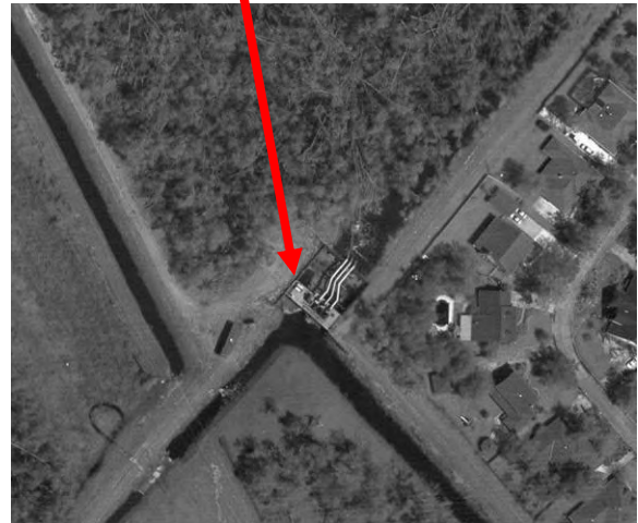
Arial view of the pump station
