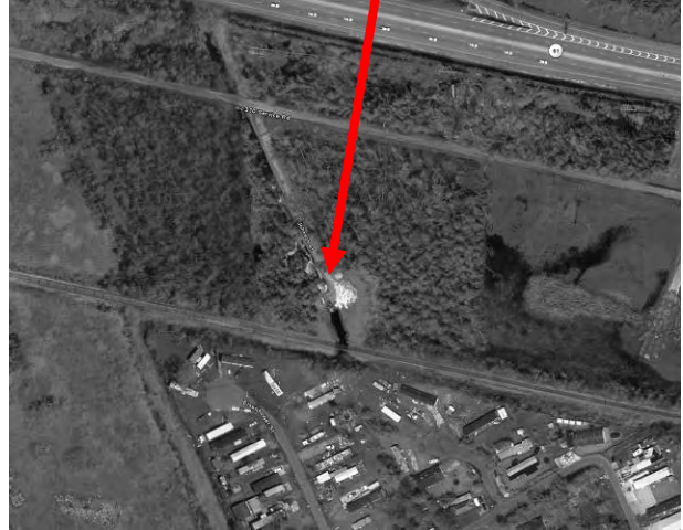
Arial view of the pump station
