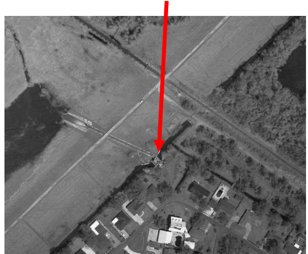
Arial view of the pump station
