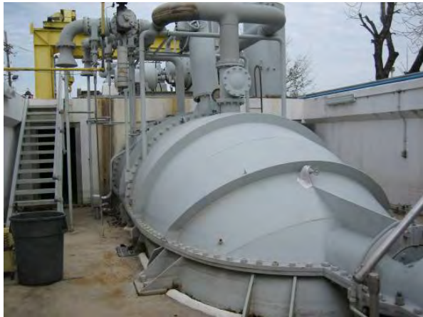
After Hurricane Katrina: View towards the discharge
