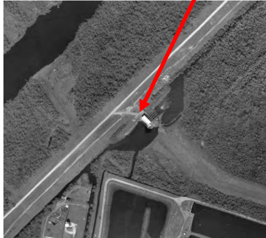
Arial view of the pump station
