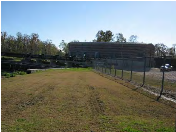
After Hurricane Katrina: View from the side
