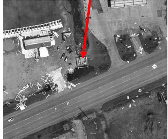
Arial view of the pump station
