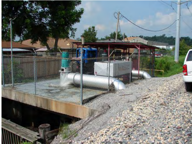
View of pump station from the ground
