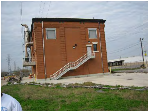
After Hurricane Katrina: View of the station
