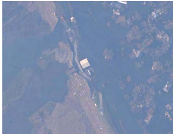
After Hurricane Katrina: Aerial view of the pump station
