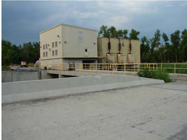
View of pump station from the ground
