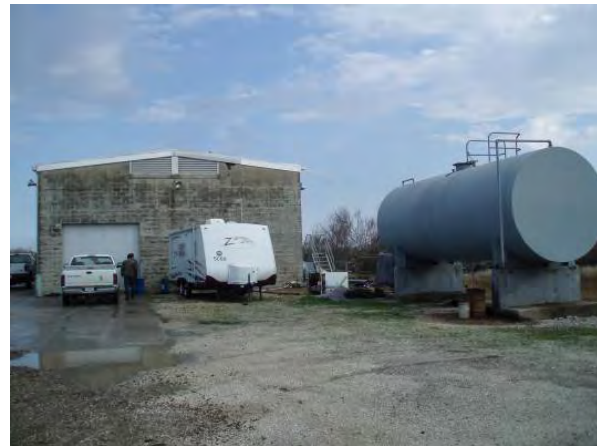
After Hurricane Katrina: View from the side
