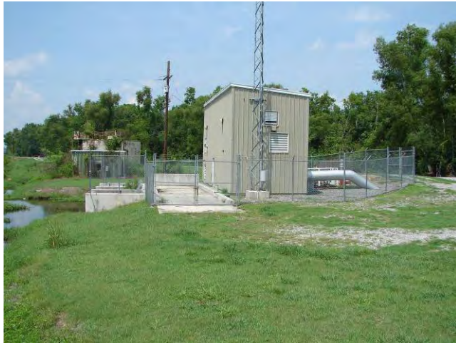
View of pump station from the ground
