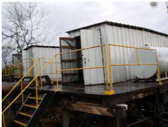
After Hurricane Katrina: View from the inlet canal
