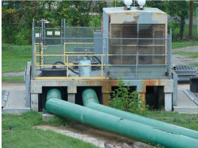
View of pump station from the ground
