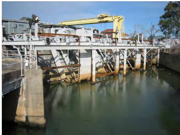
After Hurricane Katrina: View from the discharge
