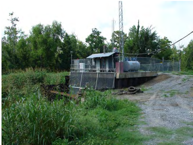
View of pump station from the ground
