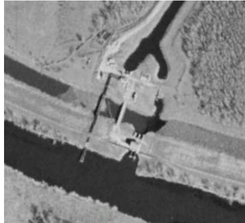
Before Hurricane Katrina: Aerial view of the pump station
