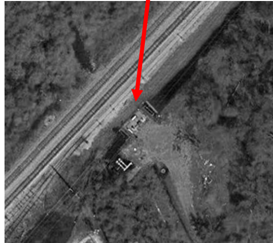
Arial view of the pump station
