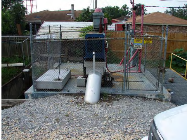
View of pump station from the ground
