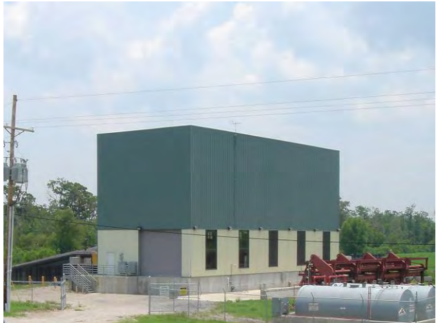
View of pump station from the ground
