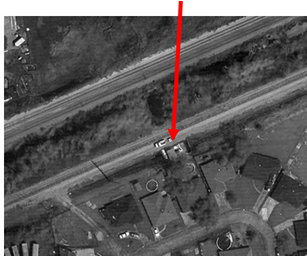
Arial view of the pump station
