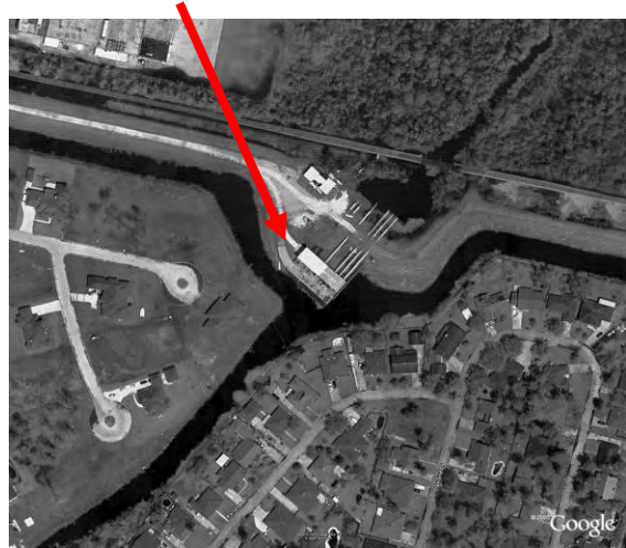
Arial view of the pump station
