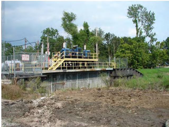
View of pump station from the ground
