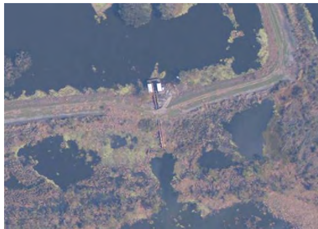
After Hurricane Katrina: Aerial view of the pump station
