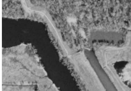
Before Hurricane Katrina: Aerial view of the pump station
