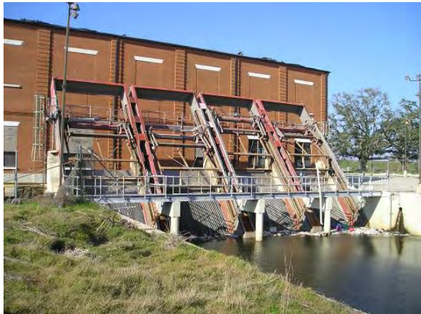
After Hurricane Katrina: View from the intake canal
