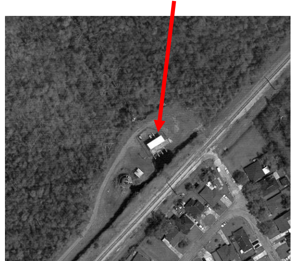
Arial view of the pump station
