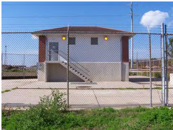
After Hurricane Katrina: View of the station
