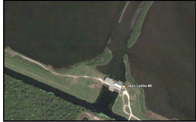
Before Hurricane Katrina: Aerial view of the pump station
