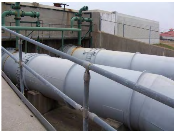
After Hurricane Katrina: View from the discharge side
