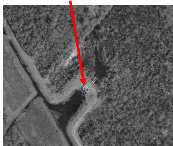
Arial view of the pump station
