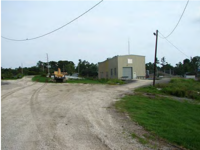
View of pump station from the ground
