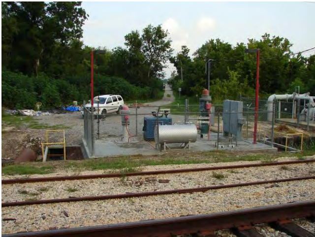
View of pump station from the ground
