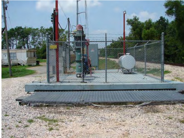
View of pump station from the ground
