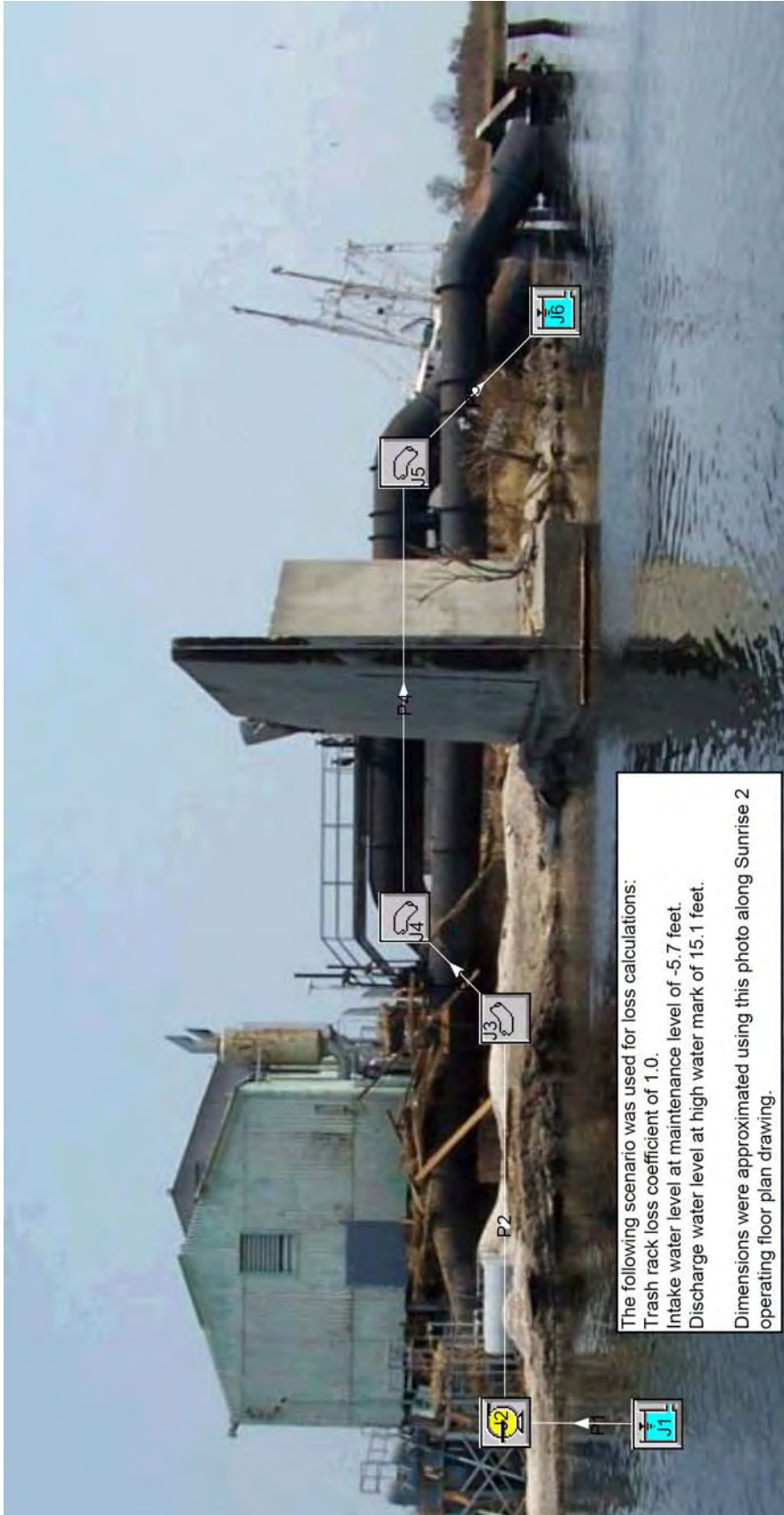
Figure 7-458 – Layout of 48 x 54” Patterson Pump at Sunrise 2
