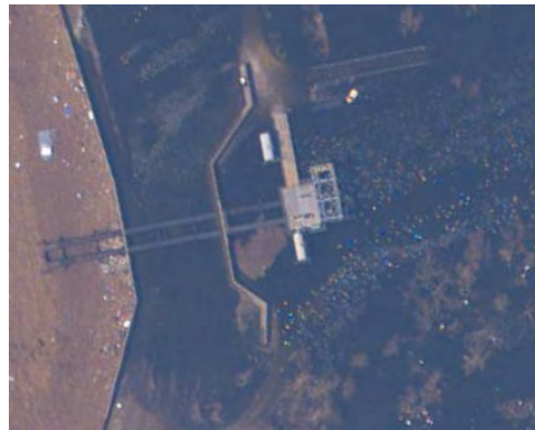
After Hurricane Katrina: Aerial view of the pump station
