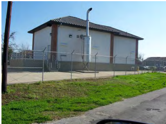
After Hurricane Katrina: View of the station
