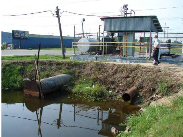
View of pump station from the ground
