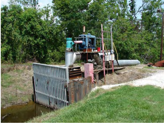
View of pump station from the ground
