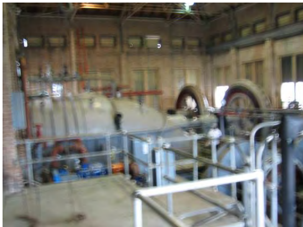
After Hurricane Katrina: View inside the station
