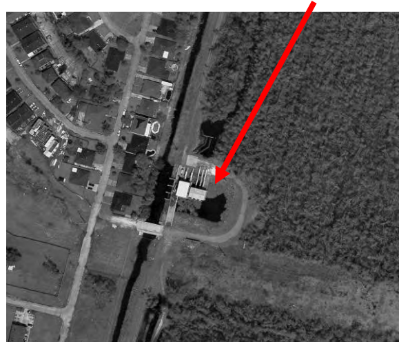
Arial view of the pump station
