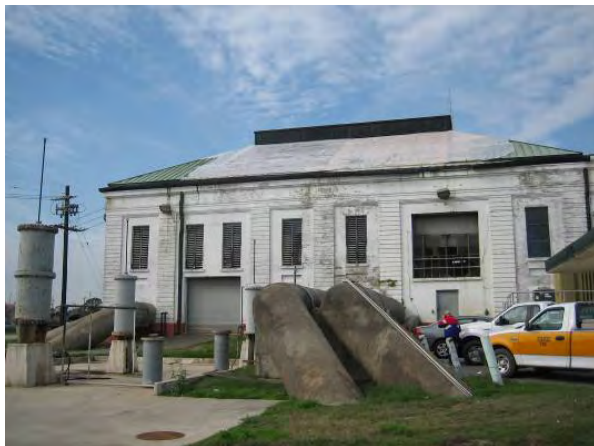
After Hurricane Katrina: View from the discharge
