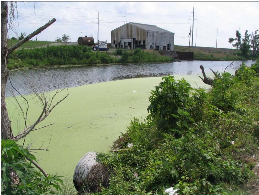
Photo 18. Forty Arpent Canal and at Pump Station No. 3, Bayou Villere.
