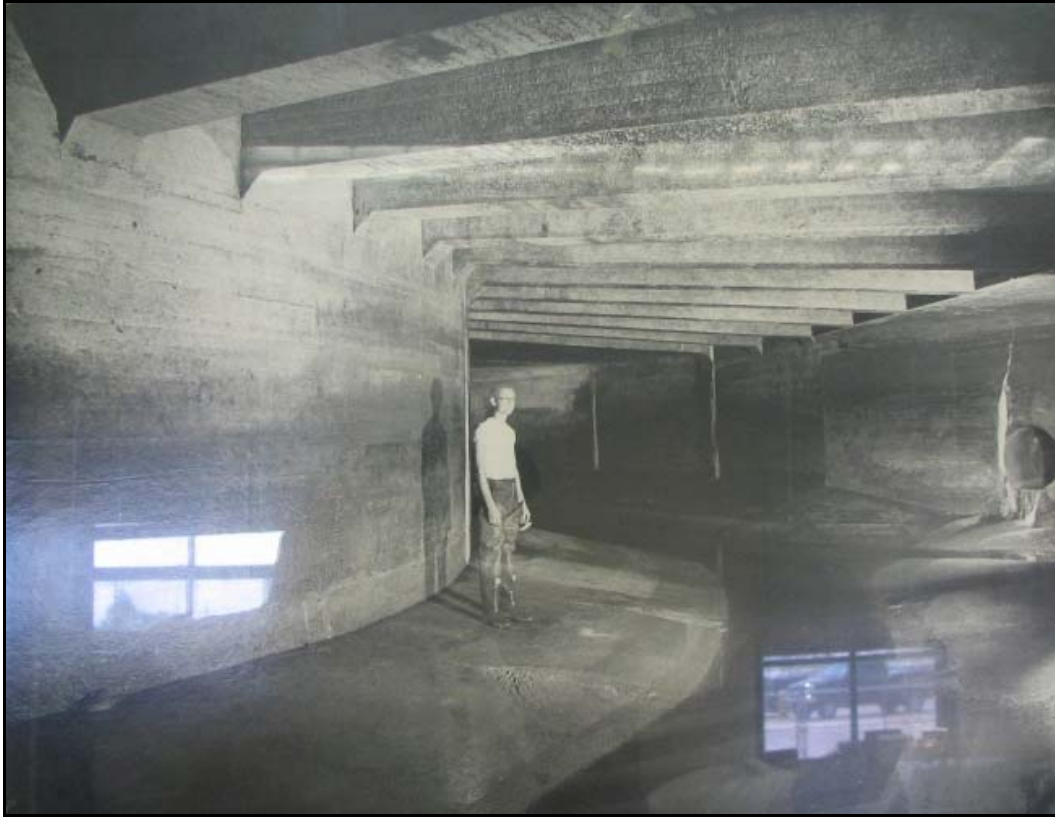
Photo 4. Claiborne Canal after construction.
