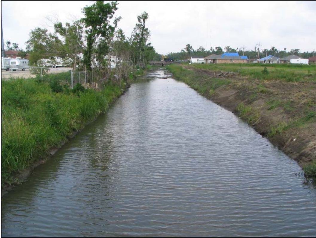
Photo 17. Interior Canal near Judge Perez Drive.
