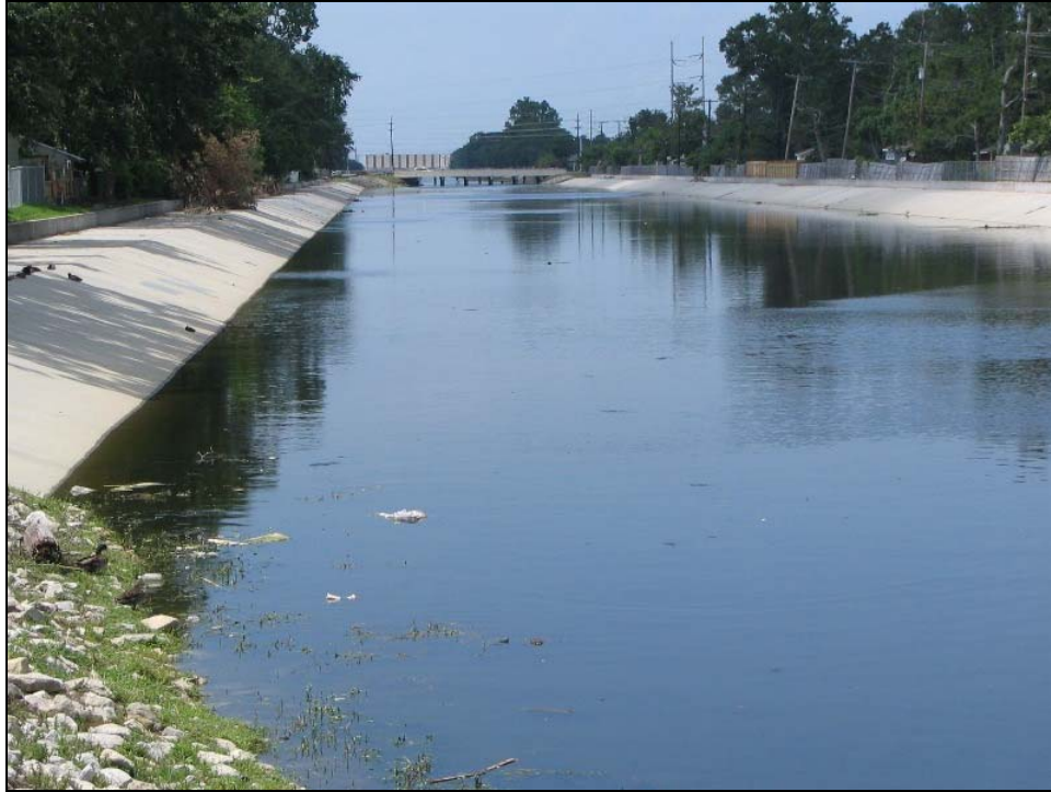
Photo 27. Elmwood Canal (interior) from Kawanee Avenue.
