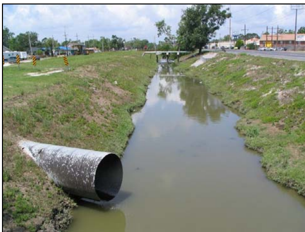
Photos 23 and 24. Storm sewer outfalls into canals.
