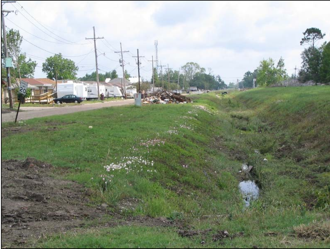
Photo 15. Typical roadside ditch collector.
