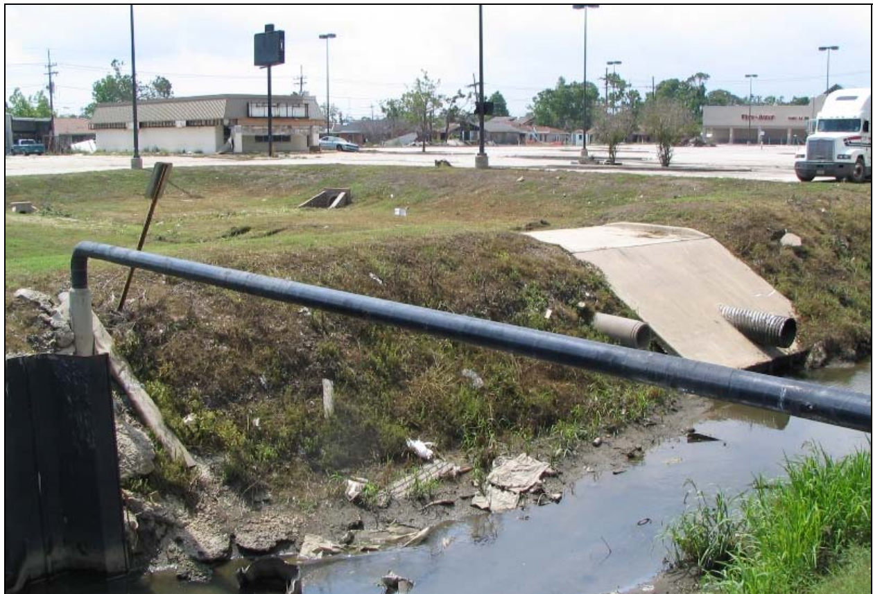
Photo 19. Onsite detention Basin on Judge Perez Drive.
