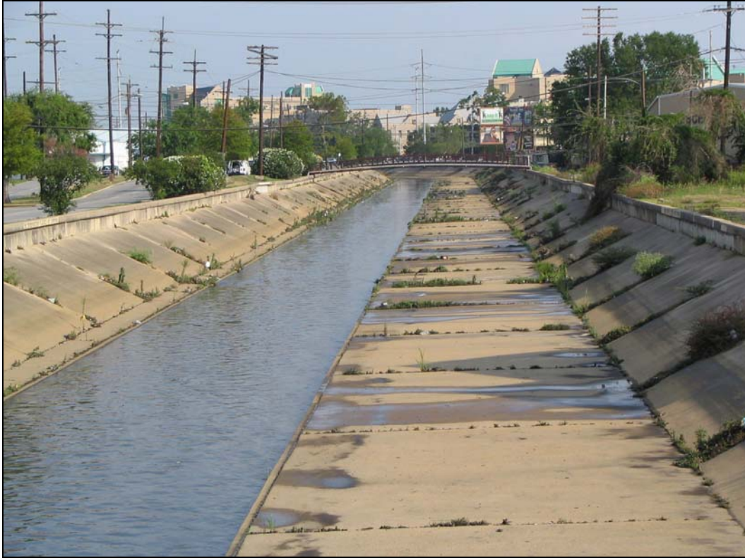
Photo 6. Palmetto Canal from Jefferson Davis Parkway.
