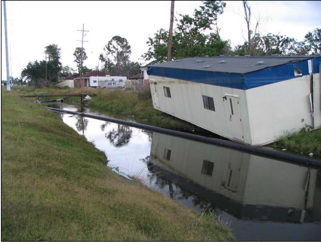
Photo 12. Dwyer Canal near Crowder Boulevard.
