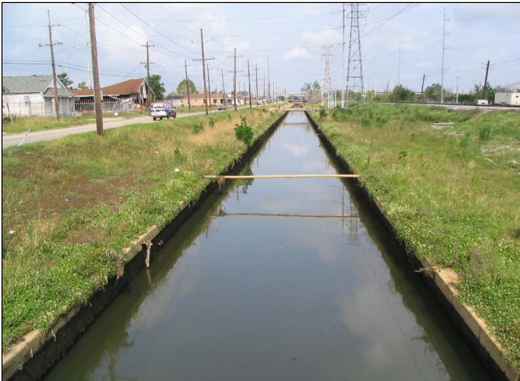
Photo 5. Florida Avenue Canal from Louisa Street.
