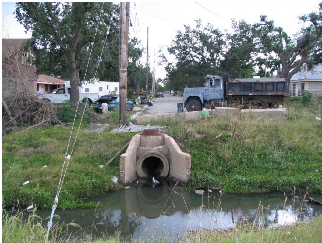
Photo 9. Storm sewer outfall into Dwyer Canal.
