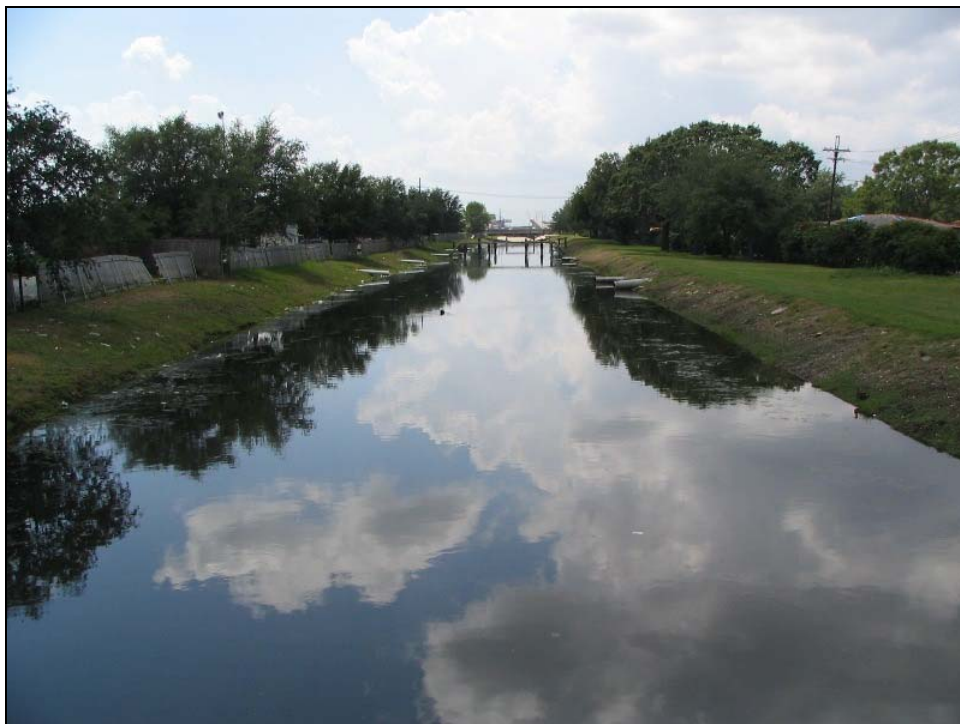
Photo 26. Interior Canal No. 3 from Bissonet Drive near Veterans Boulevard.
