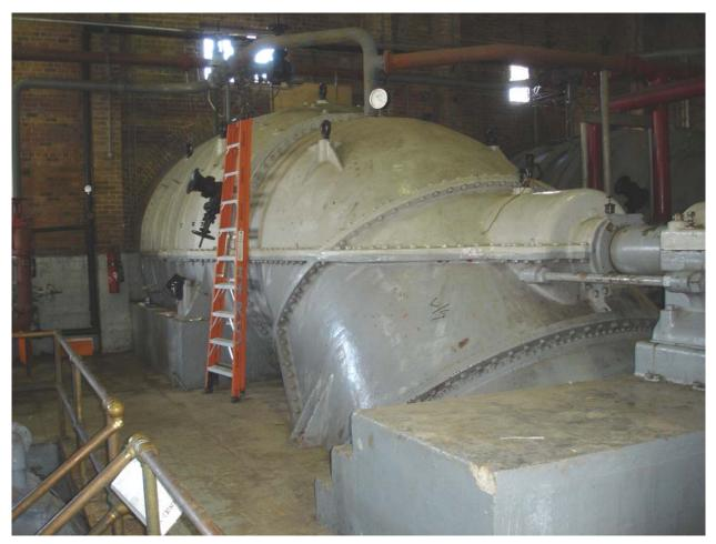
Figure 7. Large Horizontal Shaft Pump
