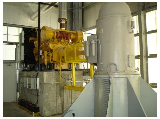
Figure 20. Vertical Diesel Driven Pump with Right-Angle Drive Speed Reducer
