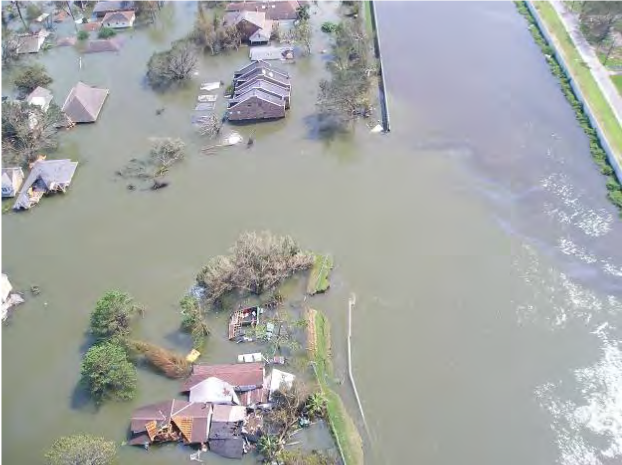
Figure 4. Aerial Photograph of the 17th Street Canal Breach Showing I-Wall and Embankment Translation
