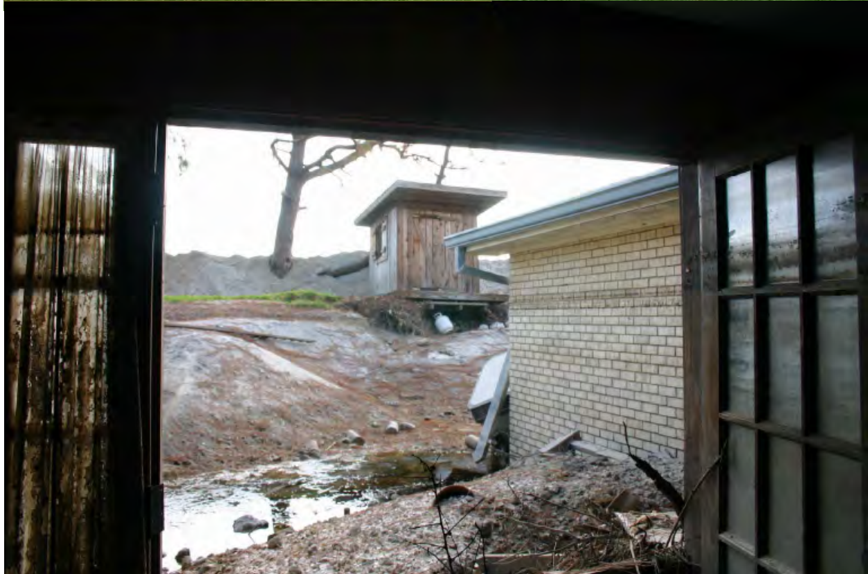
Figure 30. Playhouse at the London Avenue Canal North Breach Before the Failure (top photo) and After (bottom photo)
