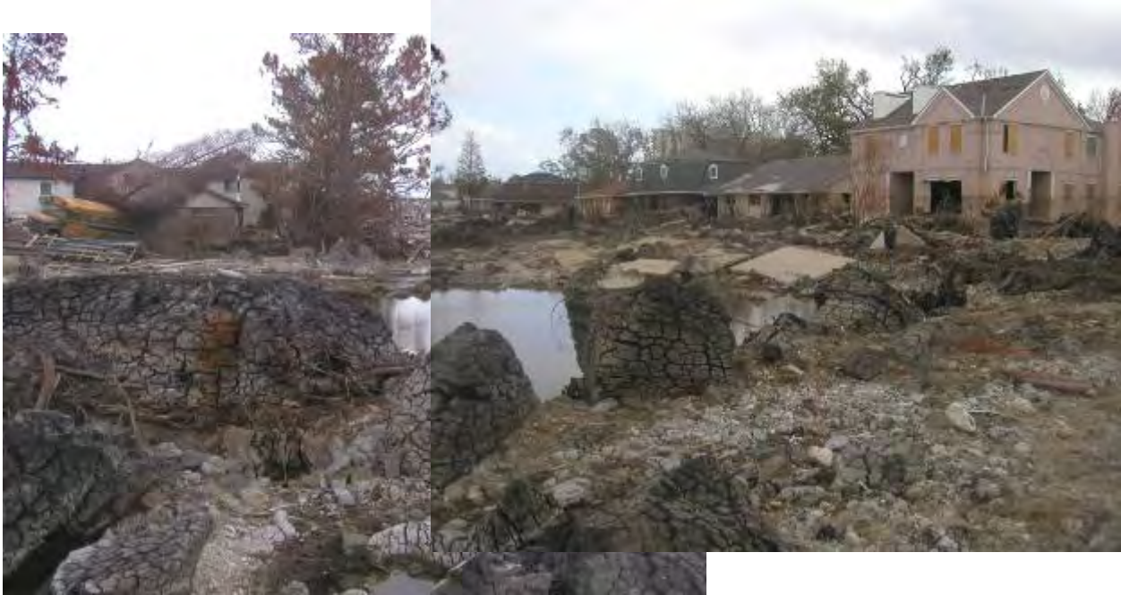
Figure 8. Marsh Blocks From the Levee Embankment at the 17th Street Canal Breach
