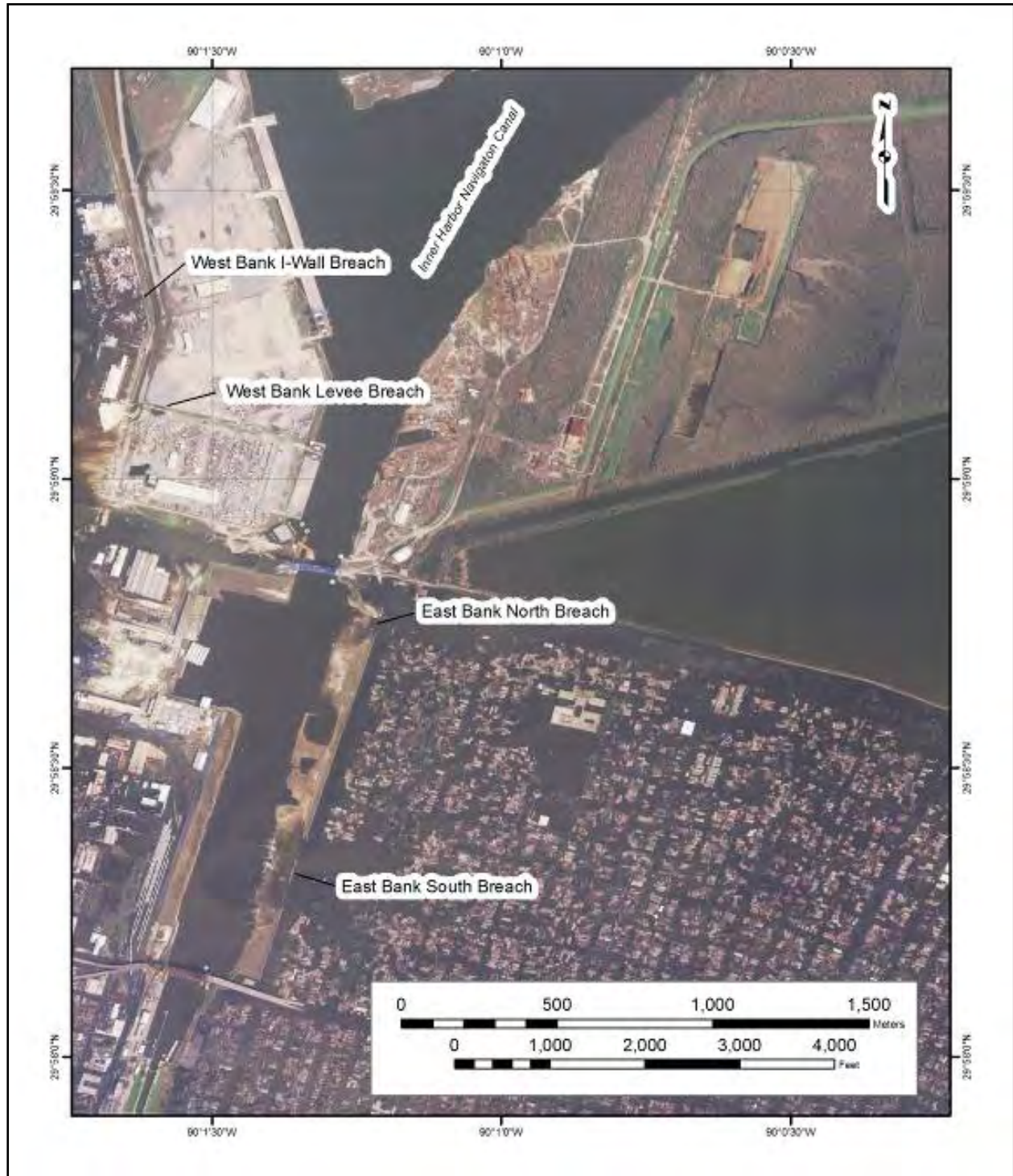
Figure 43. Four Breach Locations on the Inner Harbor Navigation Canal
