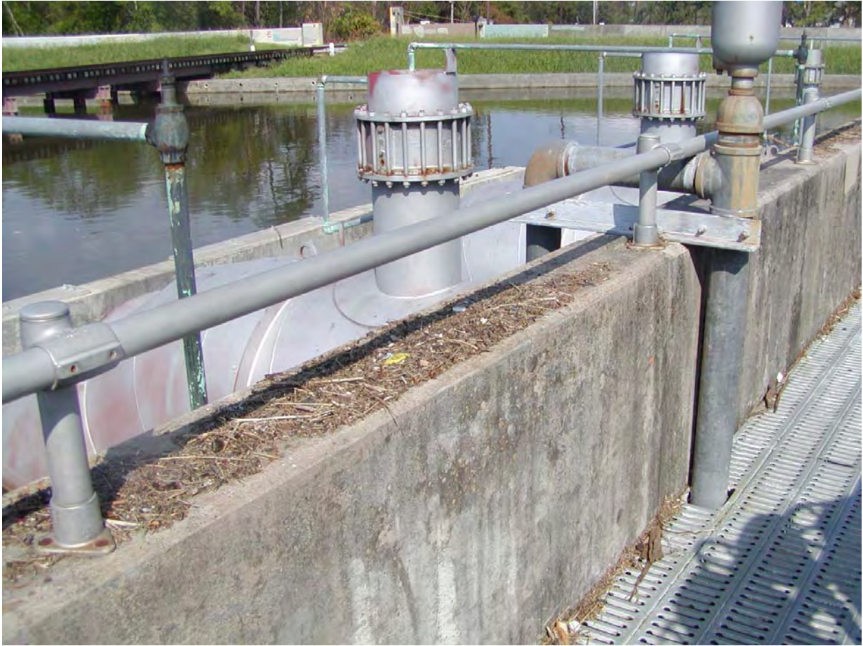
Figure 1-84. Debris on top of floodwall at OP#6 at 17th Street Canal.
