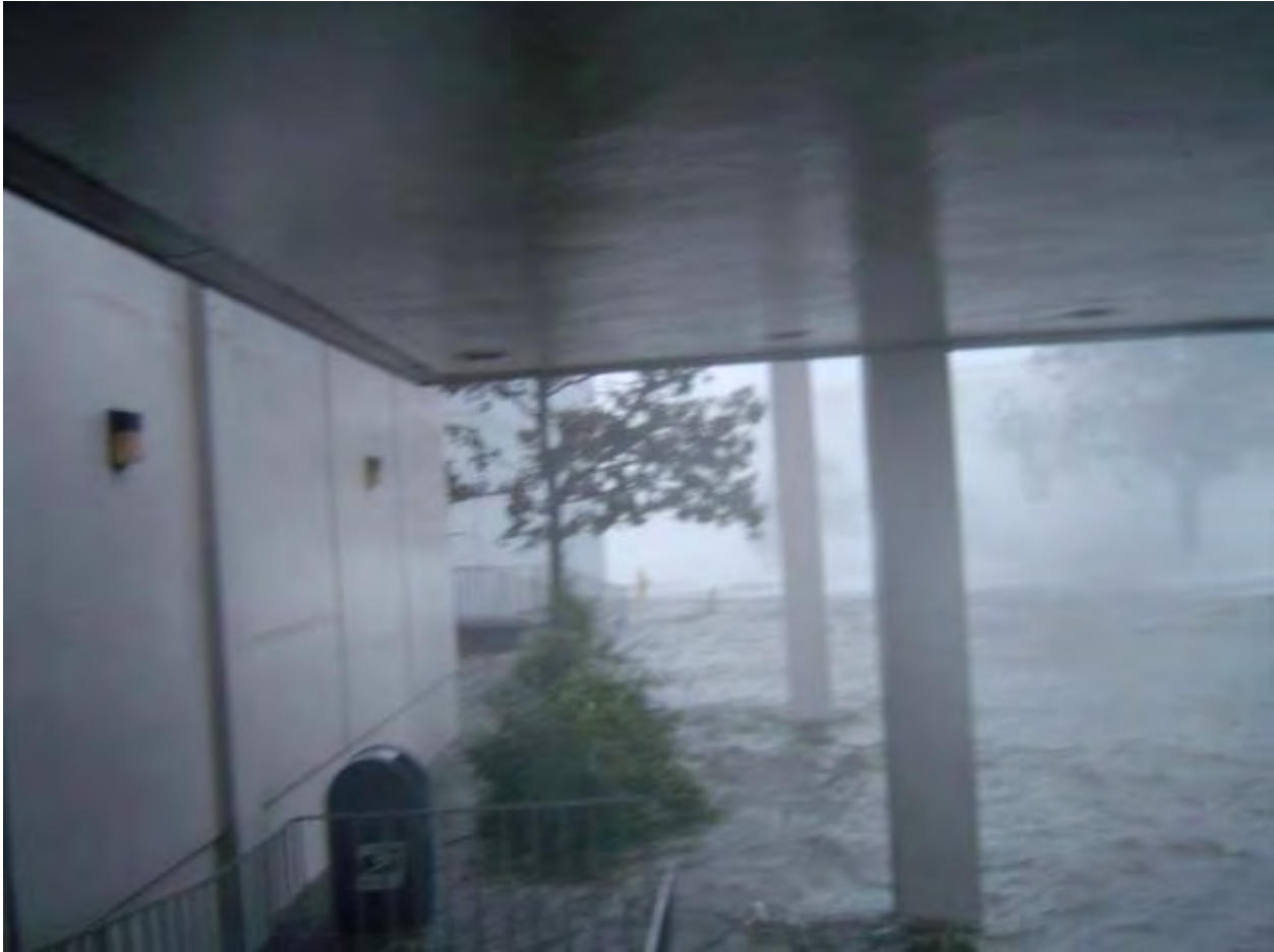
Figure 1-35. Time = 7:29, APH-22. Wall on south side of terminal building, east walkway
