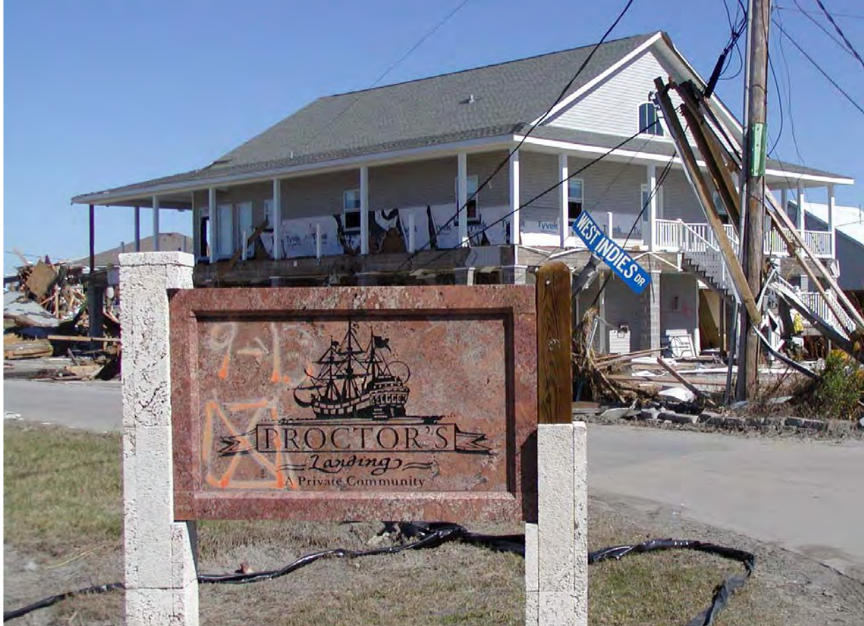
Figure 1-103. Home in Shell Beach containing high water mark LA 1087 at 31" above second level floor.
