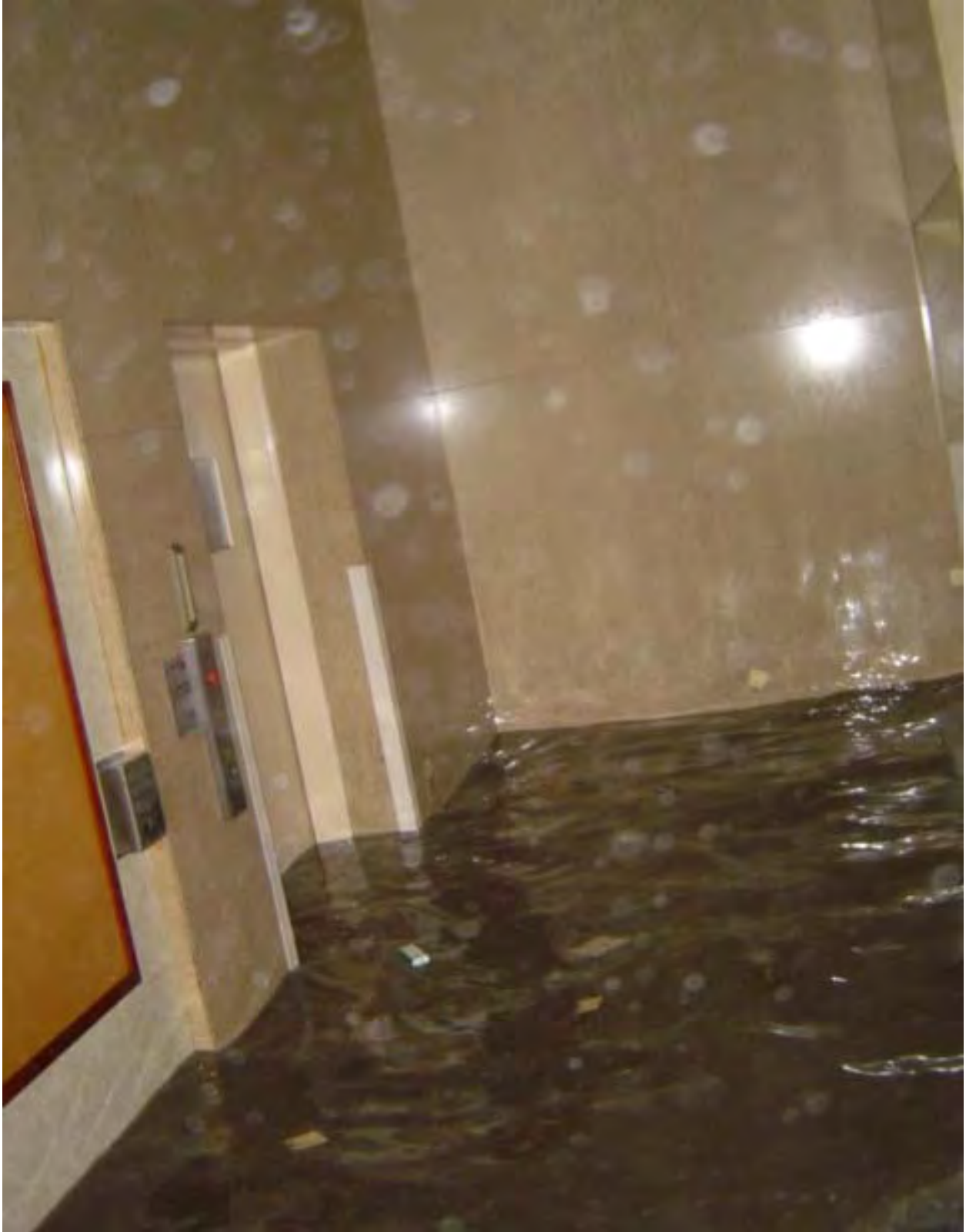
Figure 1-45. Time = 10:56 AM, APH-10, elevator east of lobby.
