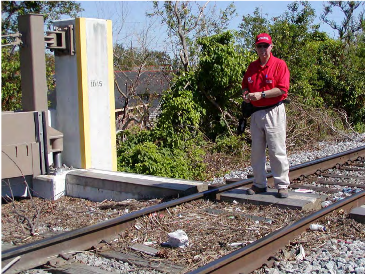
Figure 1-97. East floodgate at OP#3 at south end of London Avenue Canal. High water mark LA 1227 at top of railroad ties.
