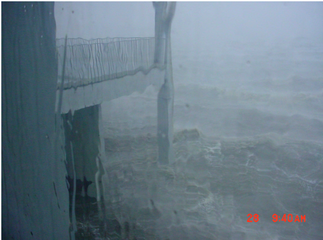
Figure 1-38. Time = 9:40 AM, APH-04. Water level on column northeast of lobby.
