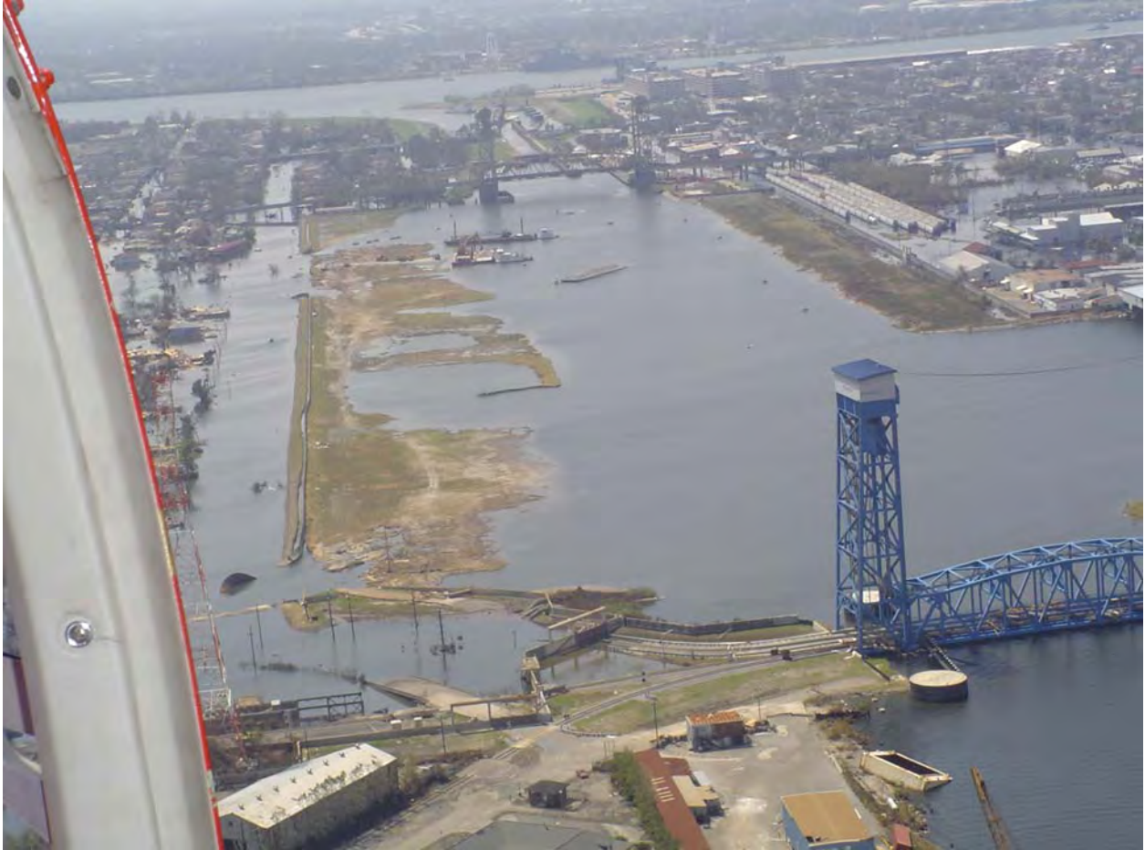
Figure 1-69. Florida Avenue railroad bridge (blue), two breaches on east side of IHNC into Lower 9 th Ward, and IHNC lock at top of picture. Picture looking south-southwest. Note debris on railroad bridge.
