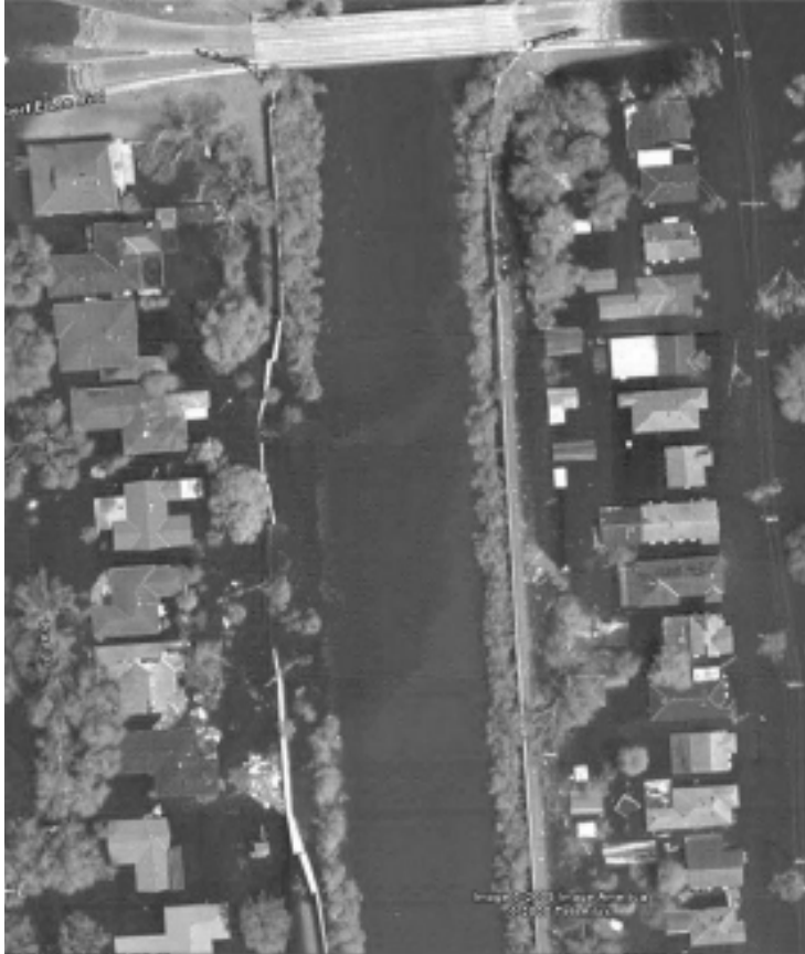
(a) North breach near Robert E. Lee Bridge Figure 11-1. London Avenue Canal breaches
