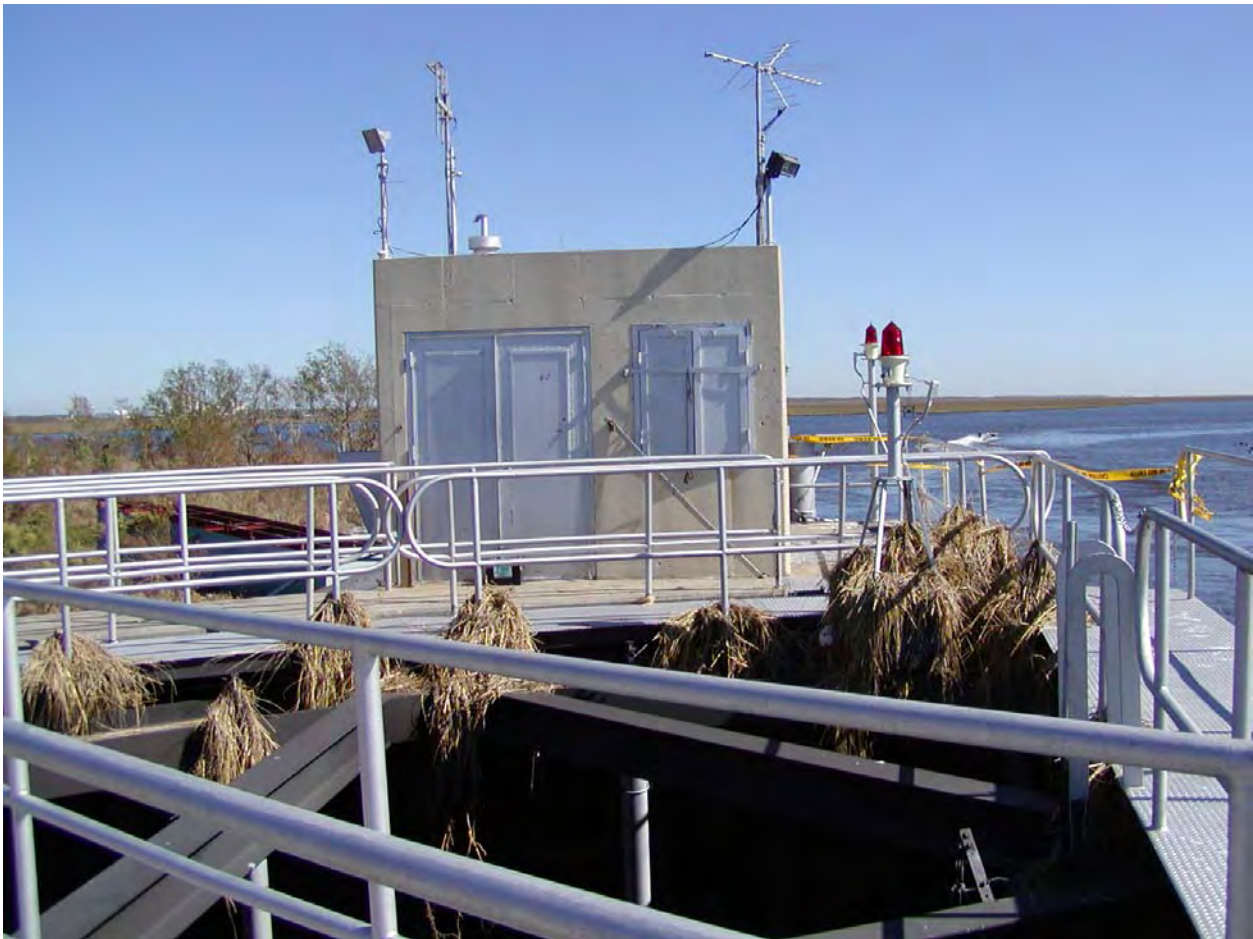
Figure 1-101. Bayou Bienvenue Gage House.
