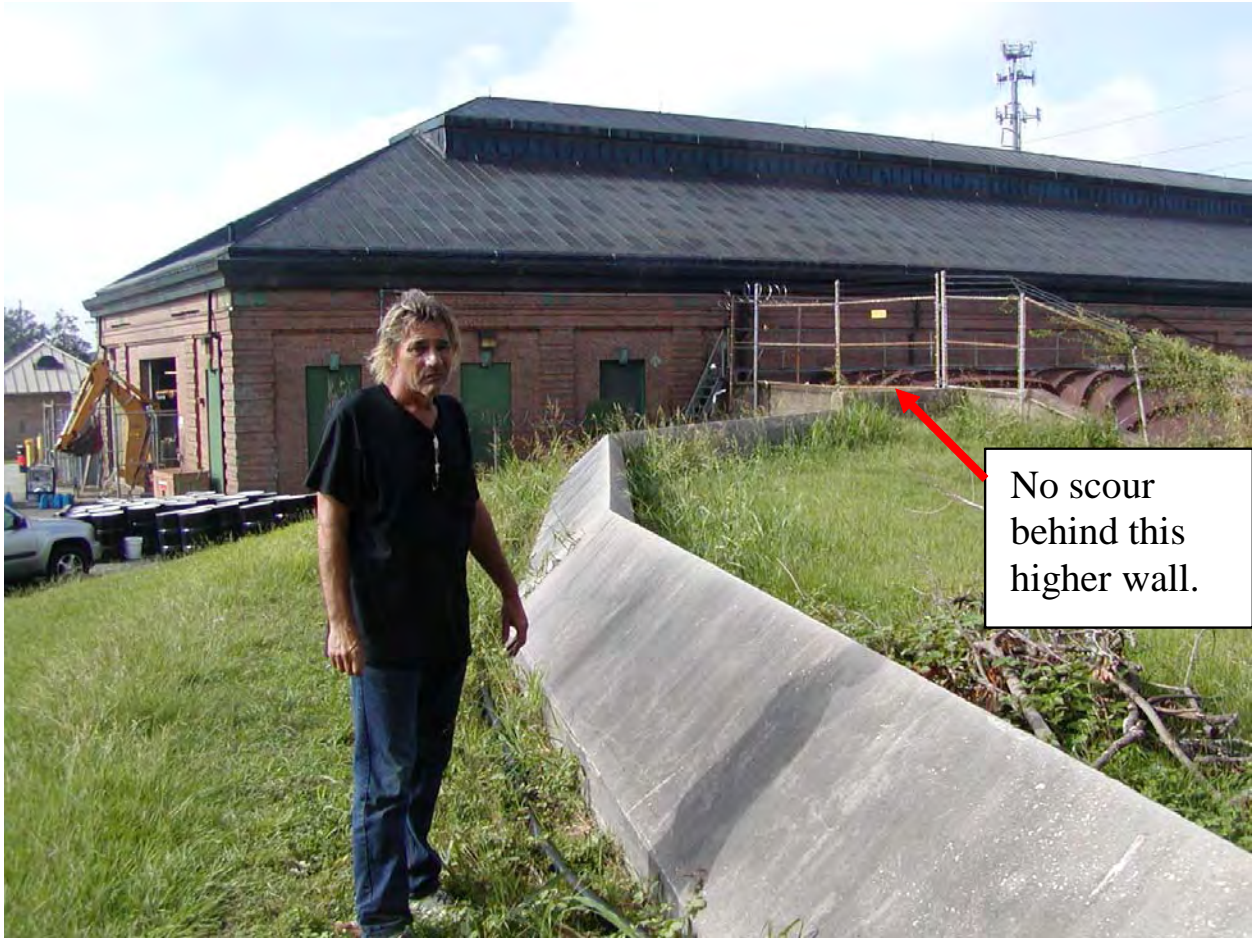
Figure 1-71. Low pump station wall at Orleans Avenue Pump station OP#7.
