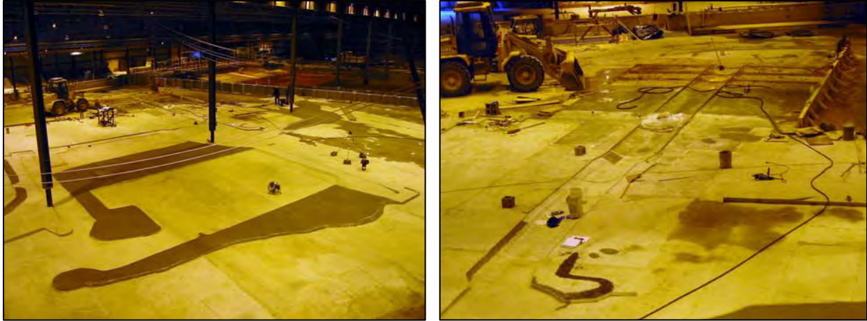
Figure 12-3. Physical model during construction; left photo showing overall view, and right view looking southward down the 17th Street Canal
