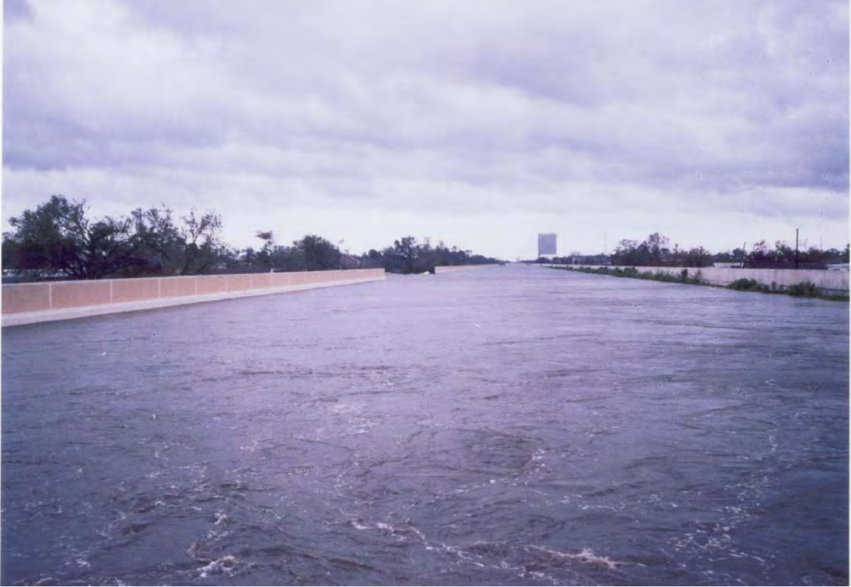
Figure 1-88. 17th Street Canal and breach at 2 pm on 8/29/05. Looking south.
