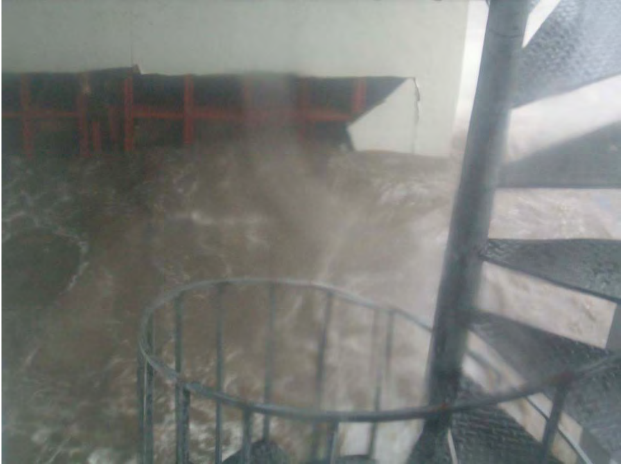
Figure 1-41. Time = 9:56 AM, APH-16. Wall north of east spiral staircase.
