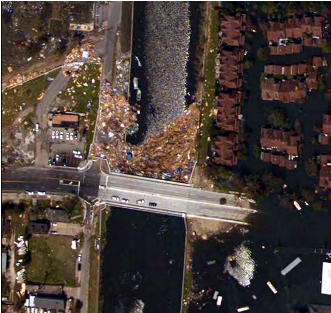
Figure 12-19. Post-storm debris at Hammond Highway Bridge. The triangular wedge is about 200 ft across at bridge
