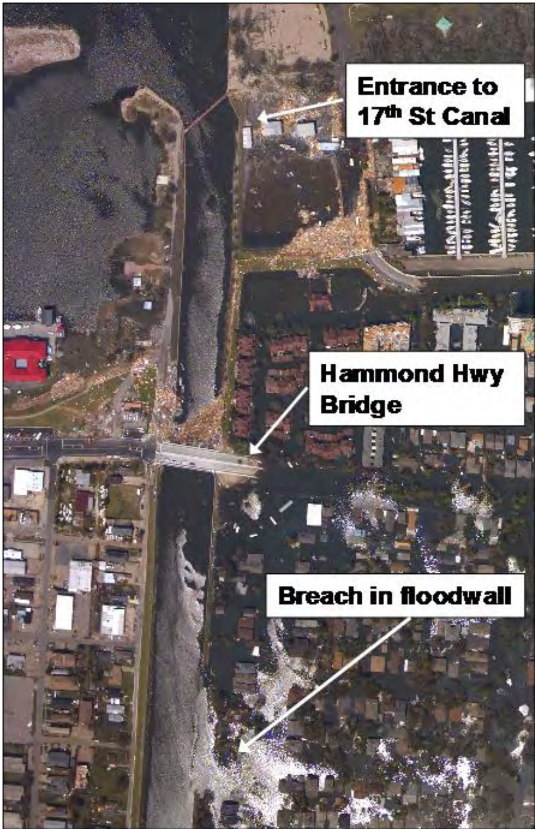
Figure 12-1. 17th Street Canal entrance region, Hammond Highway Bridge, and breach location
