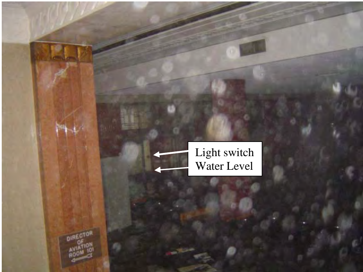
Figure 1-37. Time = 8:28 AM, APH-15. Door at south side of terminal building lobby
