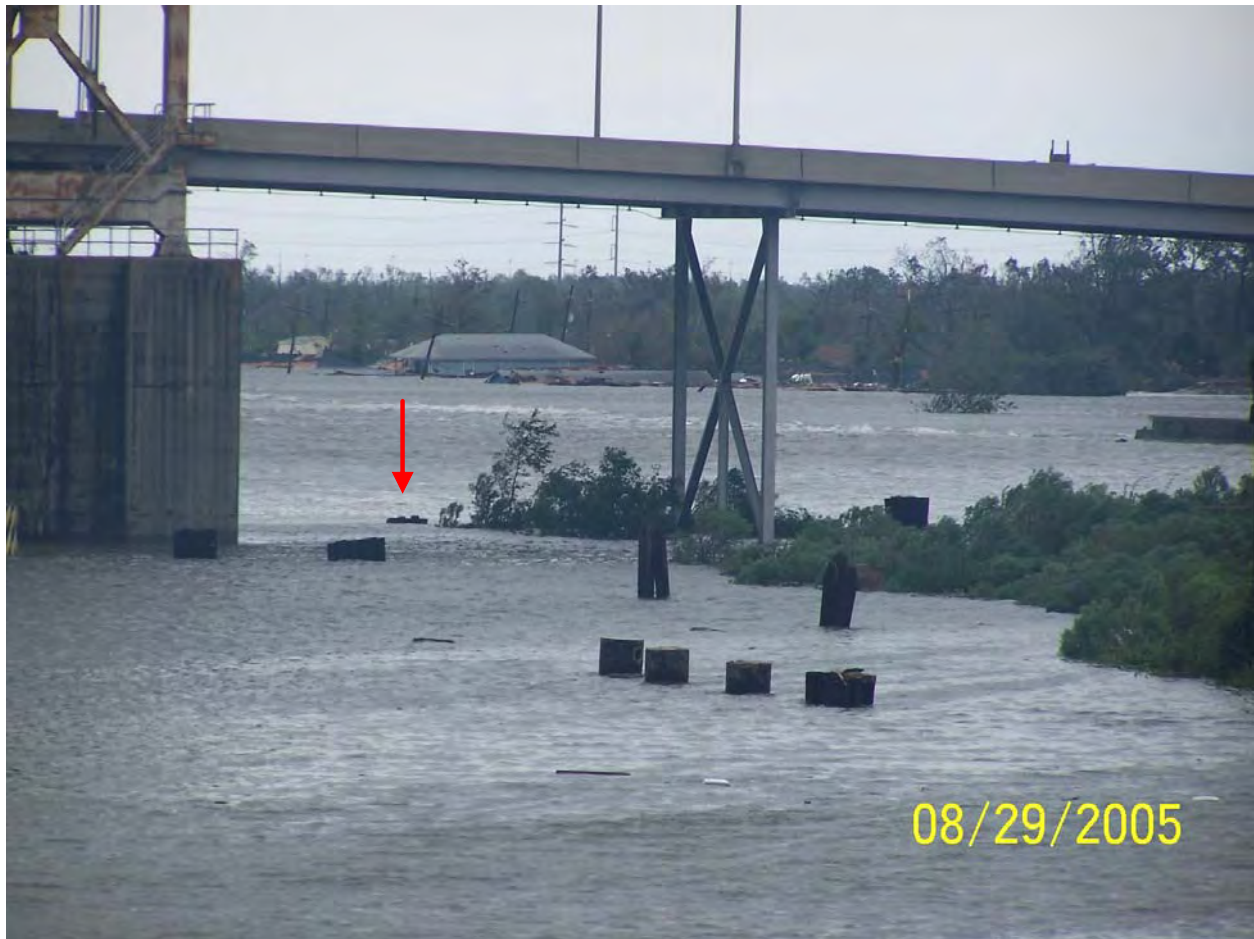
Figure 1-62. Time 3:03 PM, picture 100_0508. Breach on east side of IHNC in background. Looking northeast into Lower Ninth Ward.
