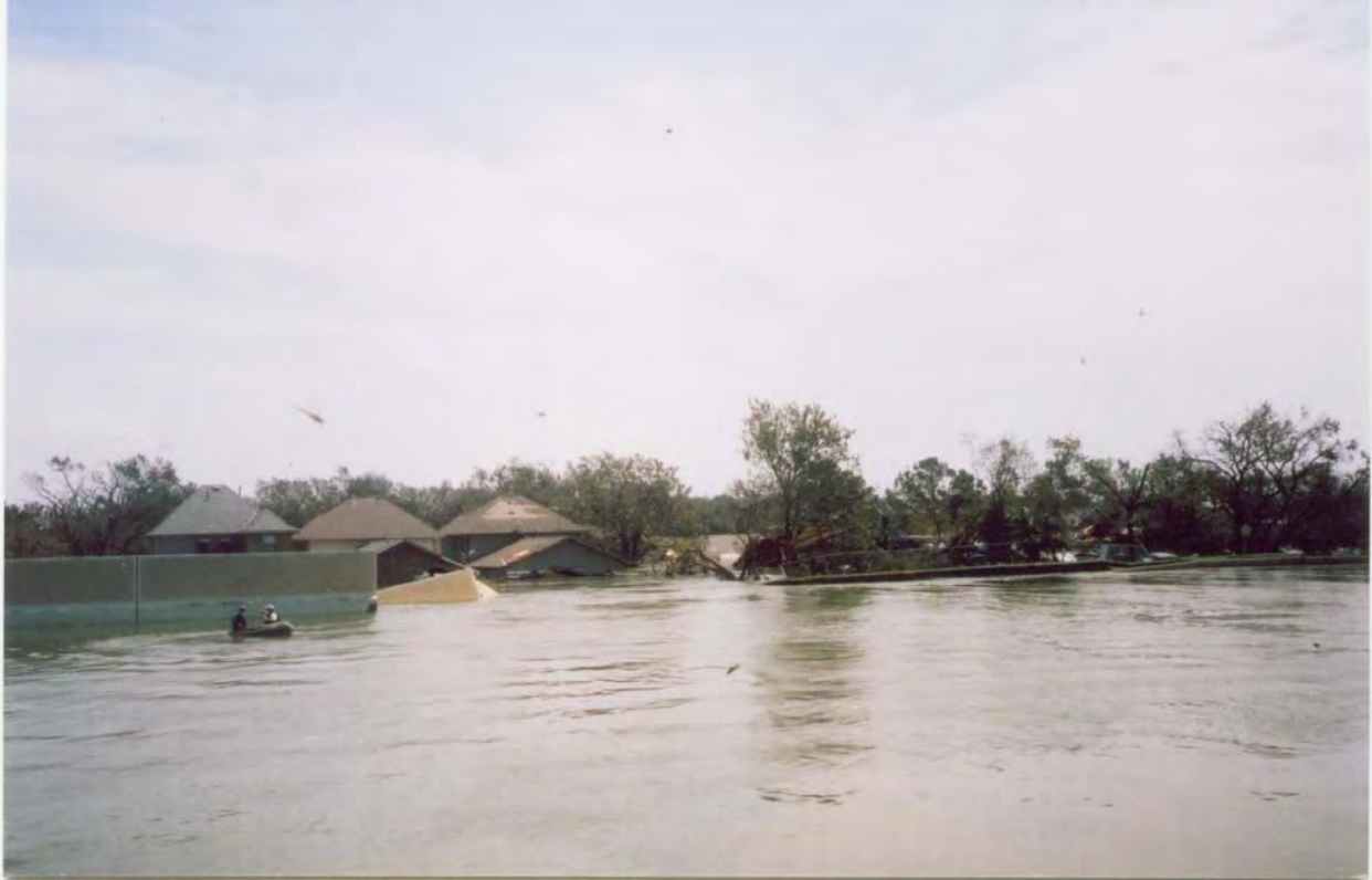
Figure 1-89. North end of 17th Street Canal breach at 3 PM on 8/29/05.
