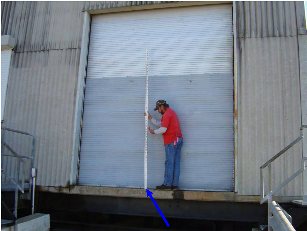
Finished Floor = 16.38 feet NAVD88(2004.65) Field Book 060854
