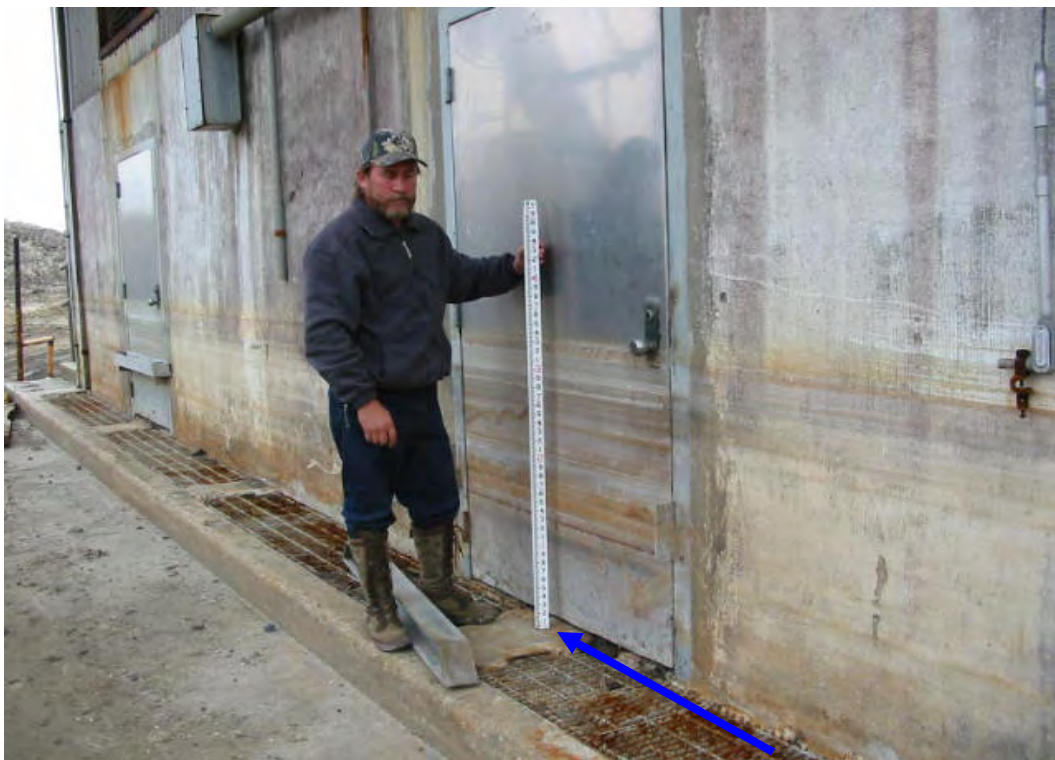
Finished Floor #1 = -0.18 feet NAVD88(2004.65) Field Book 060851
