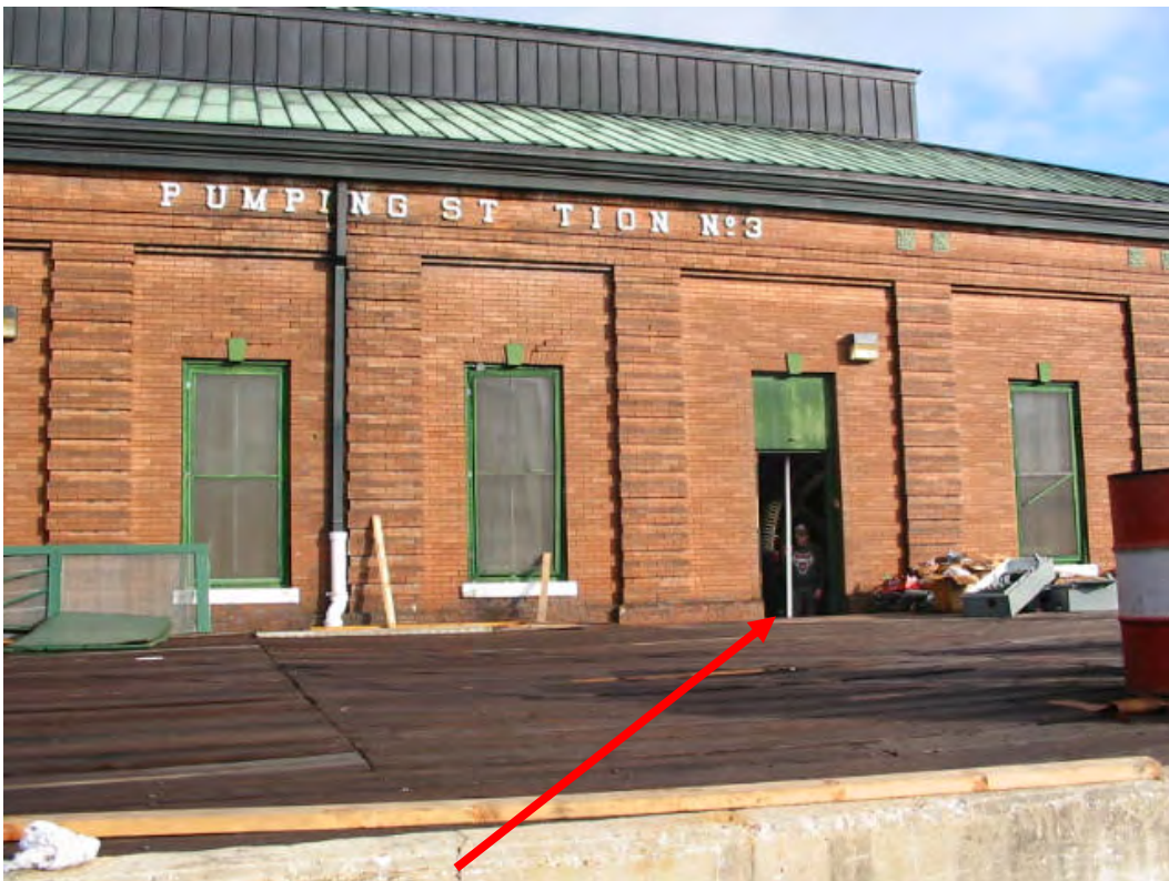
Finished Floor = 1.23 feet NAVD88(2004.65) Field Book 060851
