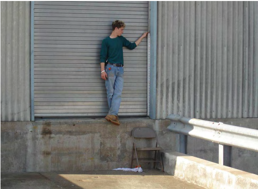
Finished Floor = 10.37 feet NAVD88(2004.65) Field Book 060854
