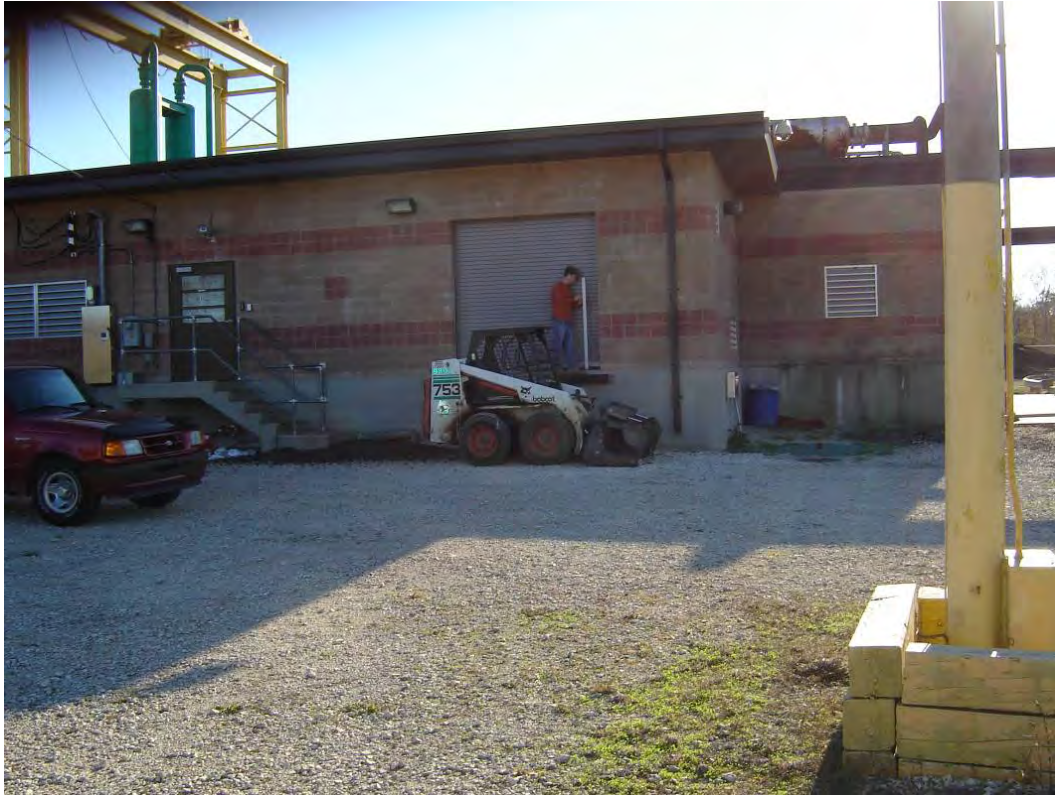
Estelle #2 Pump Station
