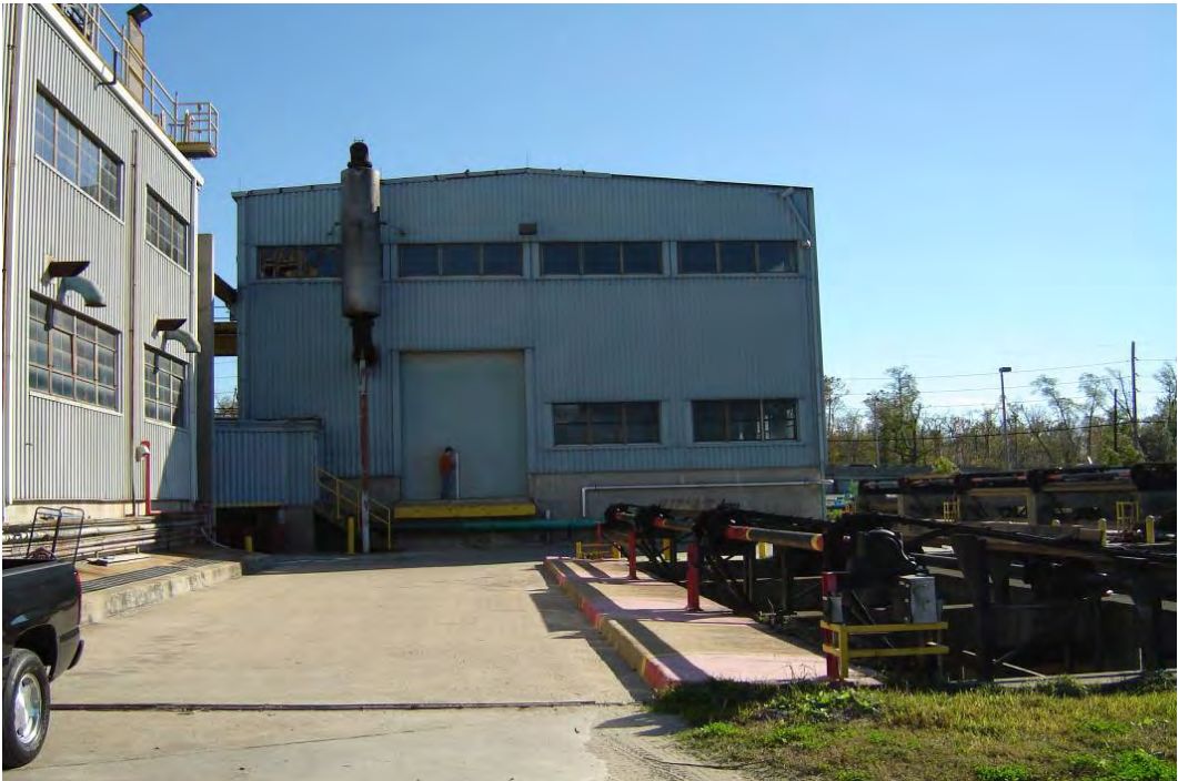
Cousins #2 Pump Station
