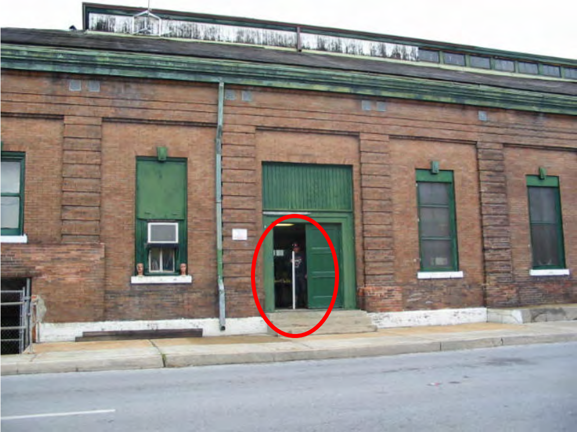
OP #2 PUMP STATION
