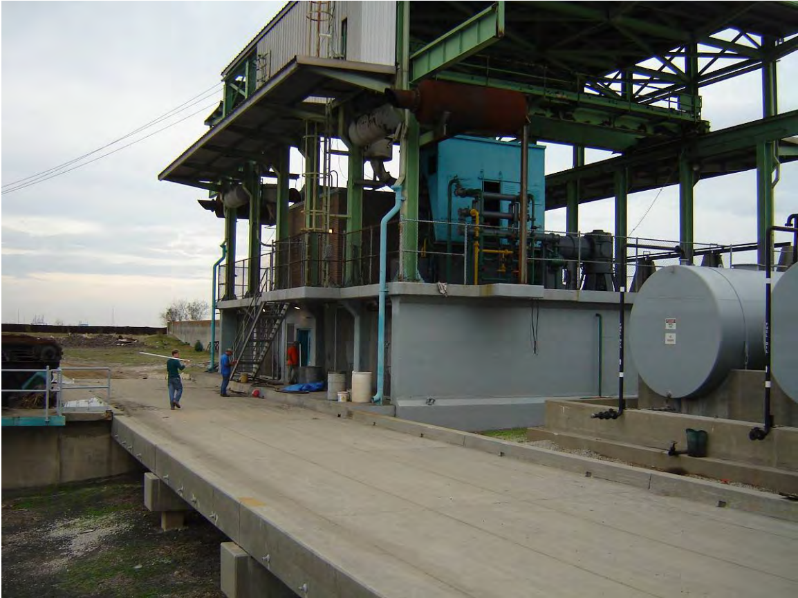
Finished Floor = 1.31 feet NAVD88(2004.65) Field Book 060851
