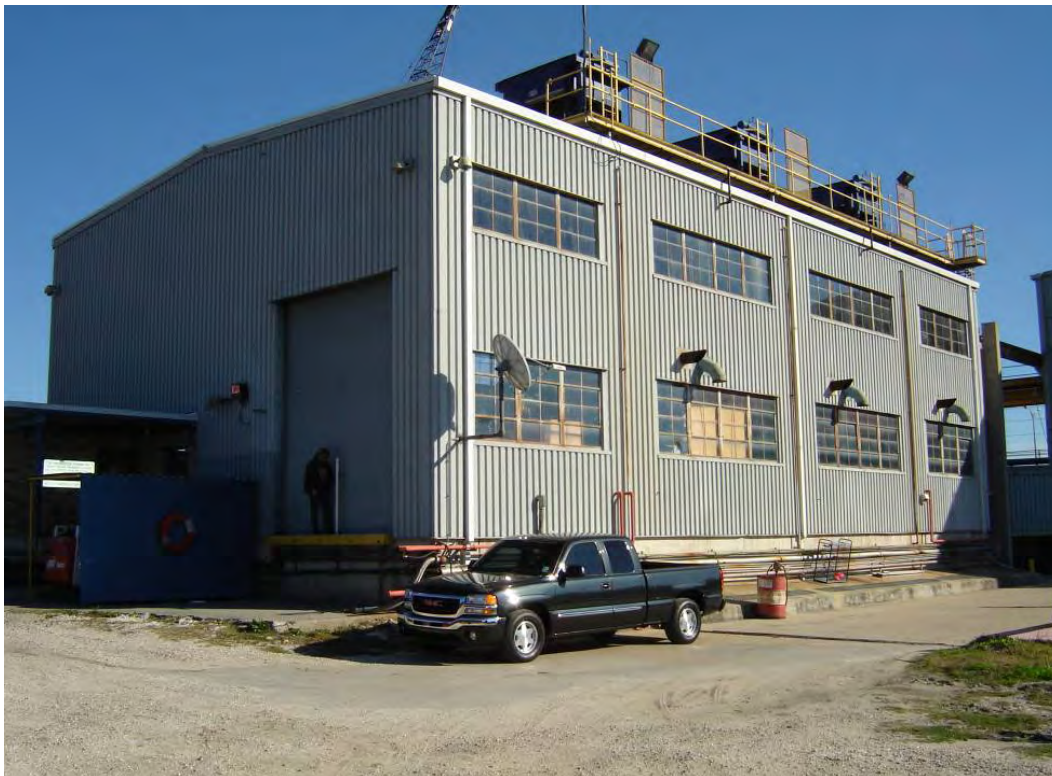
Cousins #1 Pump Station
