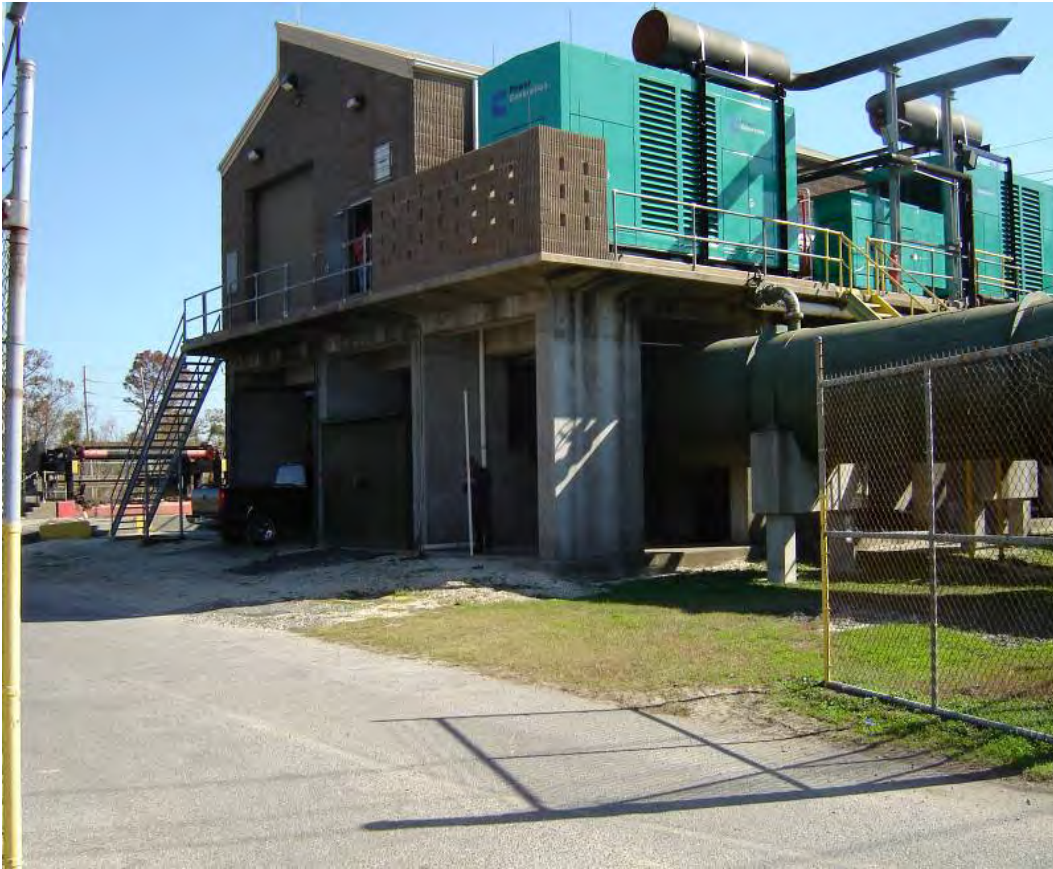
Parish Line Pump Station
