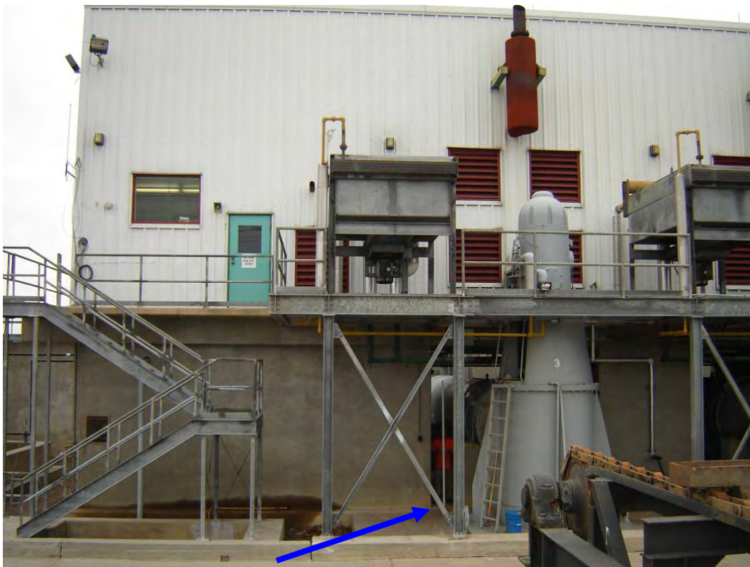
Finished Floor #2 = 2.50 feet NAVD88(2004.65) Field Book 060851
