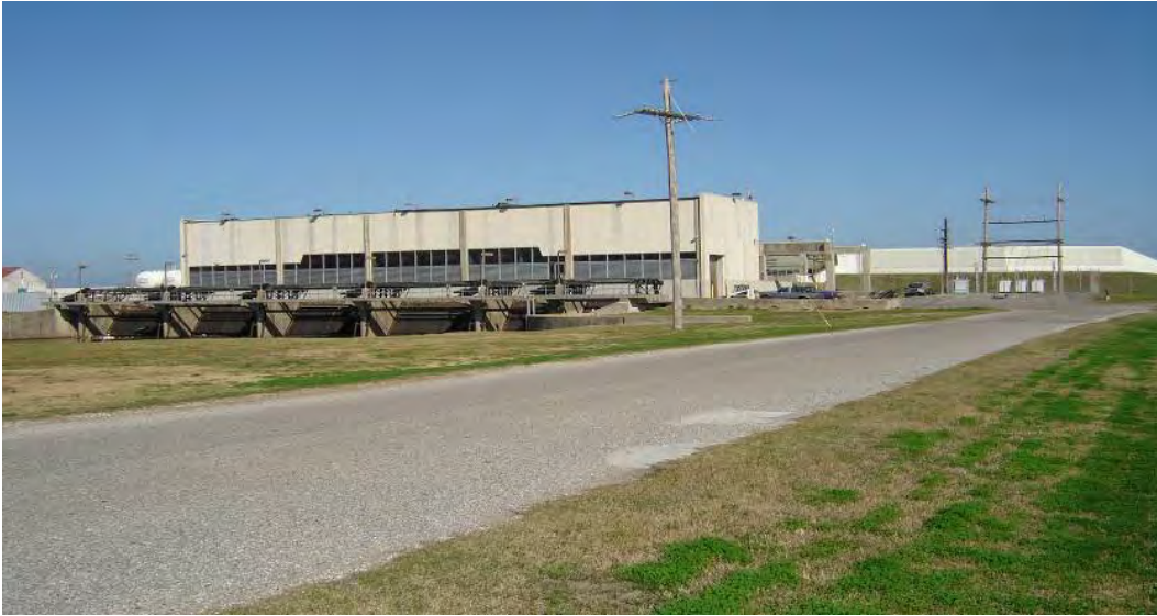
Pump Station JP-04
