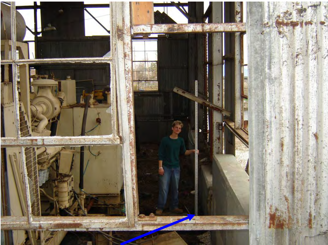
Finished Floor = 1.91 feet NAVD88(2004.65) Field Book 060851
