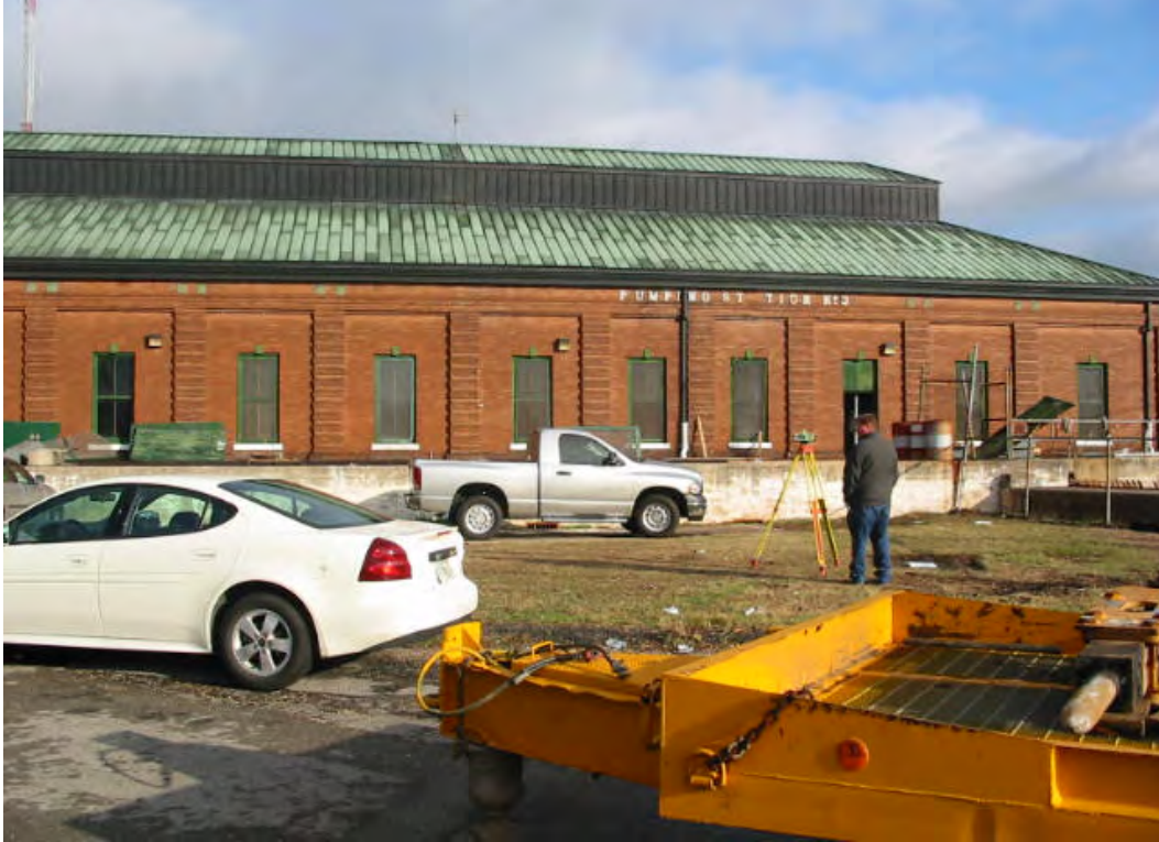
OP #3 Pump Station
