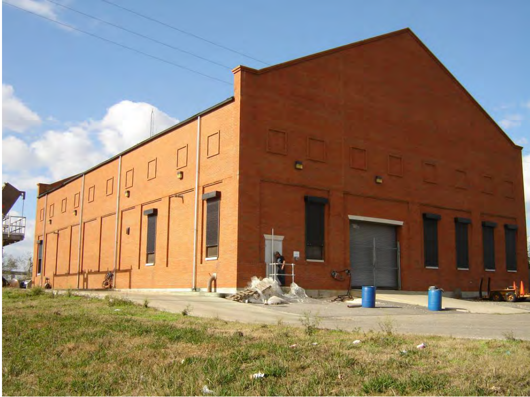
OP 11 PUMP STATION
