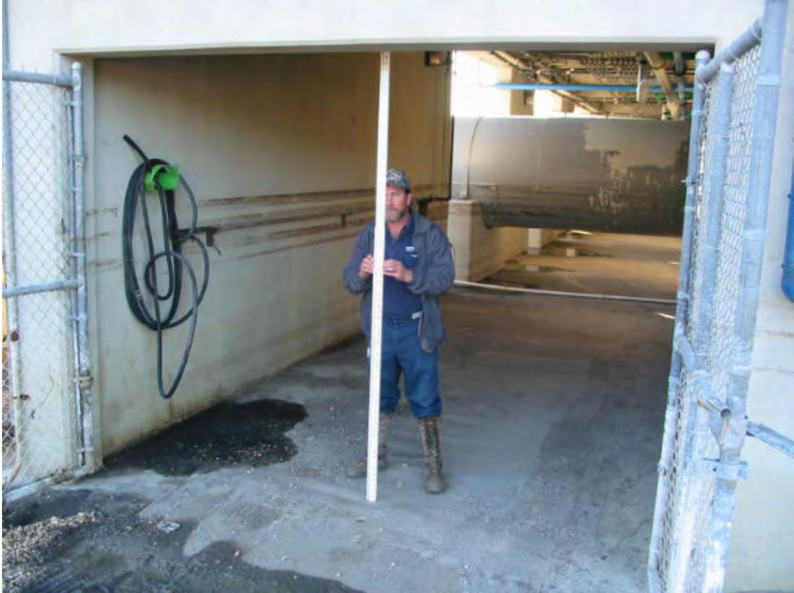
Finished Floor = 1.24 feet NAVD88(2004.65) Field Book 060851
