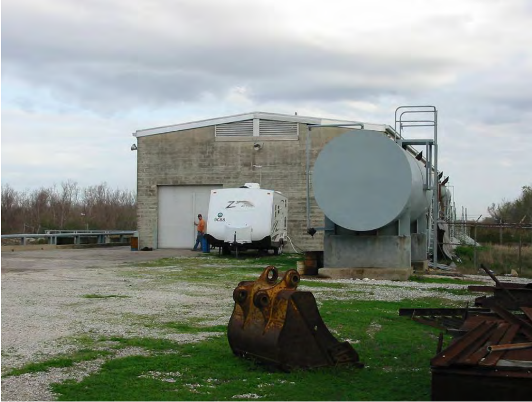
SCARSDALE PUMP STATION
