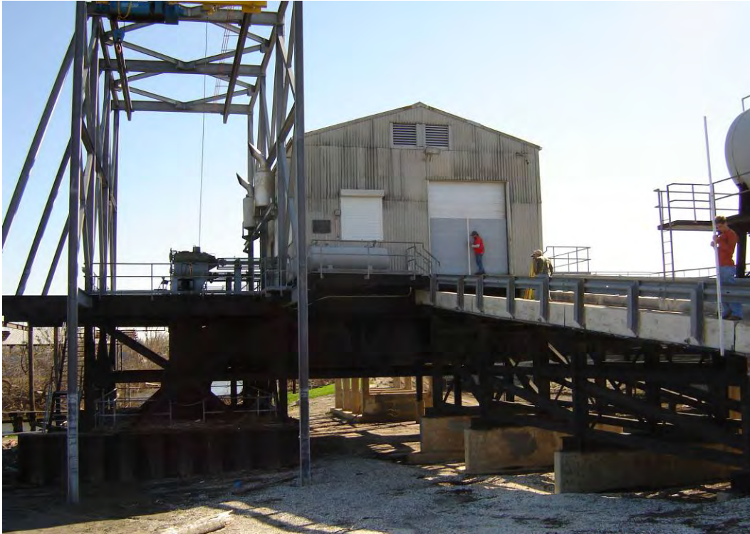
DUVIC(VENICE) PUMP STATION
