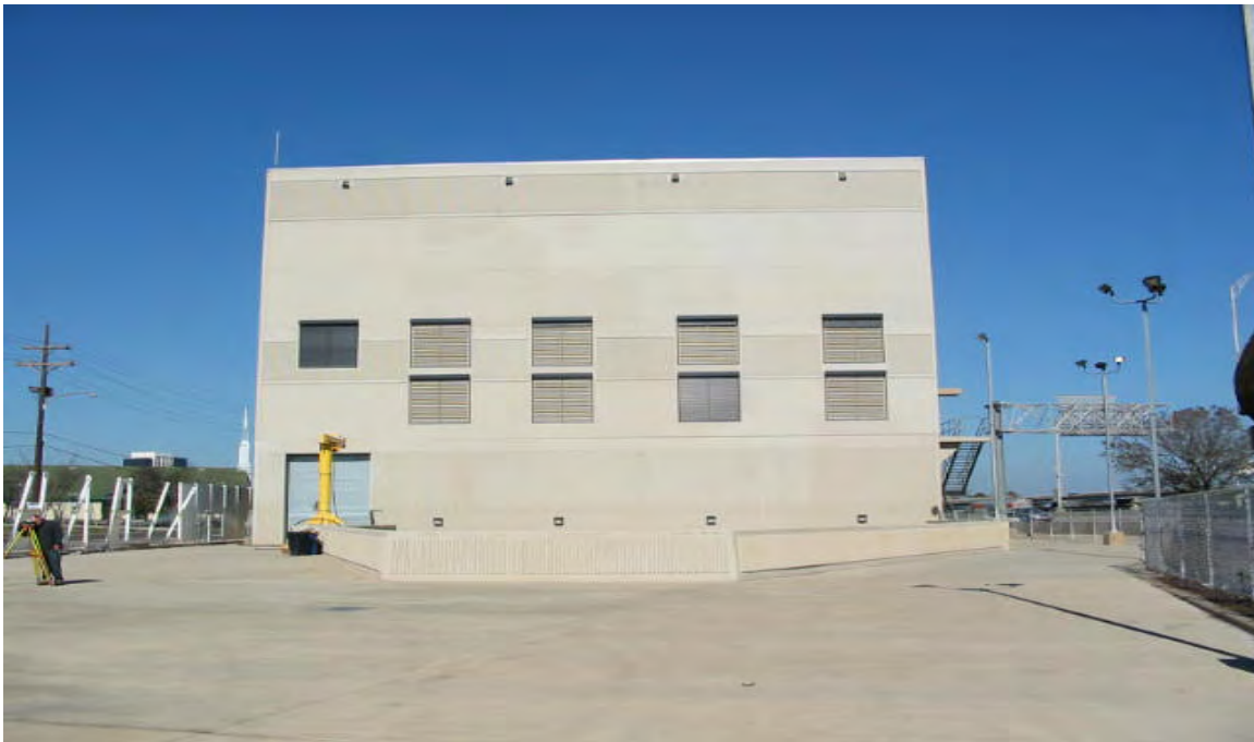
I-10 Pump Station
