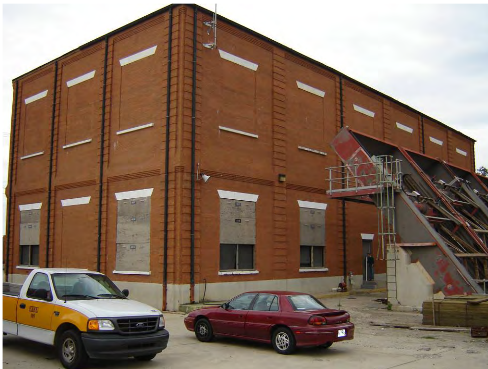
Citrus Pump Station OP 10
