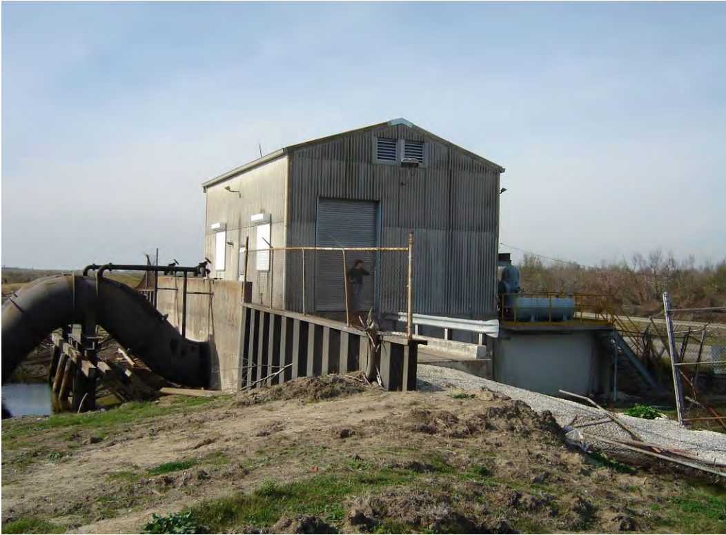
DIAMOND PUMP STATION
