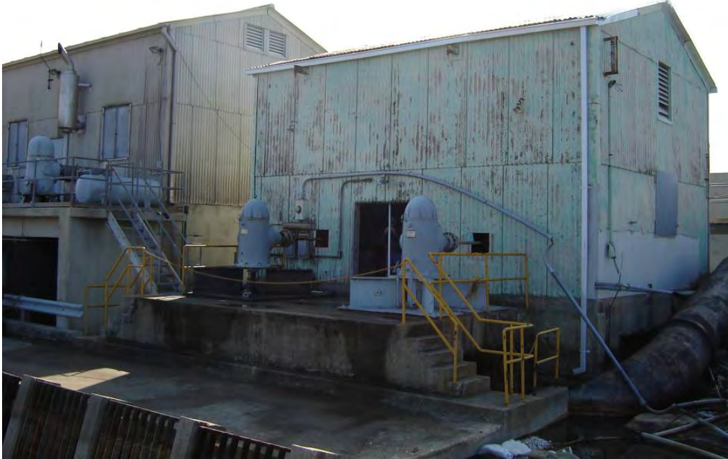
SUNRISE #1 PUMP STATION
