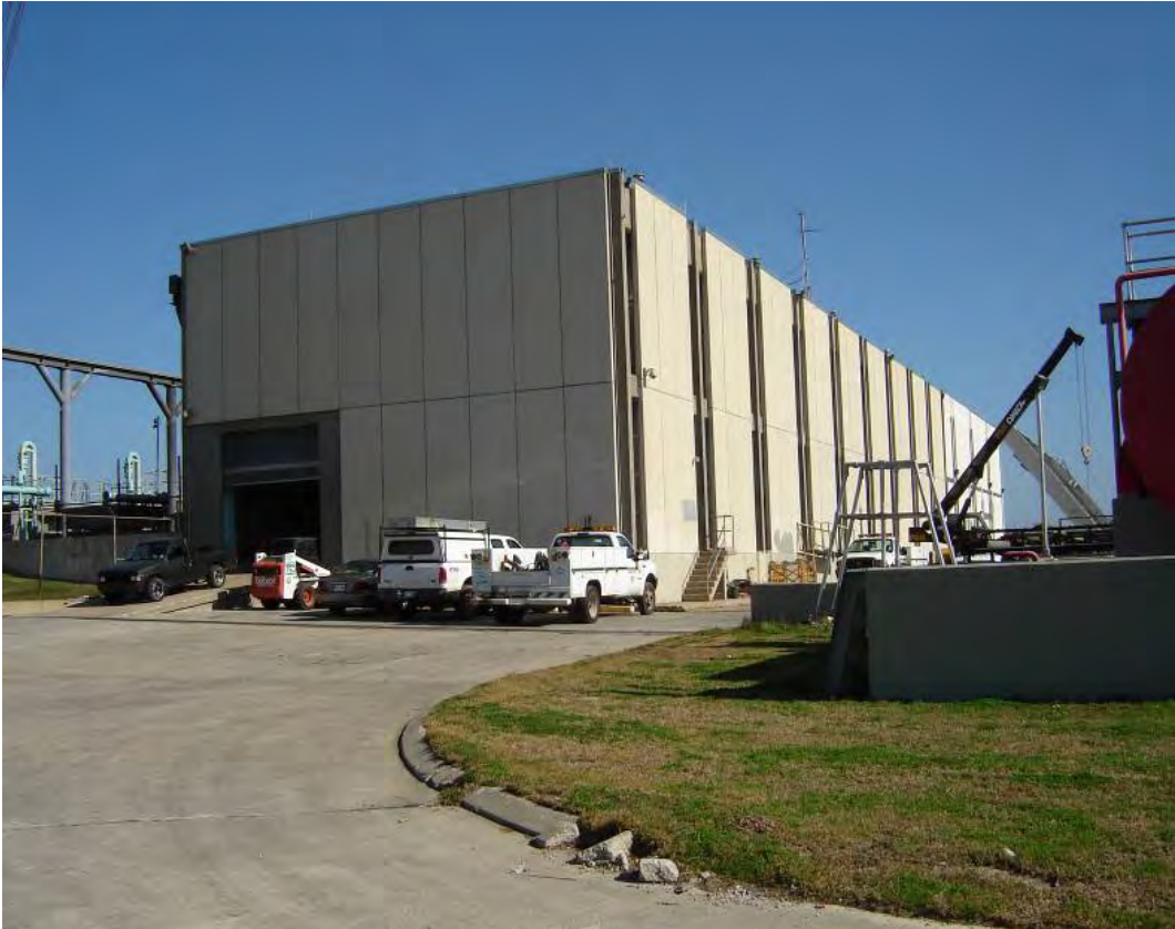
Elmwood Canal Pump Station JP-03
