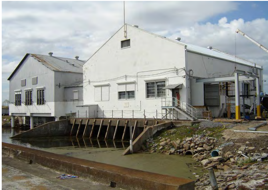
BELLE CHASE #1 Pump Station
