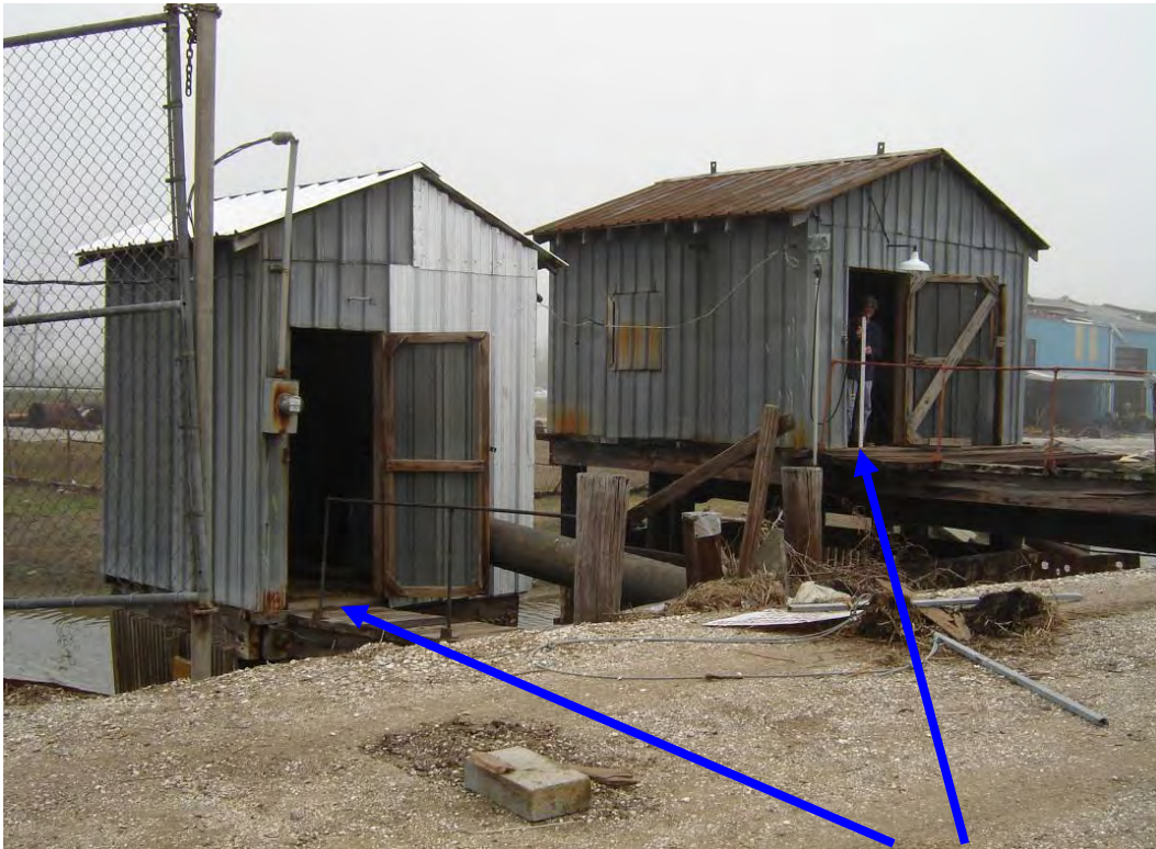
POINTE A LA HACHE PUMP STATION WEST 1 & 2
