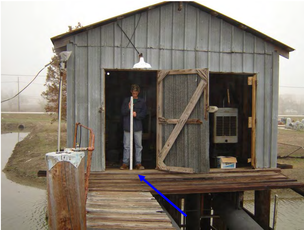
Finished Floor #2 = 6.82 feet NAVD88(2004.65) Field Book 060854
