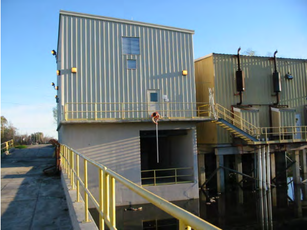
Finished Floor #1 = 14.21 feet NAVD88(2004.65) Field Book 060858
