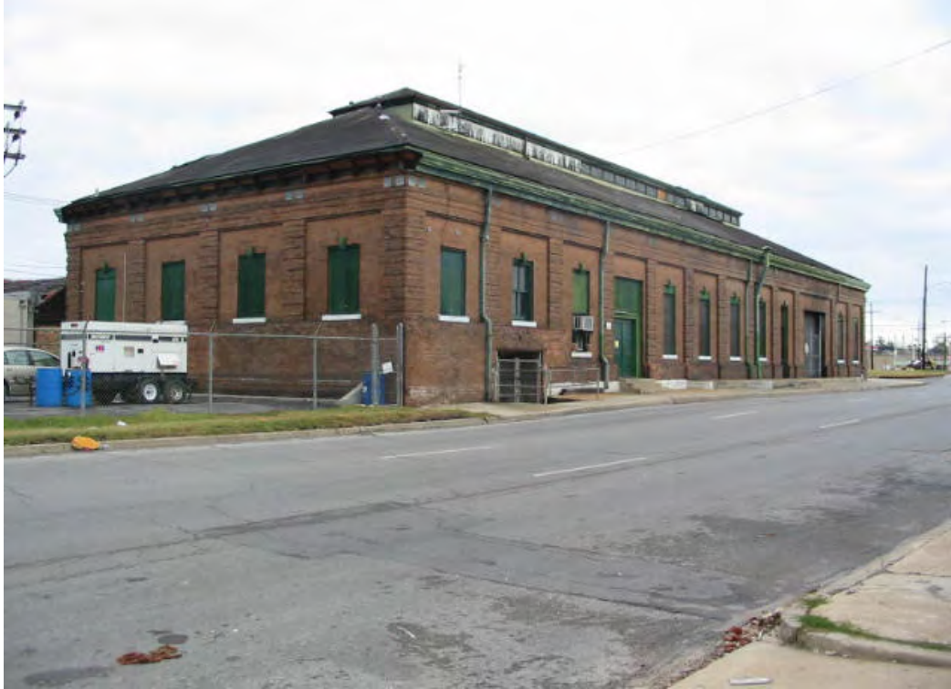
OP #2 Pump Station
