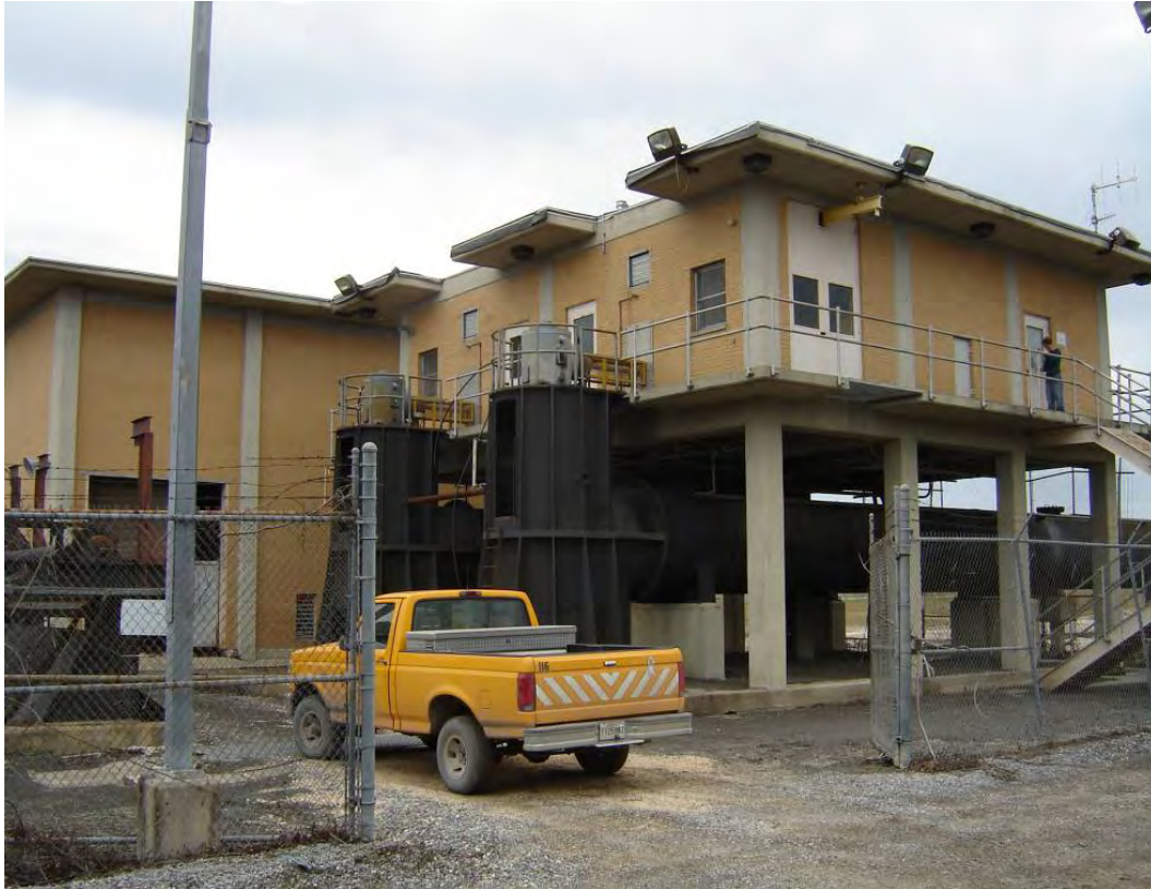
OP 20 Amid Pump Station
