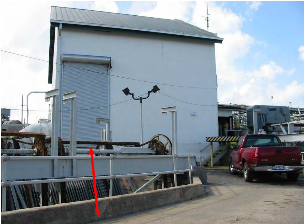
Finished Floor = 2.53 feet NAVD88(2004.65) Field Book 060851
