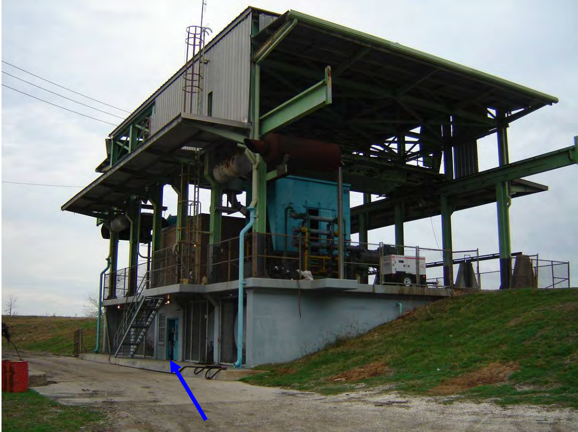
Finished Floor #2 = 2.43 feet NAVD88(2004.65) Field Book 060851
