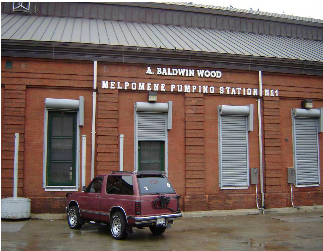
OP #1 Melpomene Pump Station #1
