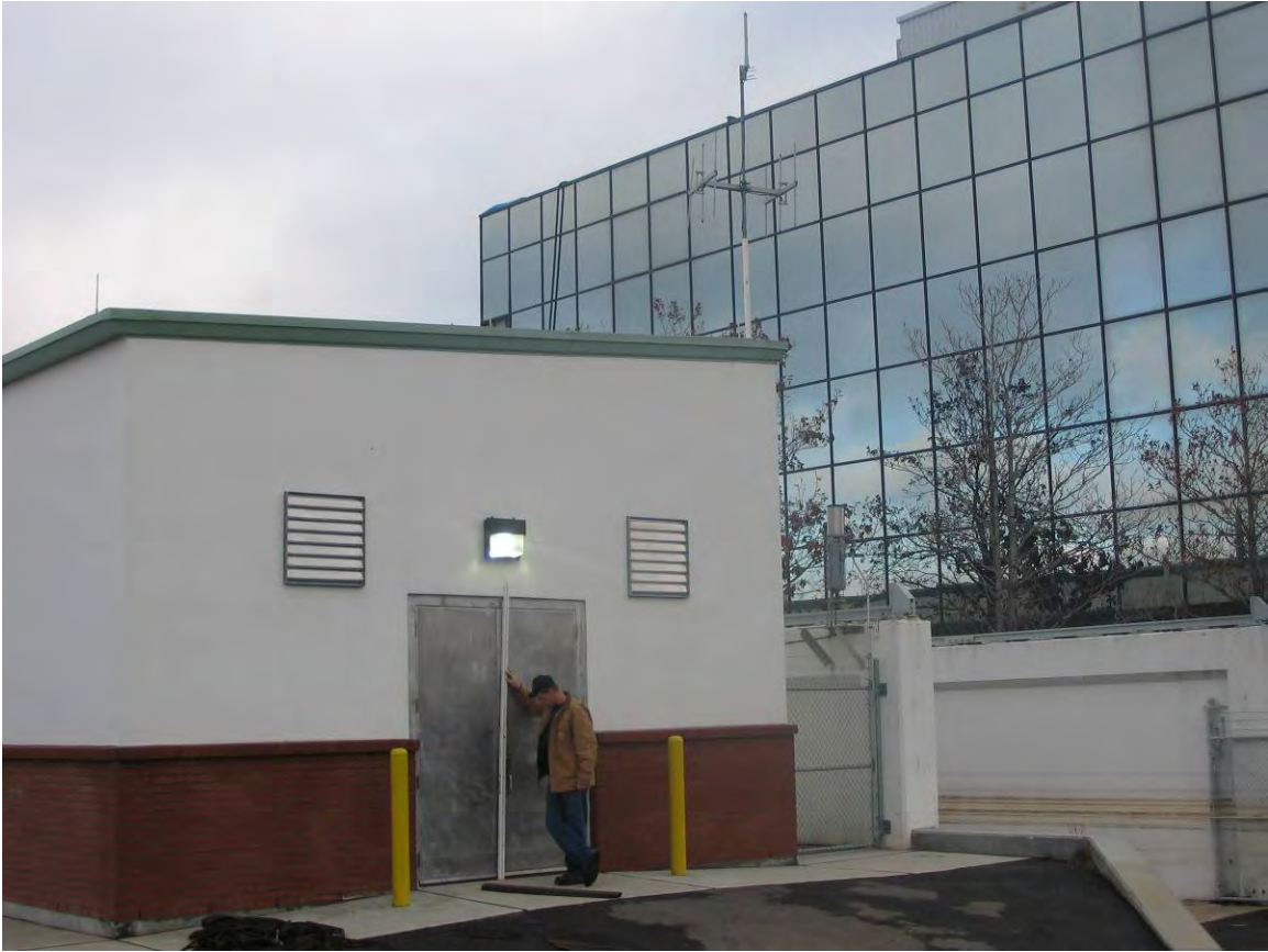
OP 12 Finished Floor = 0.44 feet NAVD88(2004.65) Field Book 060851
