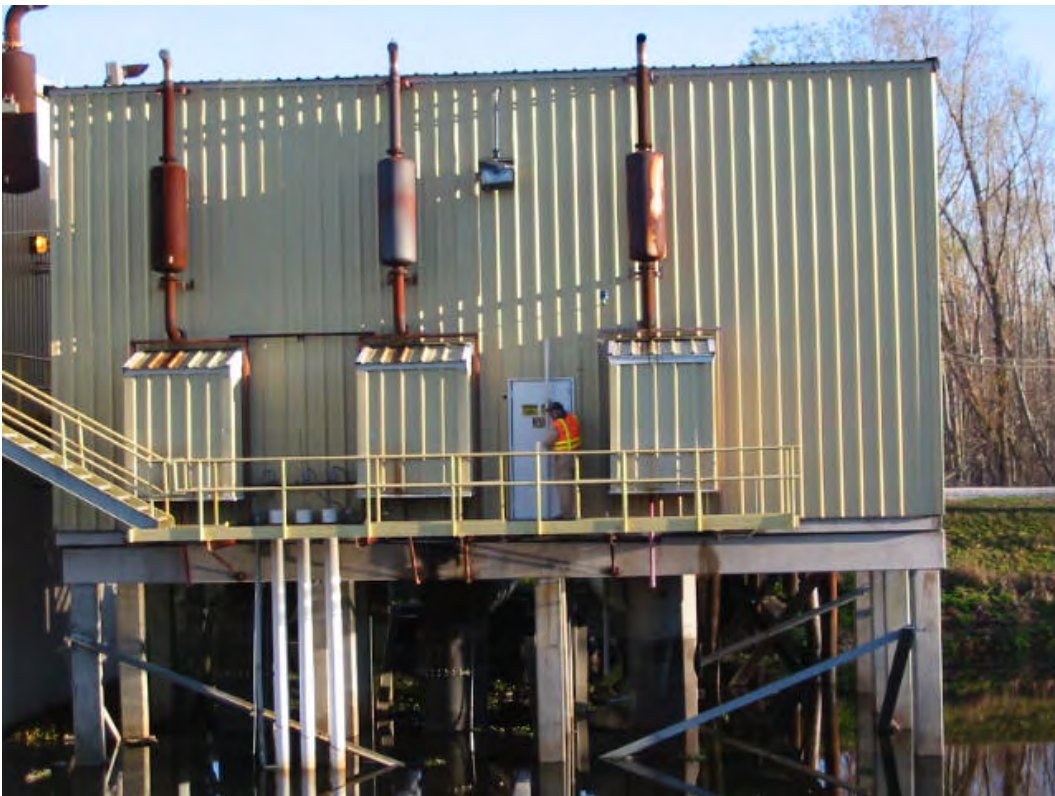
Finished Floor #2 = 8.39 feet NAVD88(2004.65) Field Book 060858
