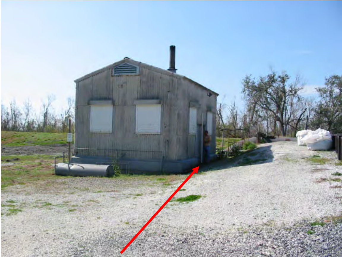
Ollie Lower Pump Station Finished Floor = 3.44 feet NAVD88(2004.65) Book 060858
