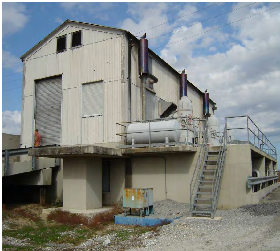
Belle Chase #2 Pump Station
