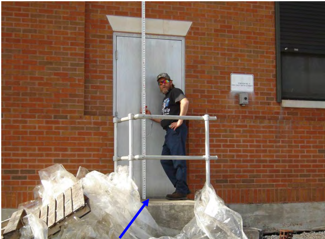
Finished Floor = 2.62 feet NAVD88(2004.65) Field Book 060852
