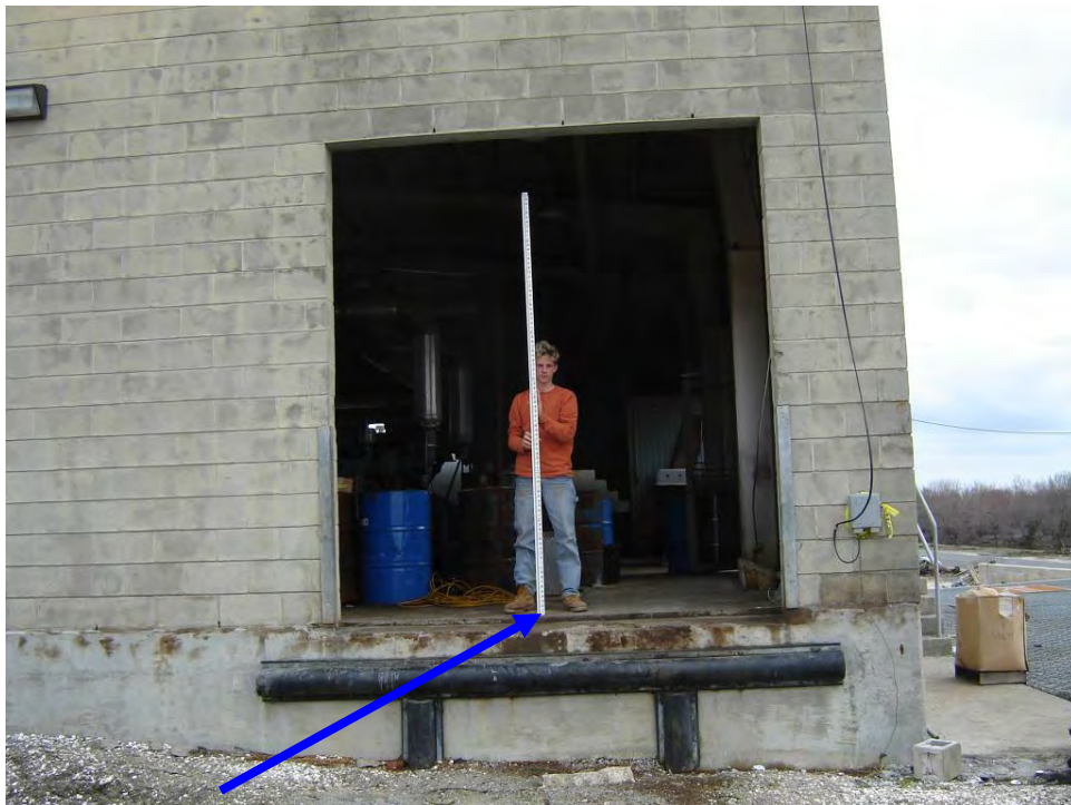
Finished Floor = 12.59 feet NAVD88(2004.65) Field Book 060852
