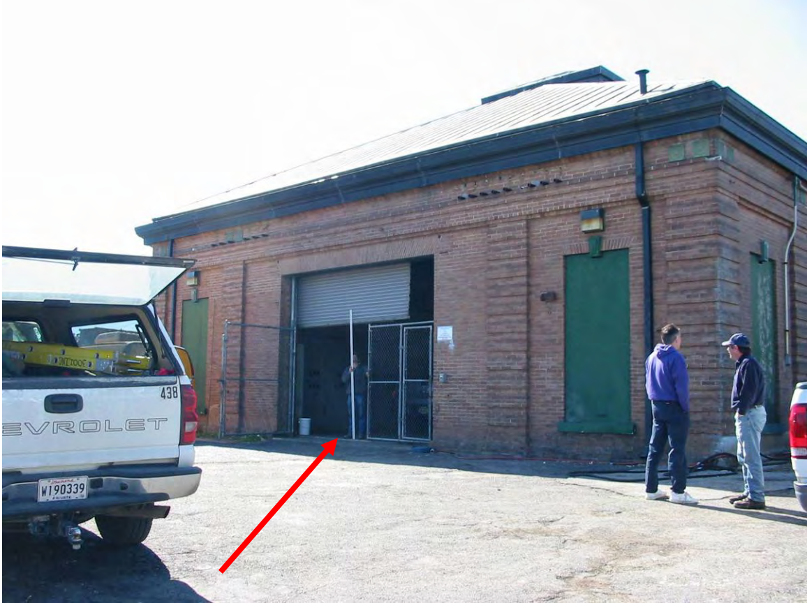
Finished Floor = 2.03 feet NAVD88(2004.65) Field Book 060851
