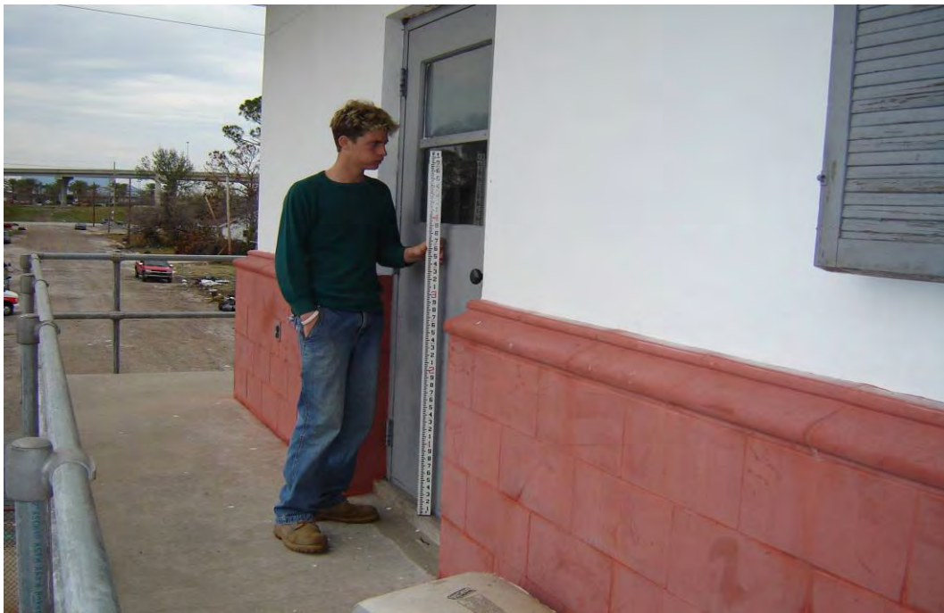
Finished Floor = 14.85 feet NAVD88(2004.65) Field Book 060851
