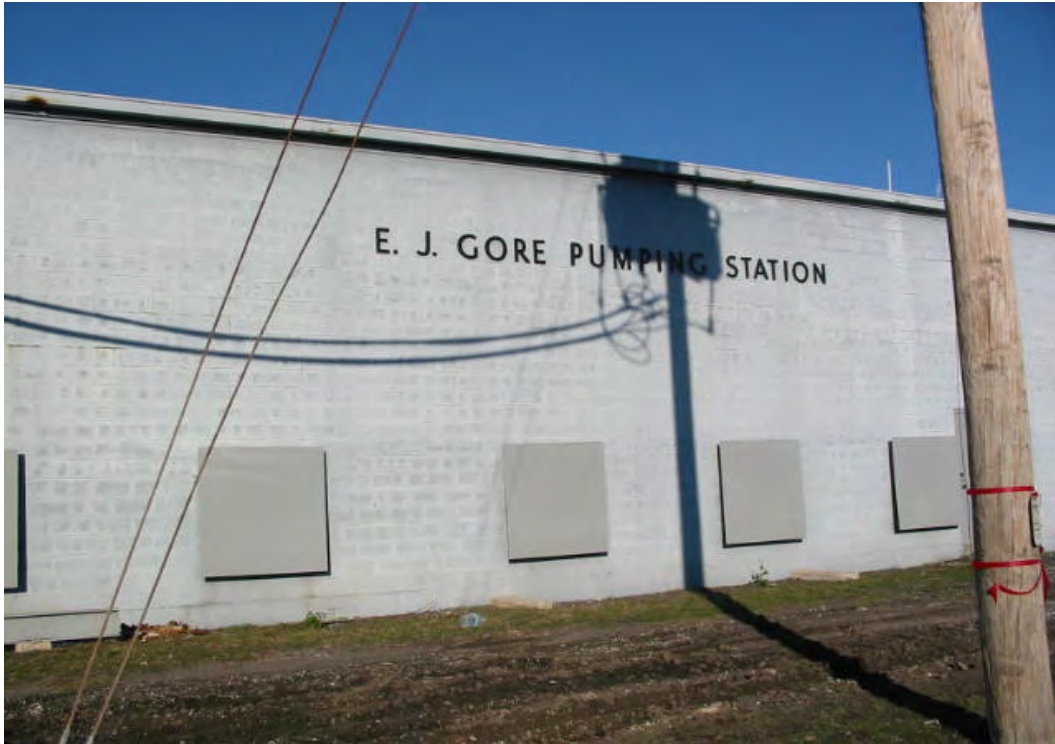
E.J. Gore Pump Station
