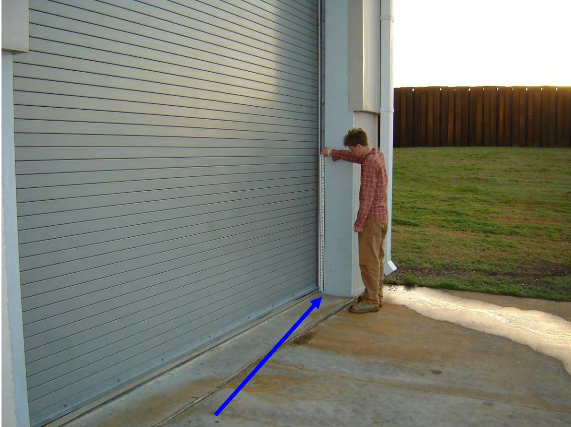
Finished Floor = -3.02 feet NAVD88(2004.65) Book # 060852
