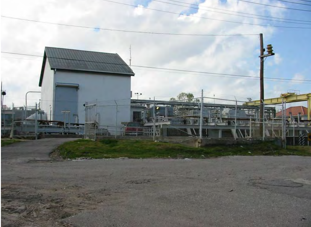
OP #4 Pump Station
