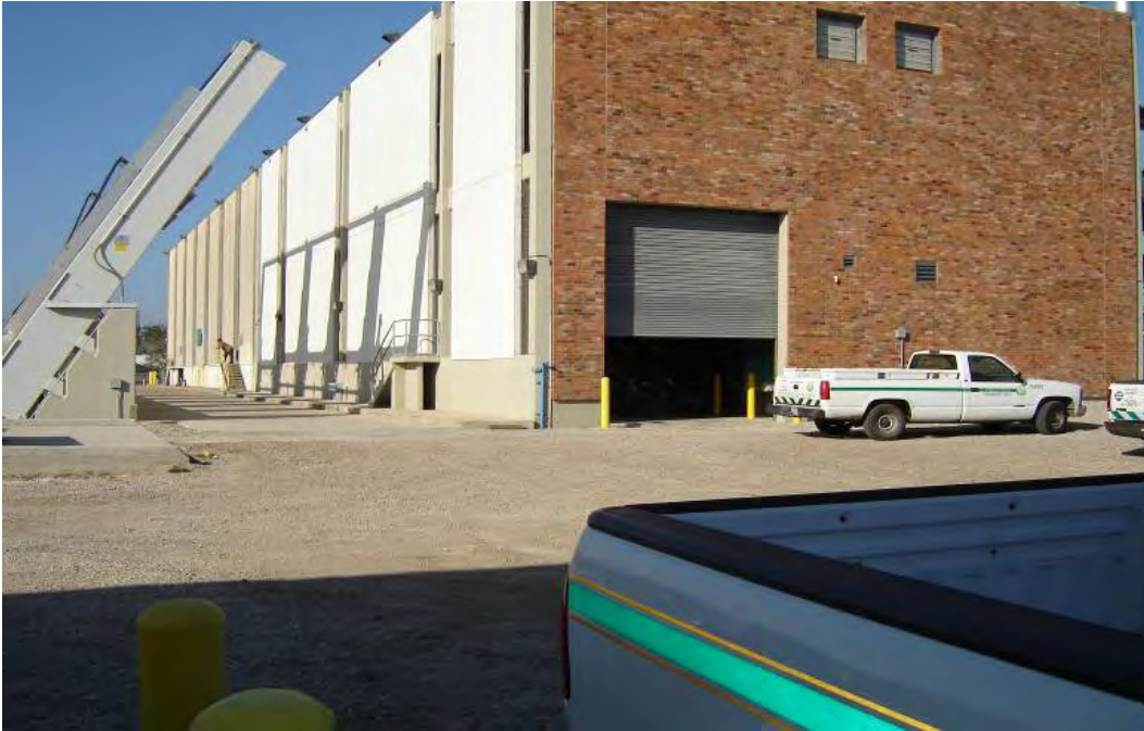
Pump Station JP-02
