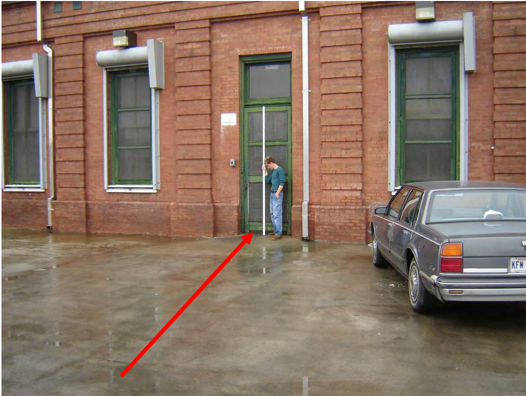
Finished Floor = 1.65 feet NAVD88(2004.65) Field Book 060851
