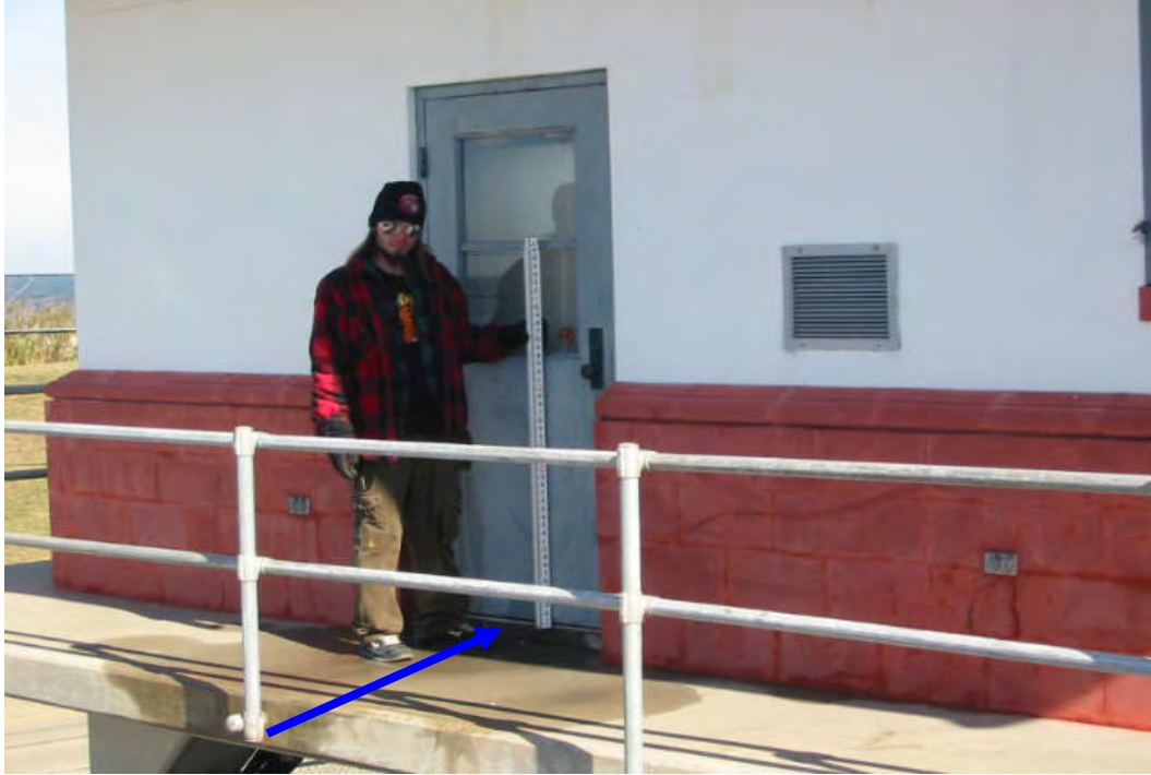
Finished Floor = 14.93 feet NAVD88(2004.65) Field book 060851
