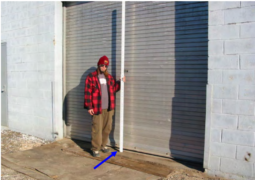
Finished Floor = 4.75 feet NAVD88(2004.65) Field Book 060851
