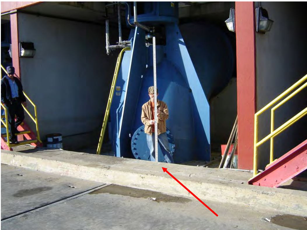
Finished Floor = -4.26 feet NAVD88(2004.65) Field Book 060852
