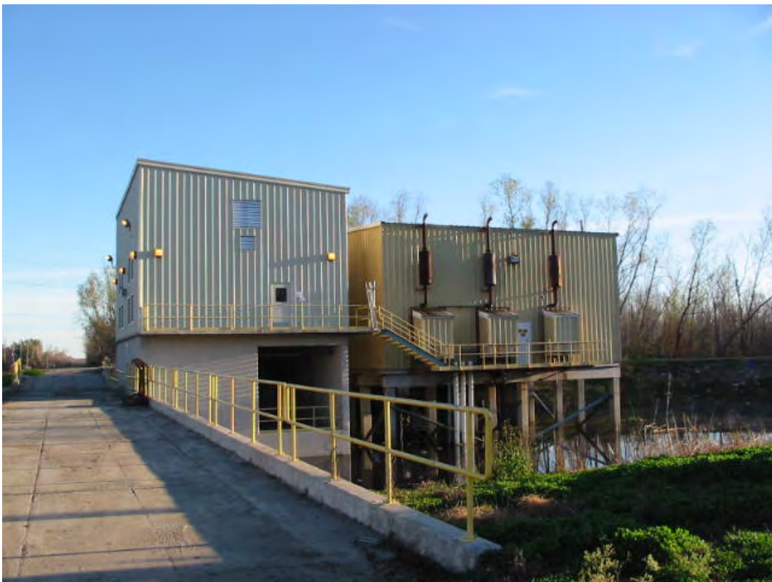
DESTREHAN #1 Pump Station
