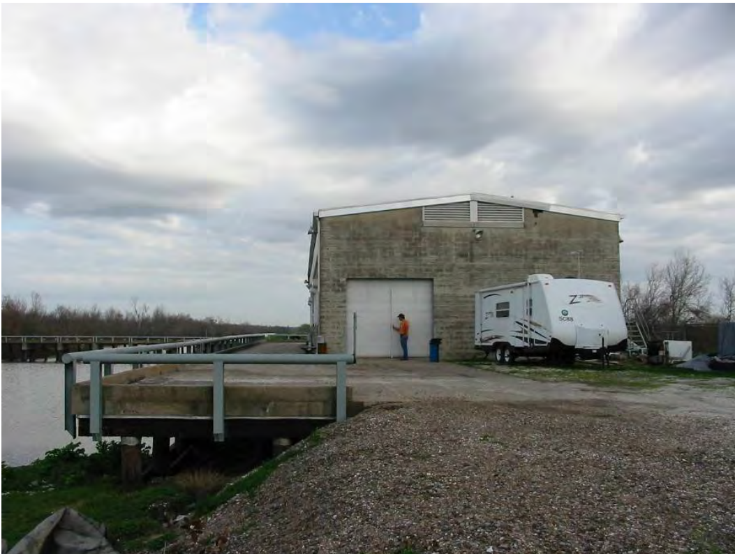
Finished Floor = 11.08 feet NAVD88(2004.65) Field Book 060852
