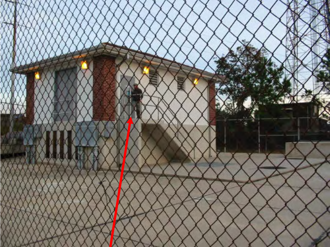
Finished Floor = 2.65 feet NAVD88(2004.65) Field Book 060851
