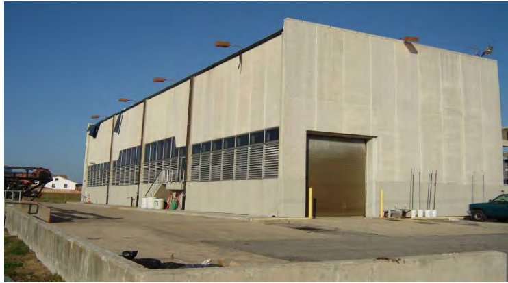
Pump Station JP-01
