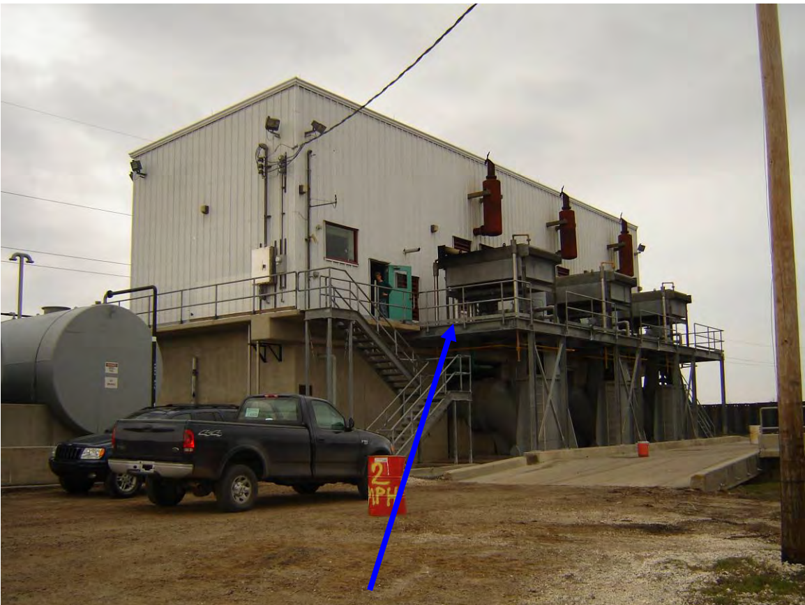
Finished Floor = 1.25 feet NAVD88(2004.65) Field Book 060851
