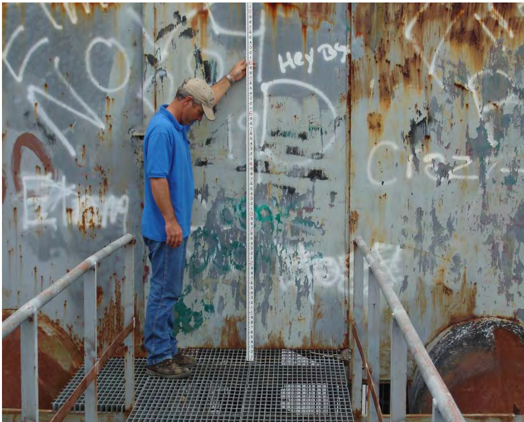
Finished Floor = 1.56 feet NAVD88(2004.65) Field book 060851
