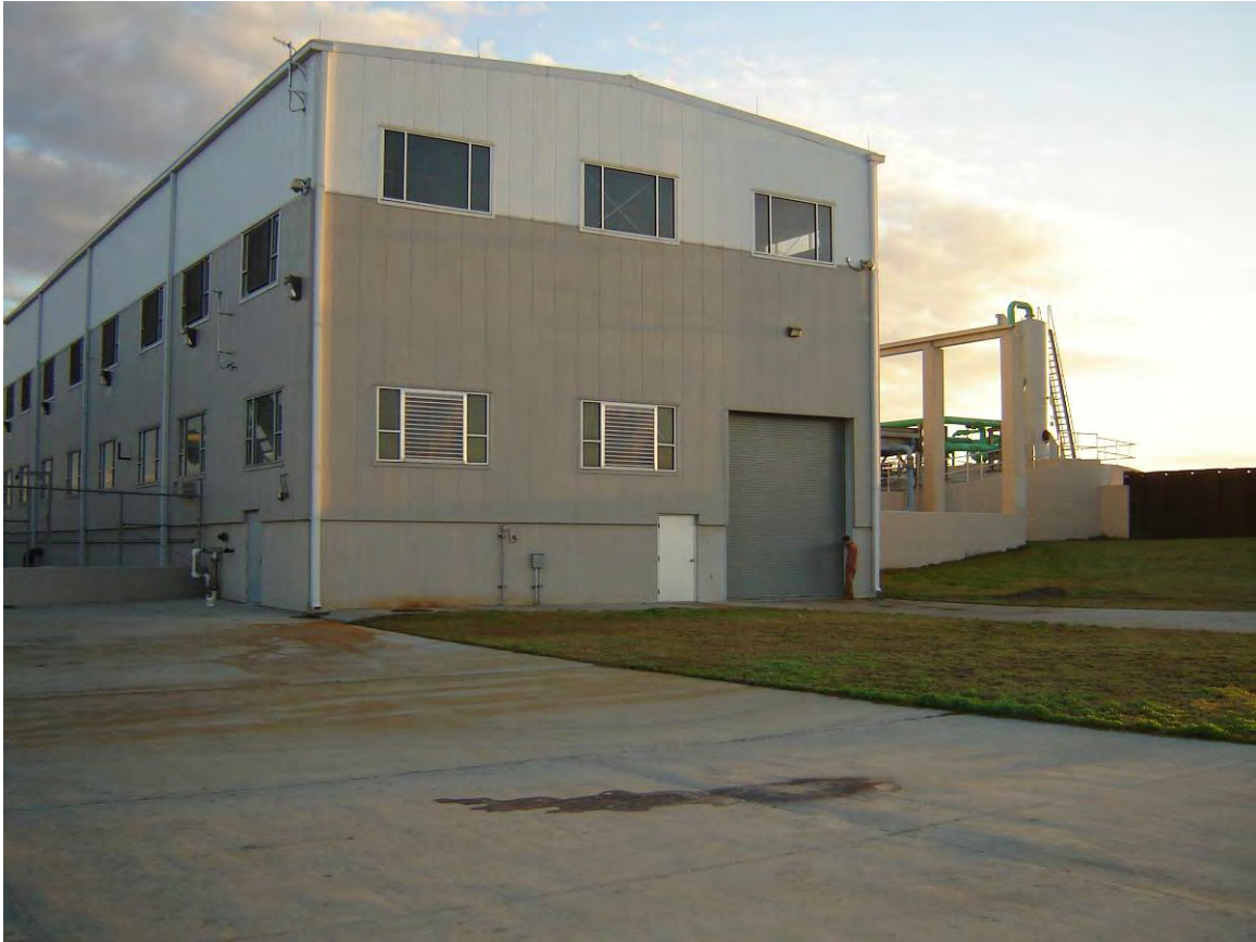
Whitney-Barataria Pump Station
