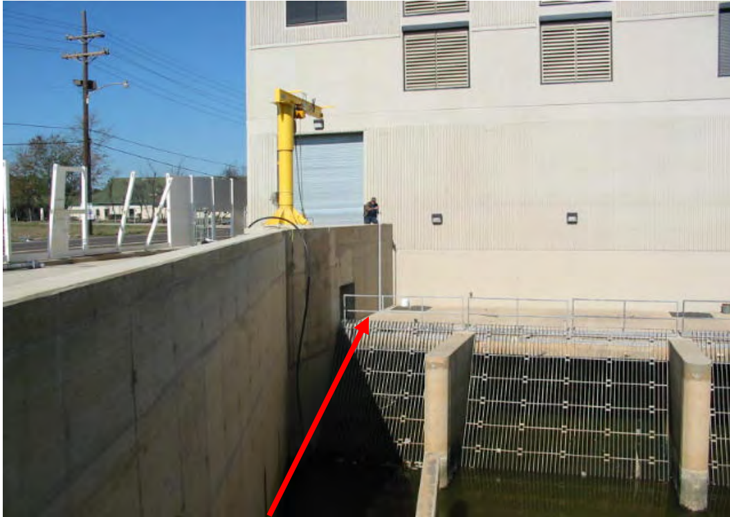
Finished Floor #1 = -11.60 feet NAVD88(2004.65) Field Book 060852
