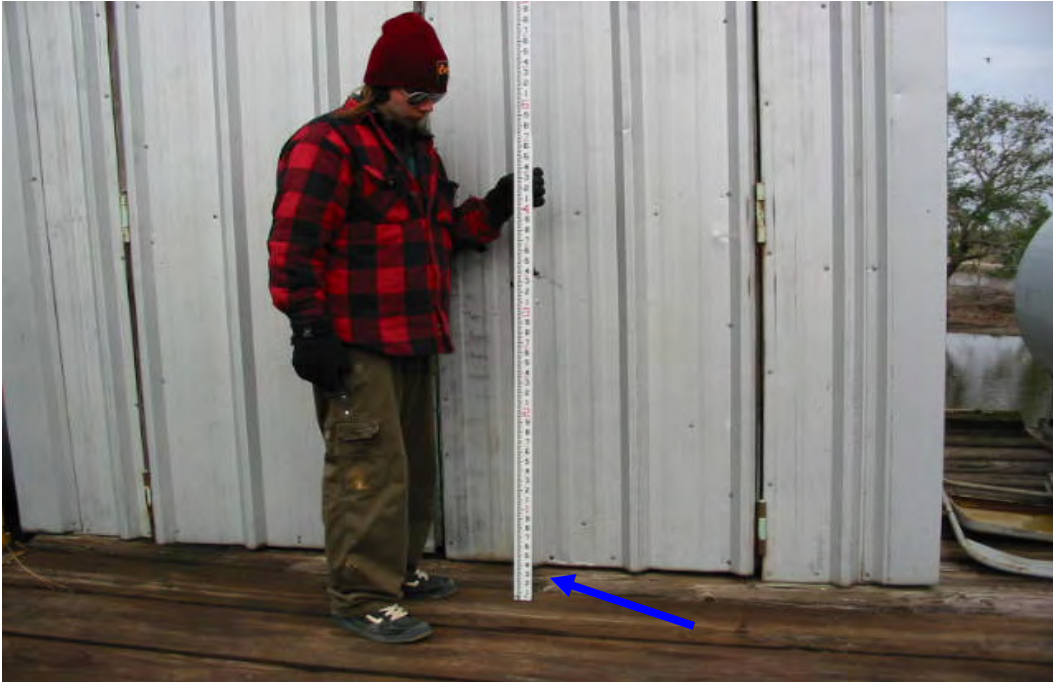
Finished Floor #1 = 7.81 feet NAVD88(2004.65) Field Book 060852
