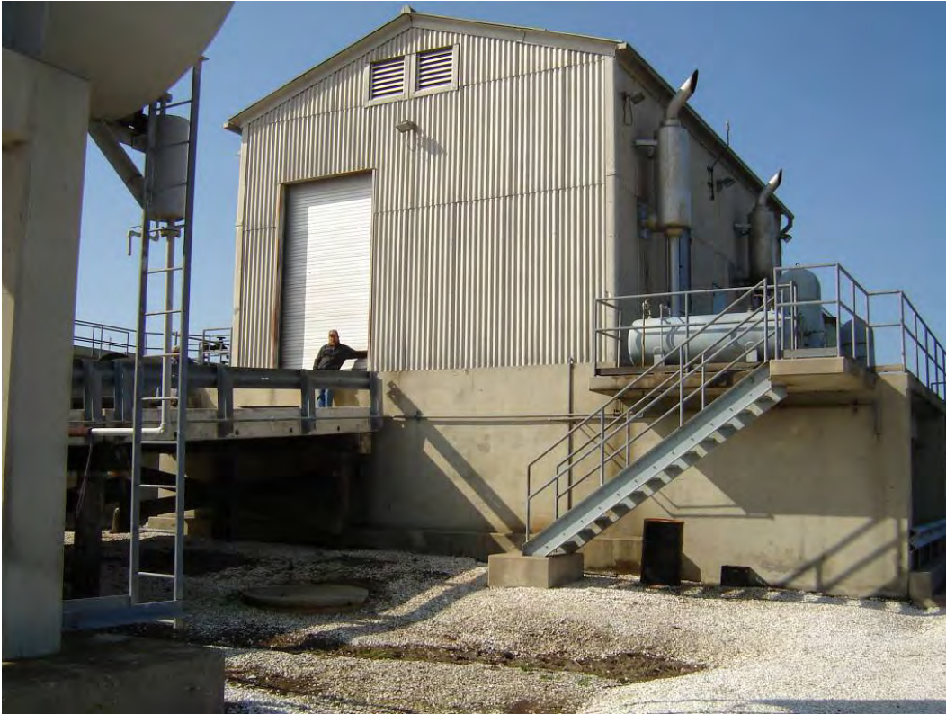
SUNRISE #2 PUMP STATION
