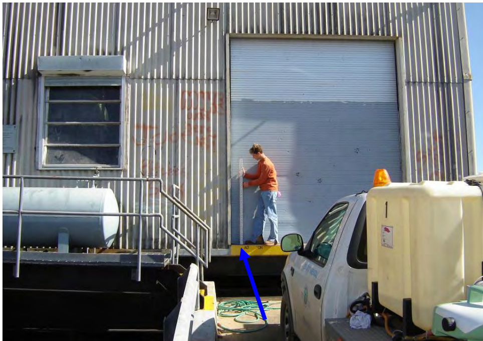
Finished Floor #3 = 9.27 feet NAVD88(2004.65) Field Book 060854
