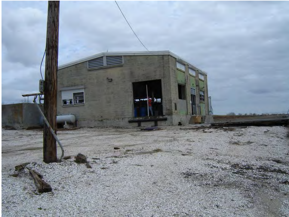
POINTE A La HACHE EAST PUMP STATION
