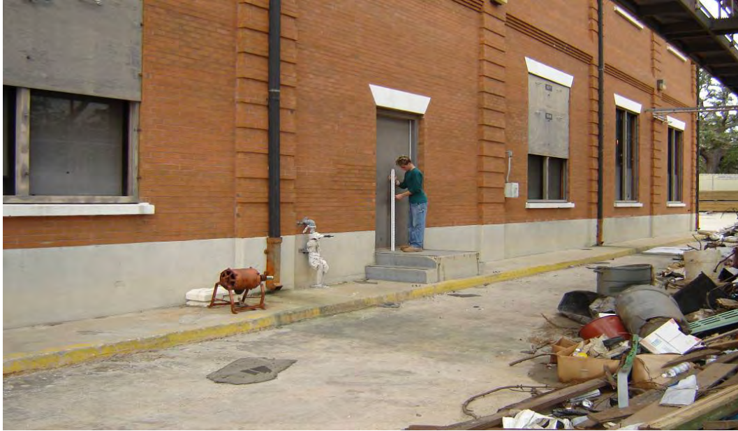
Finished floor = -1.50 feet NAVD 88 2004.65 Field book 060851
