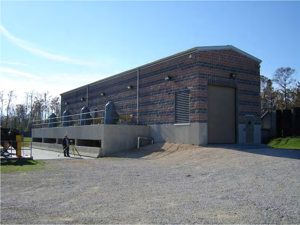
Westminister Pump Station
