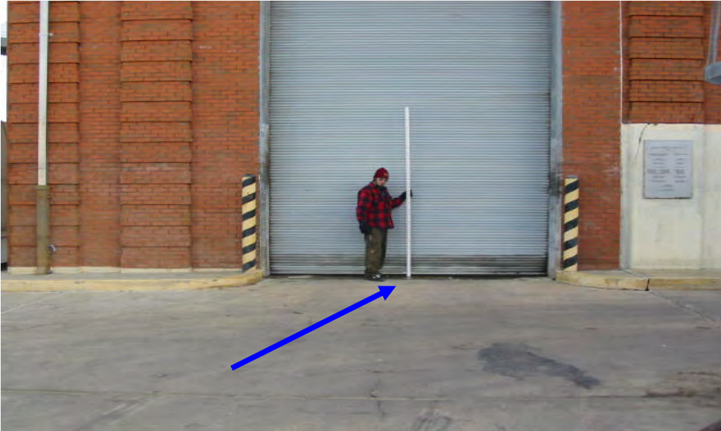
OP 19 Finished Floor #1 = -3.79 feet NAVD88(2004.65) Field Book 060851
