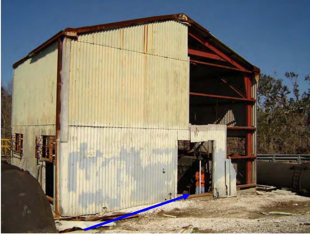
Finished Floor #2 = -8.21 feet NAVD88(2004.65) Field Book 060854
