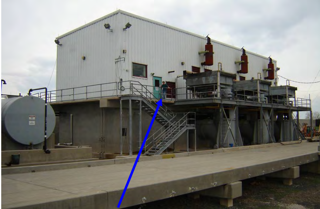
Finished Floor #1 = 15.52 feet NAVD88(2004.65) Field Book 060851
