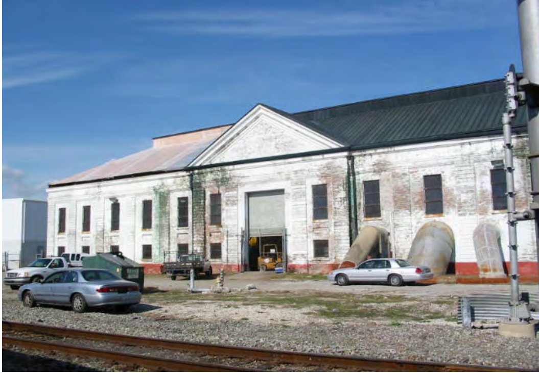
OP 17 Pump Station
