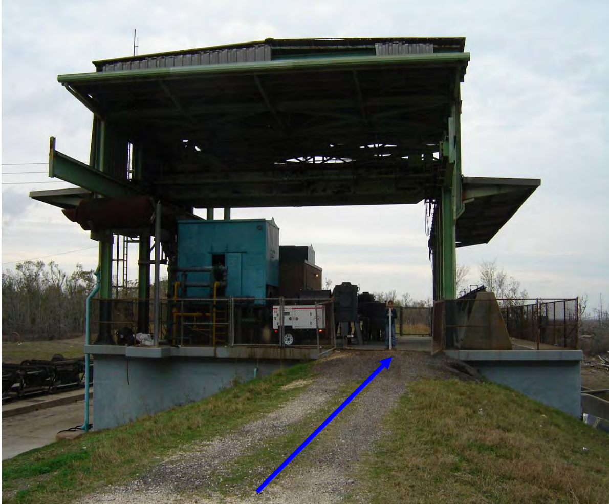
Finished Floor #1 = 13.92 feet NAVD88(2004.65) Field Book 060851
