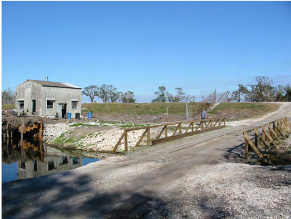
Belair Pump Station
