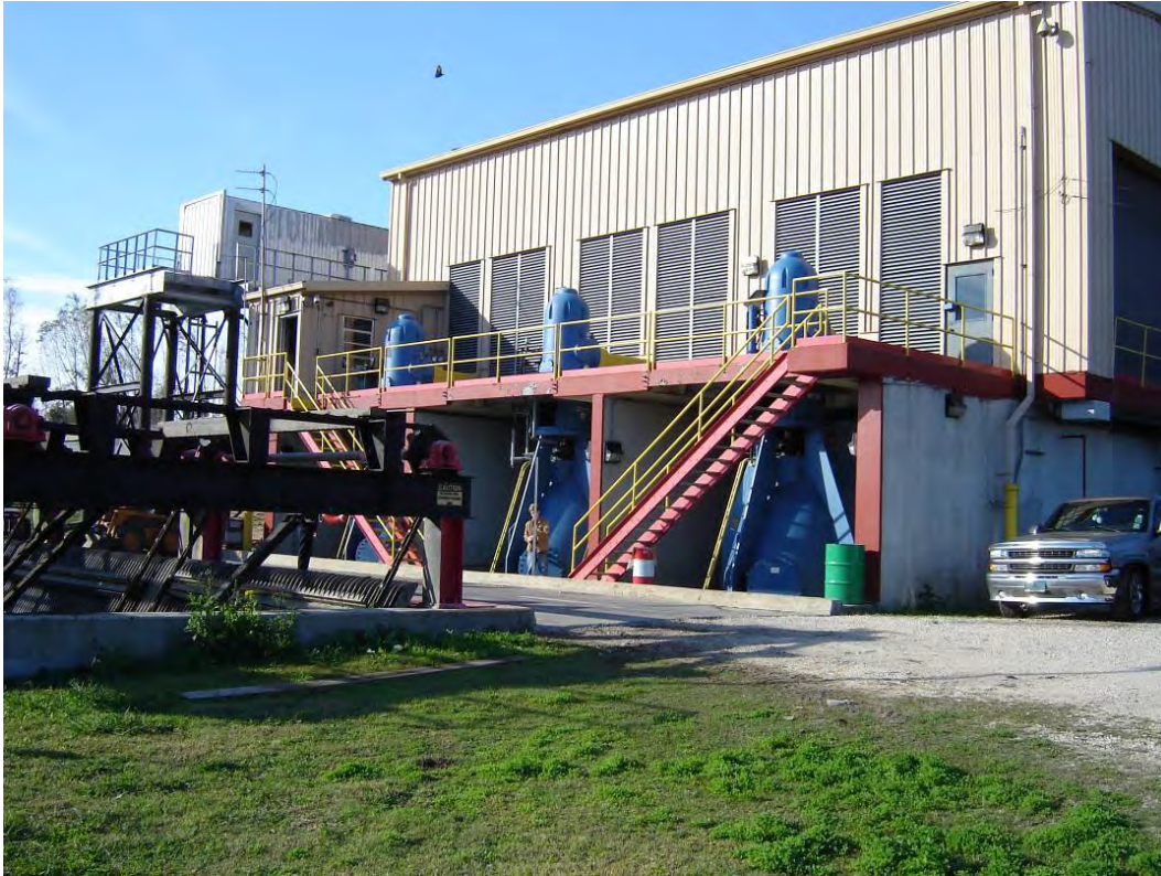
Westwego #2 Pump Station
