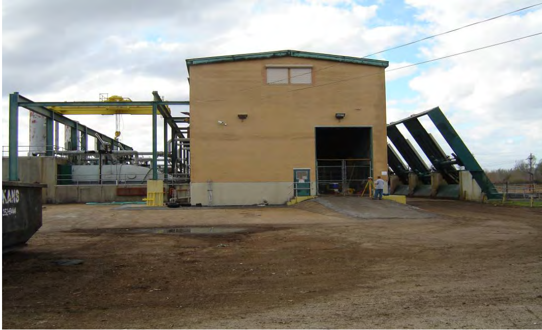
OP #13 PUMP STATION
