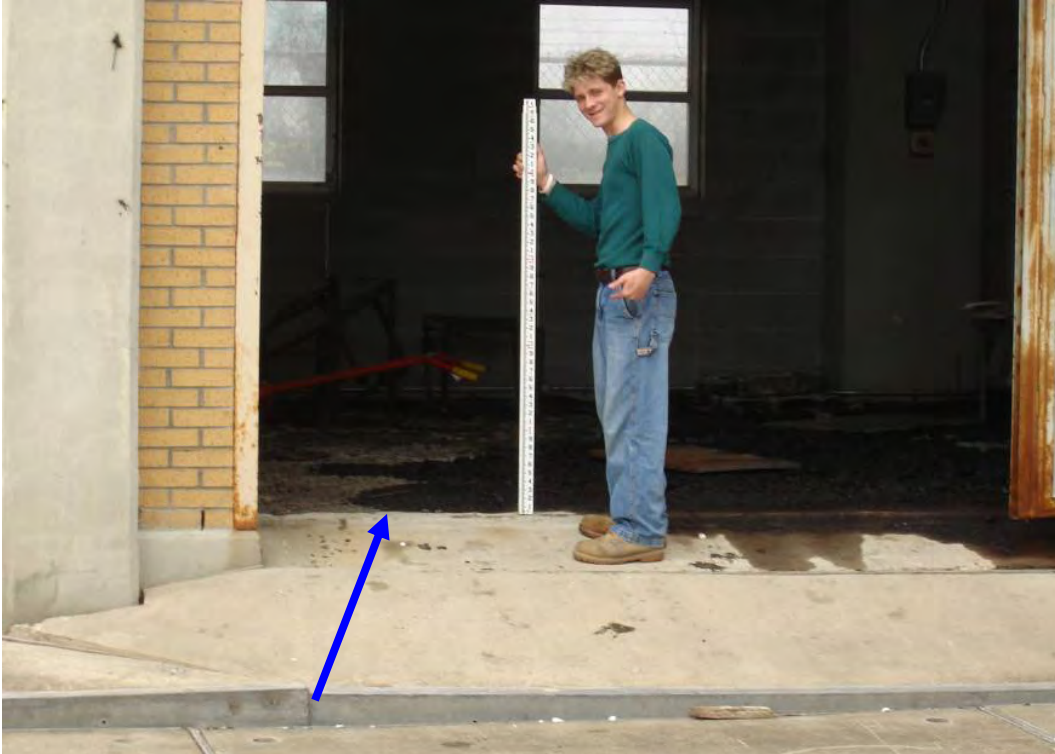
Finished Floor = 3.69 feet NAVD88(2004.65) Field Book 060851
