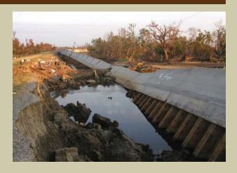
The terrestrial measure was incorrectly assumed to be equivalent to the water level datum. Using the terrestrial-based measure instead of the water level reference datum for design and construction caused some structures to be built too low.
