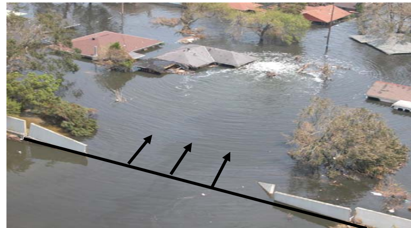
Displacement of wall levee
