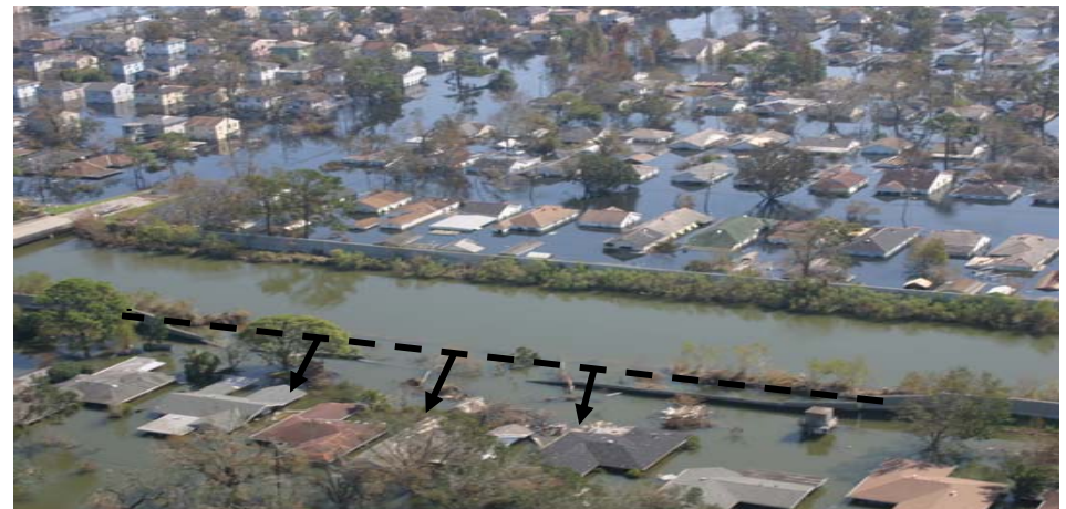
Displacement of wall levee
