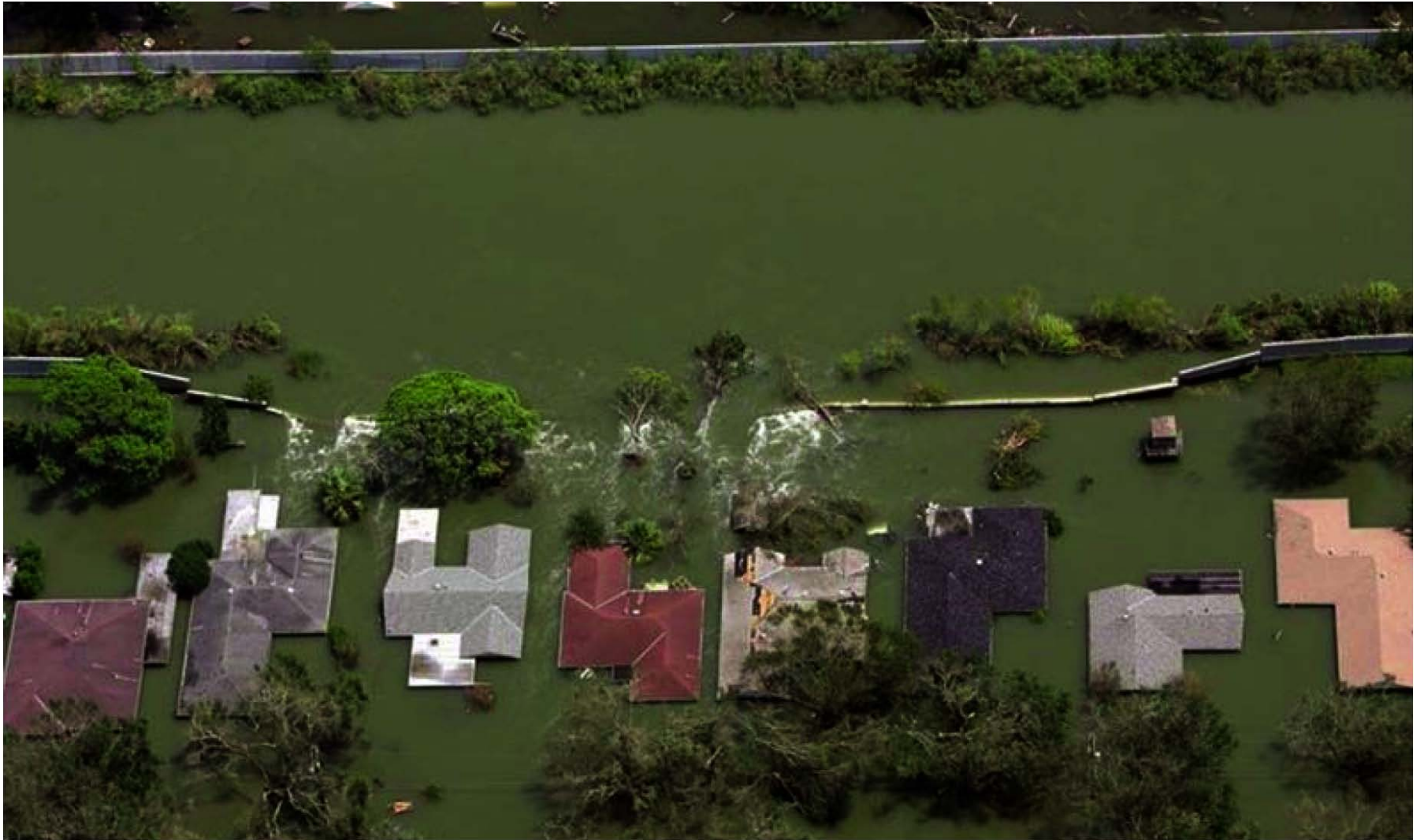
London Avenue north breach – about 410 ft wide – similar to 17 th Street canal I-wall failure
