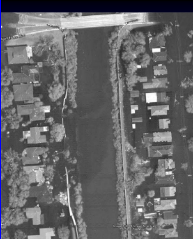
Robert E. Lee Boulevard Breach: 300 ft. Wide
