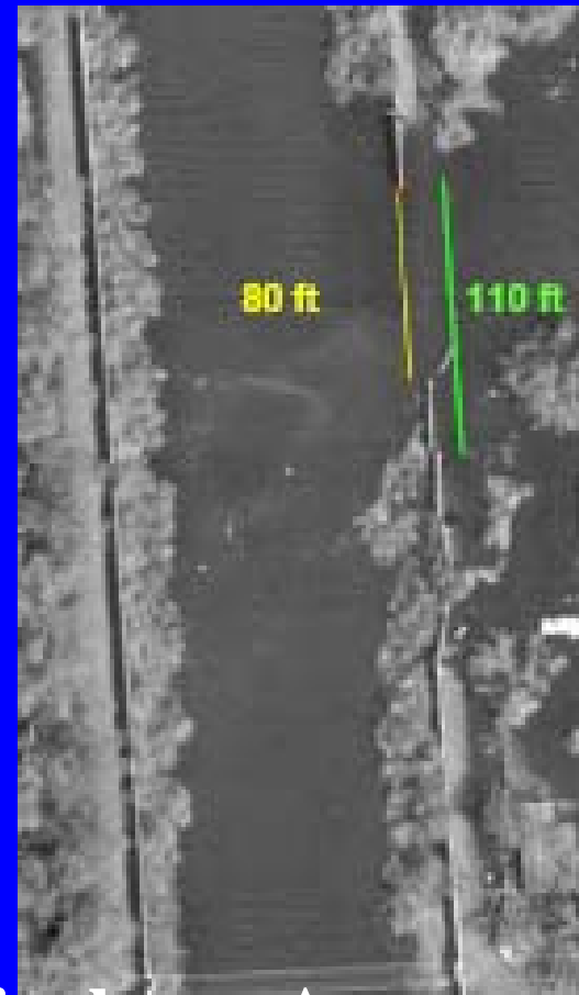
Mirabeau Avenue Breach: 80 ft. Wide
