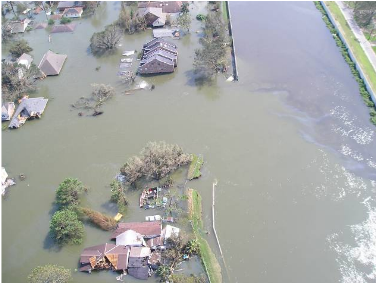
17th Street Canal Breach
