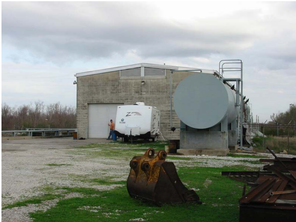
SCARSDALE PUMP STATION
