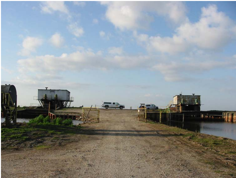
POINT CELESTE 1 AND 2 Pump stations
