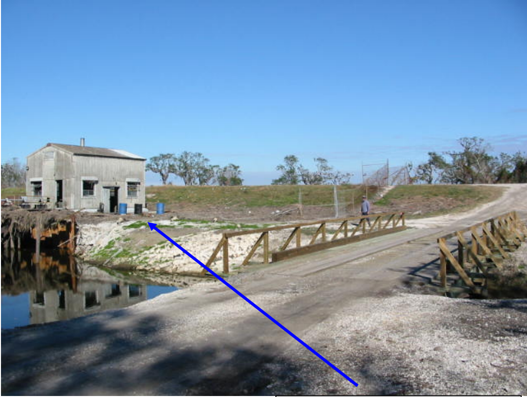
Belair Pump Station
