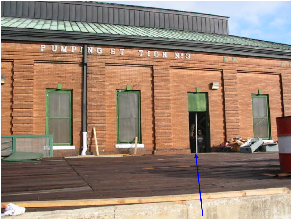
Finished Floor 1.230 feet NAVD88 2004.65 Field Book 060851
