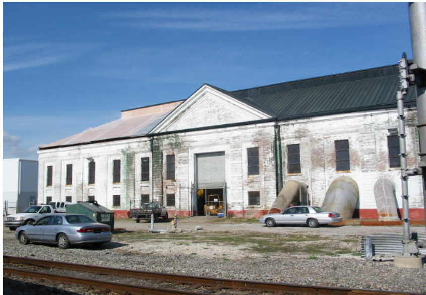
OP 17 Pump Station
