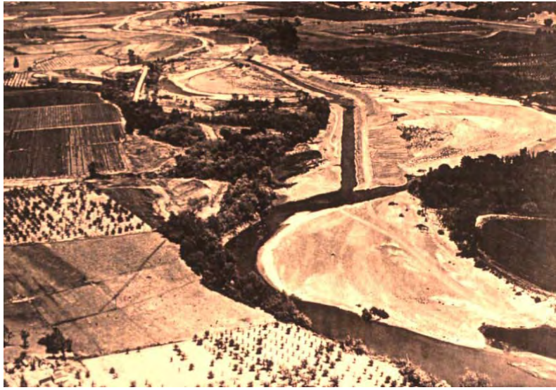
As reviewed by Mitch Swanson, formerly meandering river was channelized in late 1950s, cut-off bends mined
